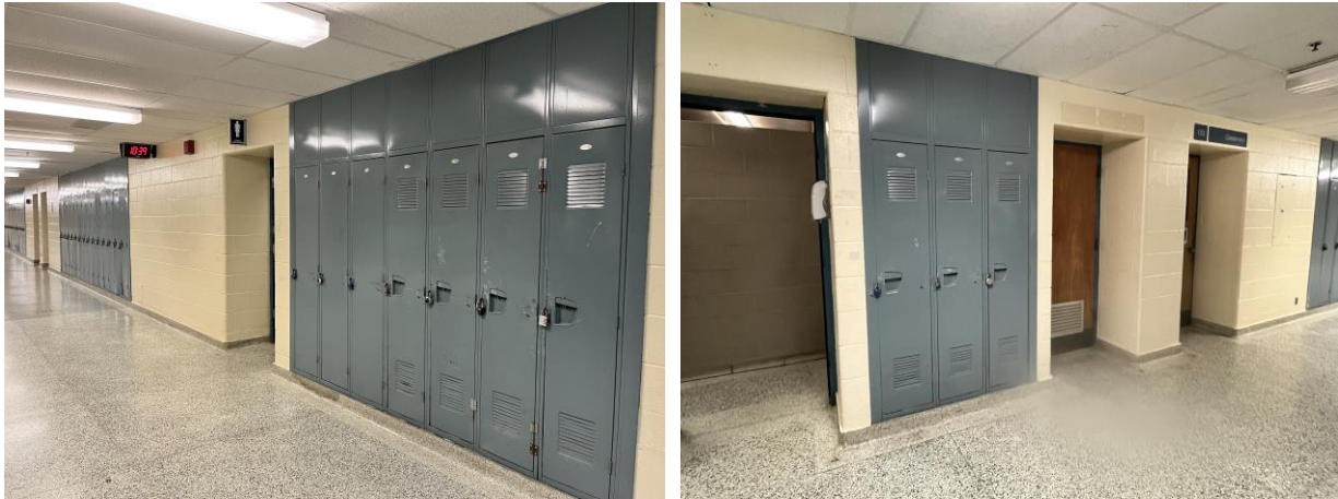
Corridor 1001 outside Washrooms
