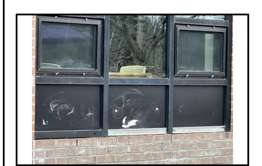
EXTERIOR VIEW - WINDOW AT KINDERGARTEN ROOM 139
