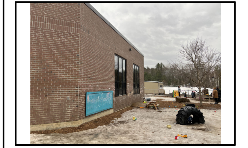
EXTERIOR VIEW - WINDOW AT KINDERGARTEN ROOM 139
