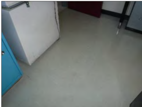
Asbestos-containing 9" light grey vinyl floor tiles with white streaks (VT1)
