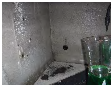
Transite panels present in the fumehood in Room 201, in good condition.
