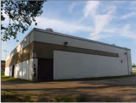
Asbestos-containing stucco present on the exterior walls of the 1959, 1962 and 1966 additions.
