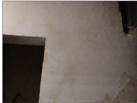
Repaired, asbestos-containing plaster on the walls of Room 158A.
