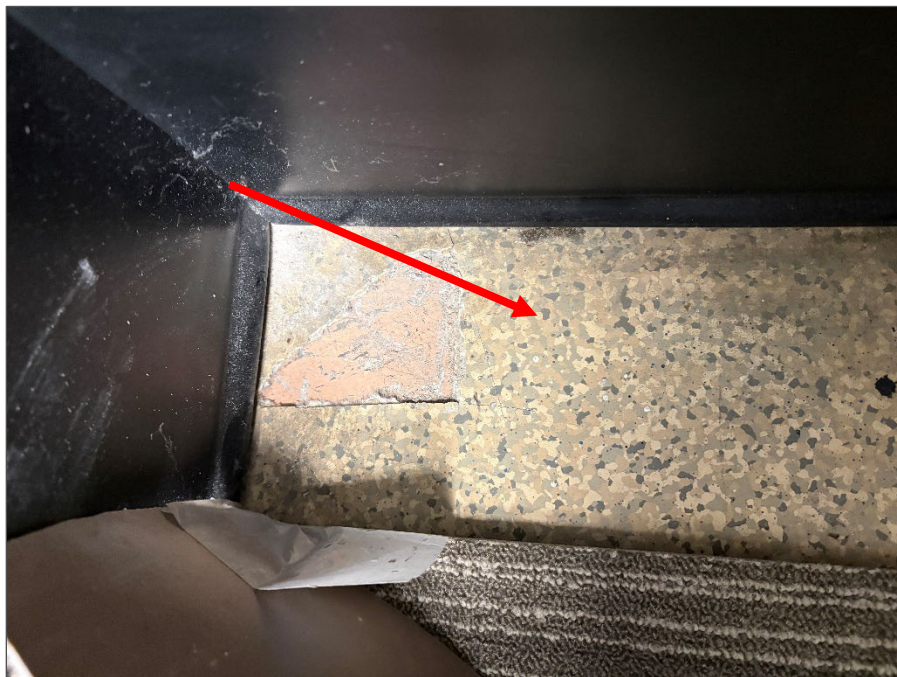
Photo 4: Non-asbestos vinyl sheet flooring, concealed beneath the carpet.
