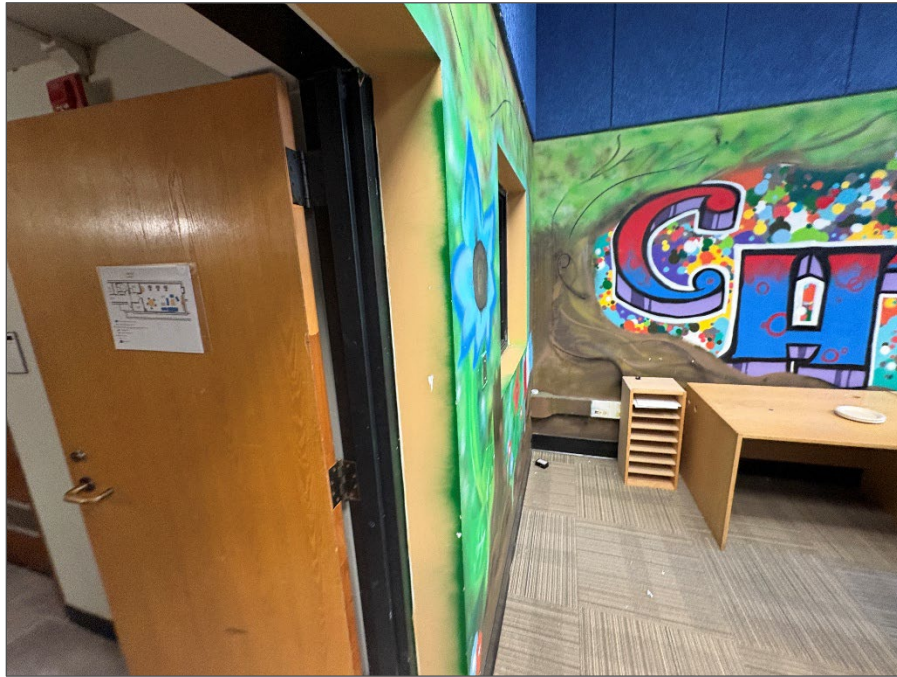
Photo 3: Non-lead based beige paint on drywall.
