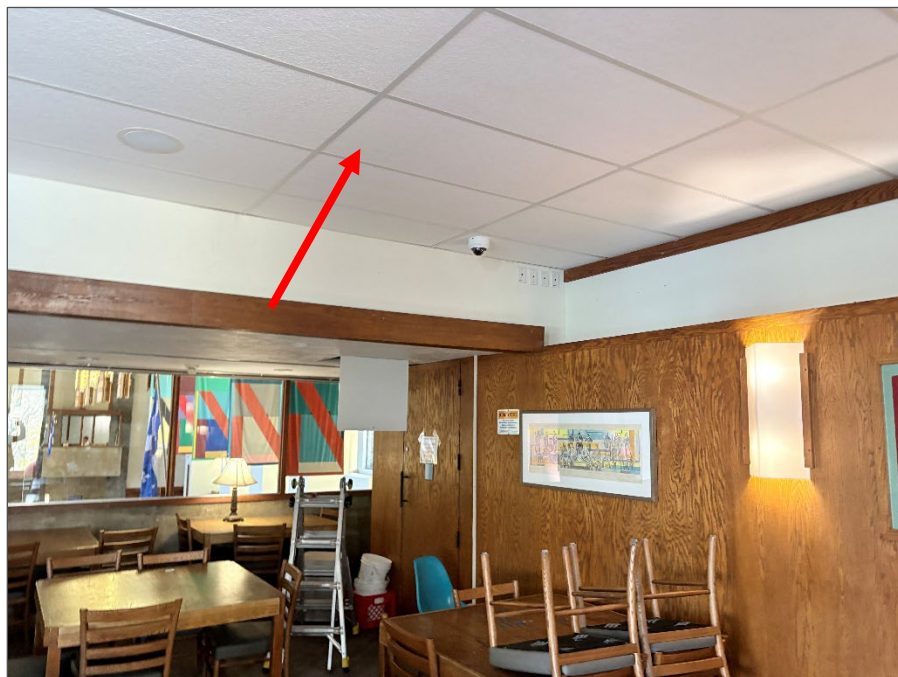
Photo 2: Non-asbestos (2' x 4') acoustic ceiling tiles.
