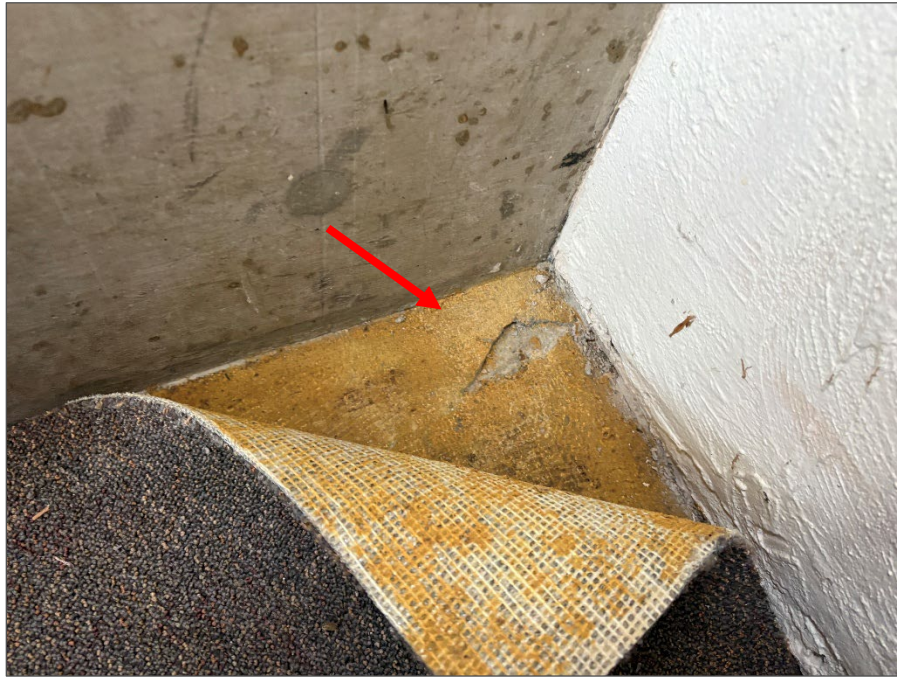
Photo 3: Non-asbestos carpet mastic.
