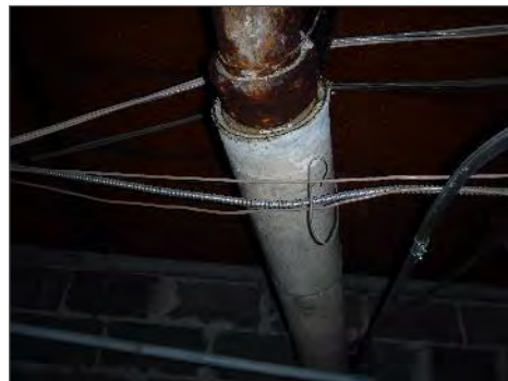
Asbestos-containing sweatwrap pipe insulation, in good condition.
