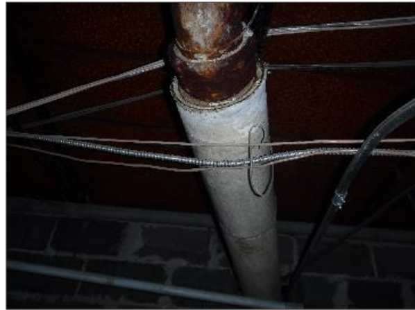
Asbestos-containing sweatwrap pipe insulation, in good condition.
