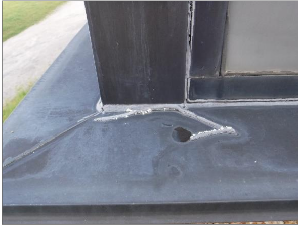
Asbestos-containing grey, soft exterior window caulking on the 1986 addition.
