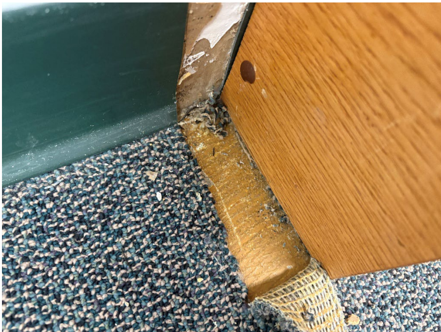
Photo 3: Non-asbestos vinyl baseboard and associated mastic.
