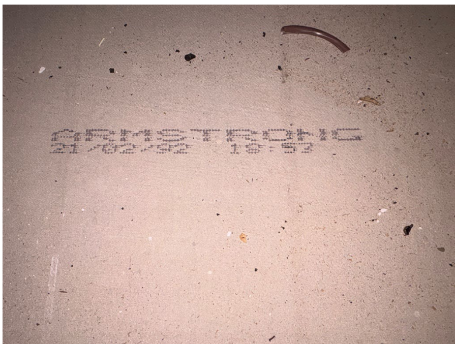
Photo 4: Non-asbestos acoustic ceiling tile (date stamped 1992).
