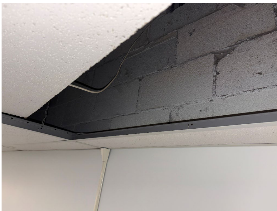
Photo 2: Non-asbestos mortar on concrete block on walls.
