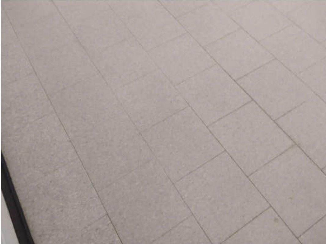
V0000 (None), 12 x 12 grey mottled, Floor, Vinyl Floor Tile and Mastic, Classroom 132 (Location #: 35) Post 2005 new
