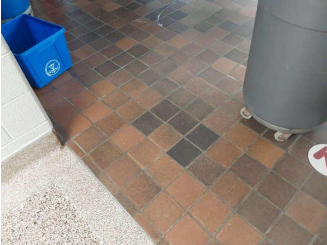
V9500 (Presumed Asbestos), Floor, Mortar, Corridor (Location #: 46)
