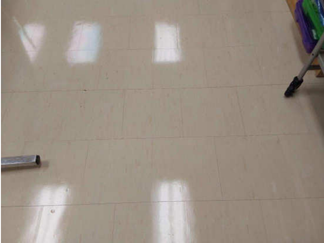
S0010 (Confirmed Asbestos), 12 x 12 tan with white and brown flecks, Floor, Vinyl Floor Tile and Mastic, Classroom 103 (Location #: 26) Mastic is presumed to contain asbestos
