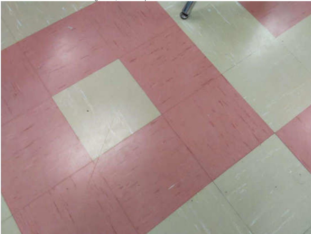
S0021 (Confirmed Asbestos), 9 x 9 red with dark red streaks, Floor, Vinyl Floor Tile and Mastic, Room 3 (Location #: 5) Mastic is presumed to contain asbestos
