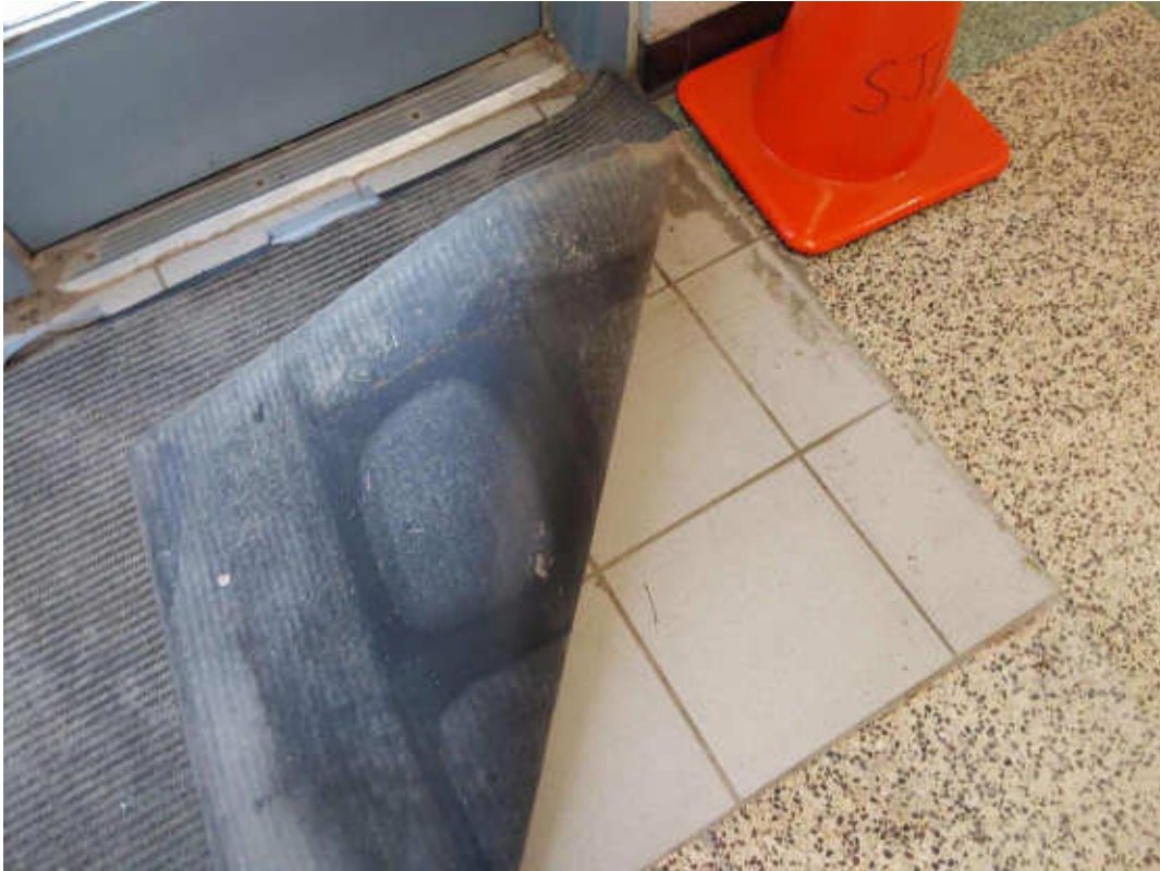
V9500 (Presumed Asbestos), Floor, Mortar, Corridor (Location #: 25)
