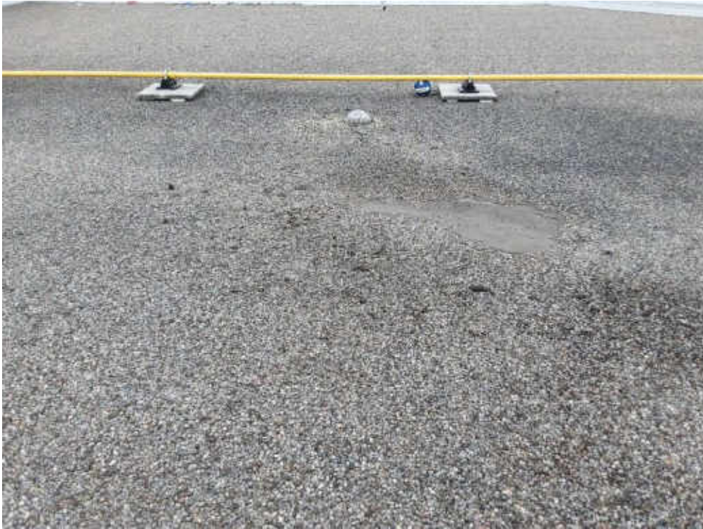
S0009C (Confirmed Asbestos), Built up roofing, Other, Roofing material, Roof 1 (Location #: 54)
