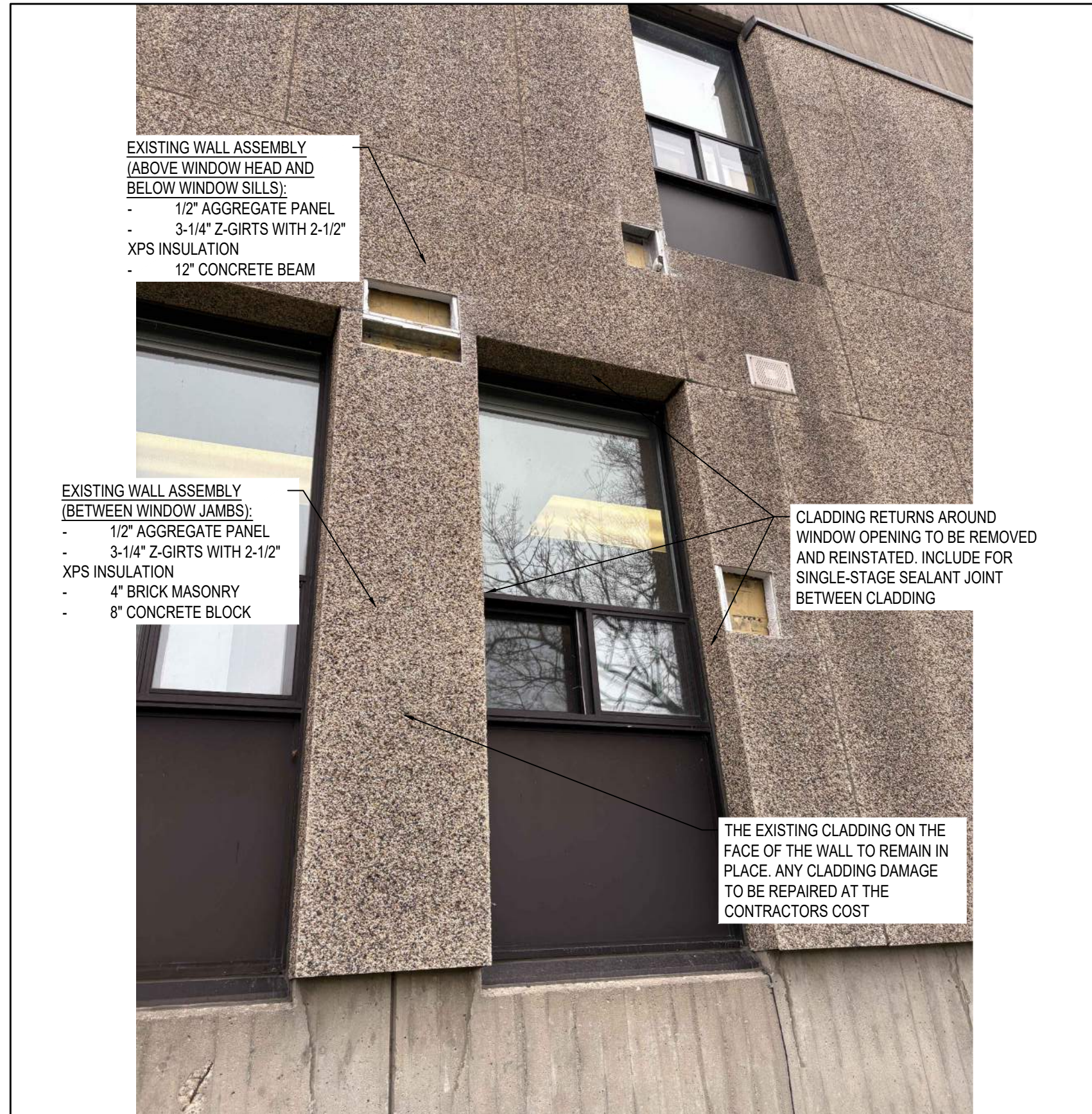
5 EXTERIOR VIEW OF W4 R600
