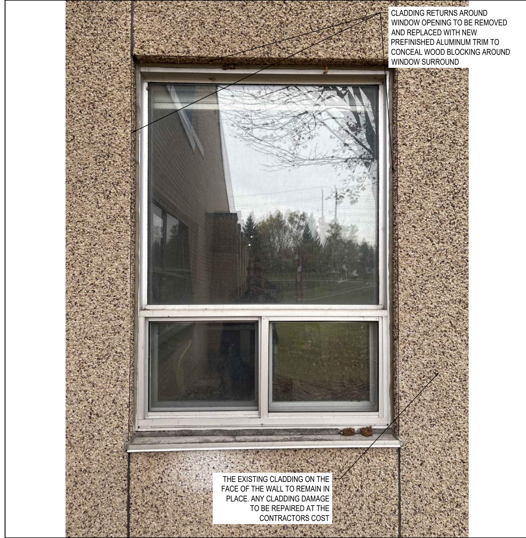
2 EXTERIOR VIEW OF W1 R600
