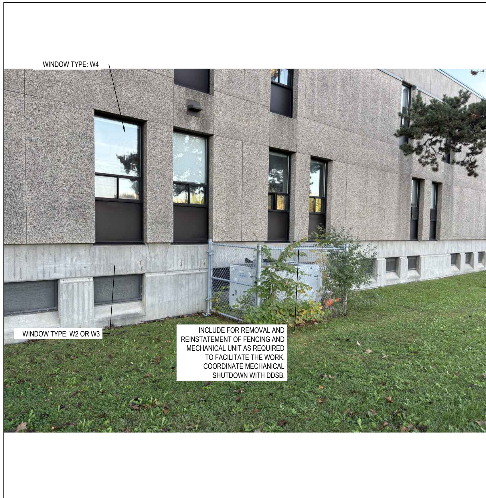
1 EXTERIOR VIEW OF W2 AND W3 R601
