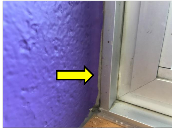
Non-asbestos firm grey caulking on interior window frame.
