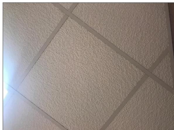
Non-asbestos 2'x2' textured acoustic ceiling tiles with pinholes.
