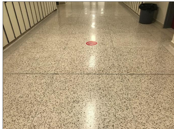
Non-asbestos terrazzo floor.
