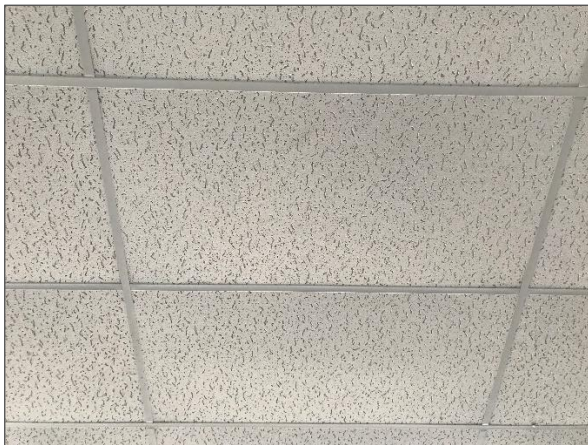
Non-asbestos 2'x4' acoustic ceiling tiles with thick widthwise fissures and pinholes.
