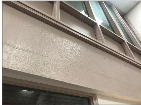
Non-asbestos textured plaster on wall.
