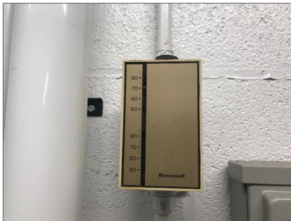
Liquid mercury is present in thermostat ampules.
