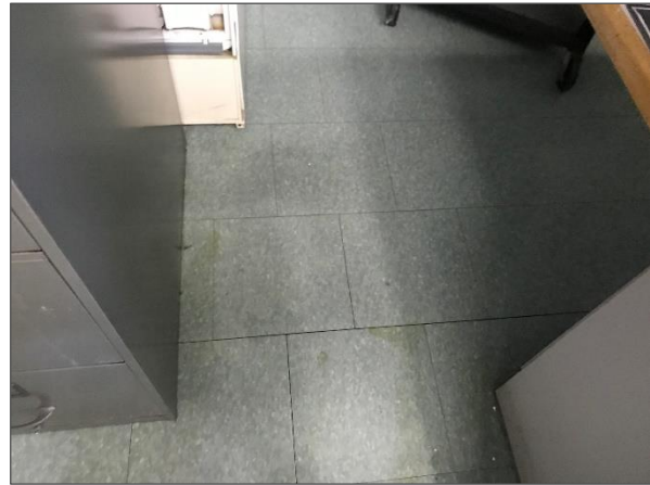
Non-asbestos 12"x12" turquoise vinyl floor tiles with white flecks.
