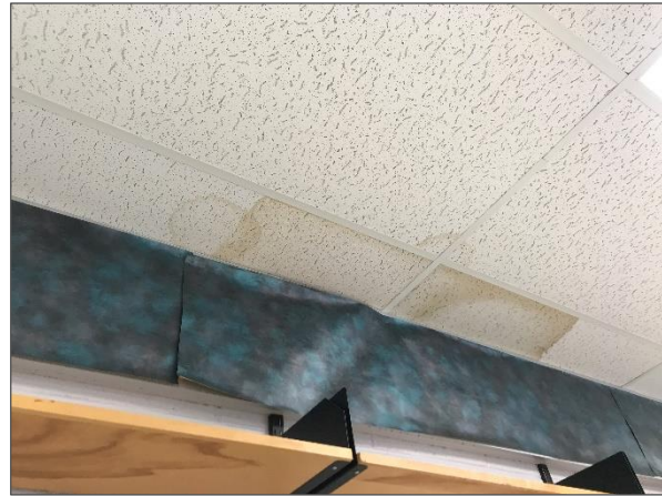
Water stained lay-in acoustic ceiling tiles in Classroom 225.
