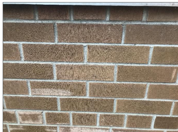
Non-asbestos mortar present between joints of exterior brick cladding.
