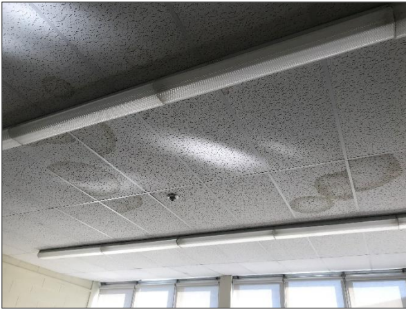
Water stained lay-in acoustic ceiling tiles in Classroom 112.
