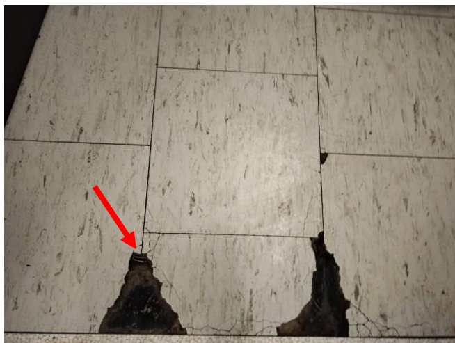
Photo 1: View of the asbestos-containing 12"x12" beige vinyl floor tiles with grey streaks (see arrow) observed to be in fair condition within Custodian Room 206.
