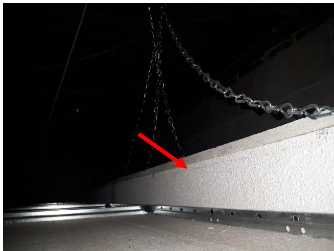
Photo 5: View of the asbestos containing insulation ceiling panels (see arrow) observed to be in good condition around the light fixtures and above the drop ceiling within Room 210.
