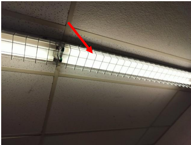
Photo 9: View of the mercury containing fluorescent light tubes (see arrow) observed to be in good condition throughout the Subject Building.
