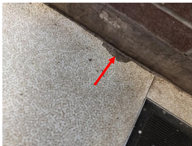
Photo 4: View of the asbestos containing beige vinyl sheet flooring (see arrow) observed in fair condition within the Corridor 110 near the Main Entrance.
