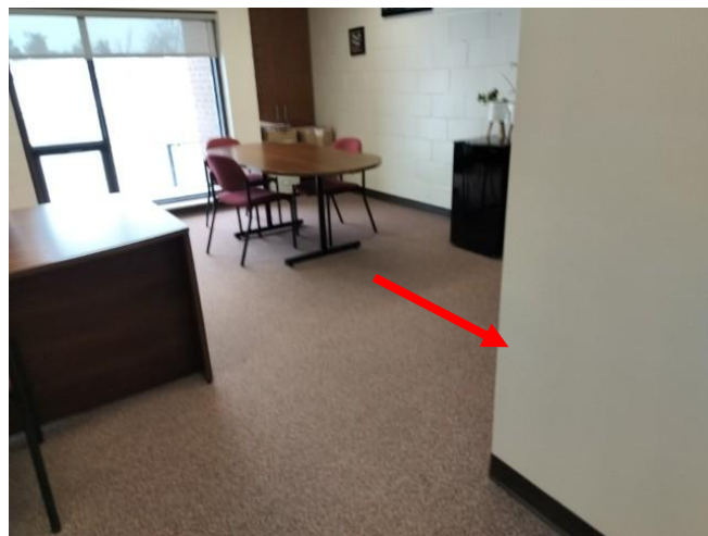
Photo 2: View of the drywall finishes with associated asbestos containing drywall joint compound (see arrow) observed to be in good condition within the Principal Room.
