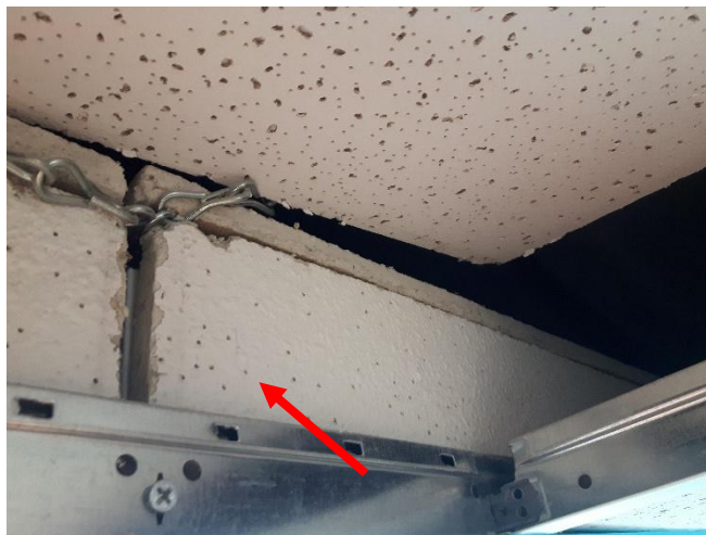
Photo 6: Additional view of the asbestos containing insulation ceiling panels (see arrow) observed to be in good condition around the light fixtures and above the drop ceiling within Room 210.
