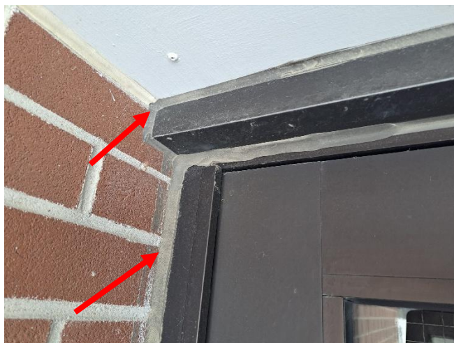
Photo 8: View of the non-asbestos containing exterior grey caulking (see right arrow) and brick mortar (see left arrow) observed to be in good condition throughout the Subject Building.
