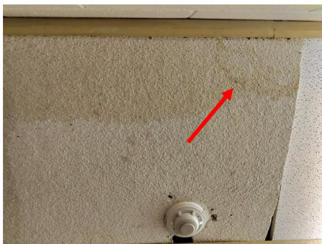
Photo 3: View of the asbestos containing 2' x 4' white textured ceiling tiles (see arrow) observed to be in fair condition in the Custodian Storage Room 115.
