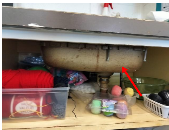
Photo 10: View of asbestos containing gold sink coating (see arrow) observed to be in good condition within Room 203
