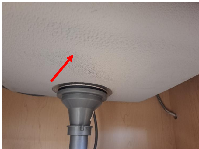
Photo 1: View of the non-asbestos containing white sink coating (see arrow) observed within Classroom 227.
