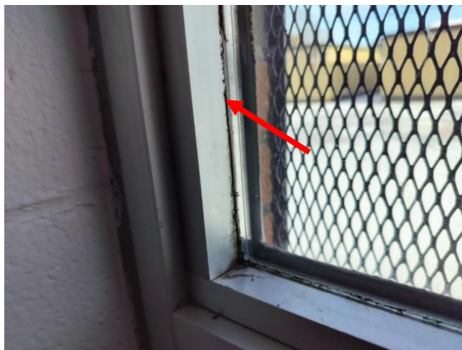
Photo 2: View of the asbestos containing grey glaze (see arrow) observed to be in good condition on the interior windows dated from 1984.
