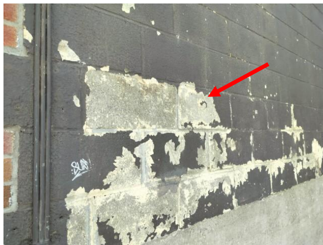
Photo 8: View of the lead containing brown paint (see arrow) observed in poor condition on the exterior concrete walls of the Subject Building.
