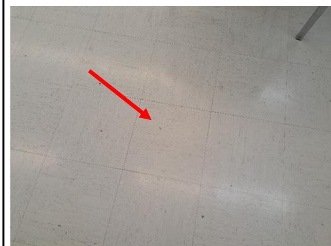
Photo 9: View of the asbestos-containing 12”x12” off-white with dark streaks vinyl floor tiles observed to be in good condition within Room 203.
