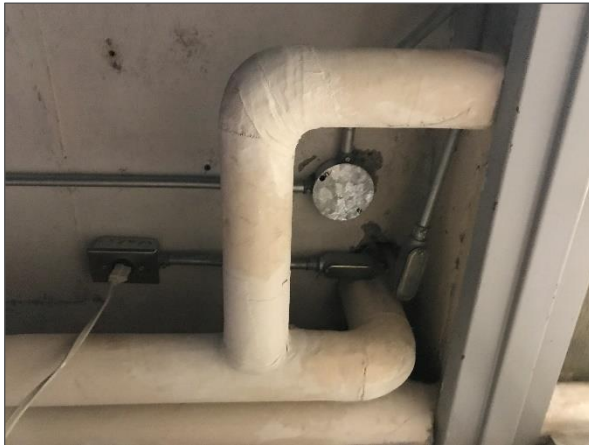
Asbestos-containing paring cement insulation on pipe elbows.
