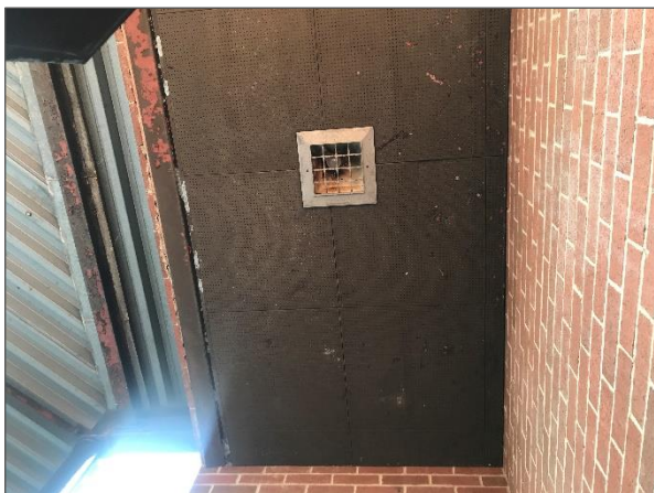
Presumed asbestos-containing Transite board present on underside of exterior canopy.
