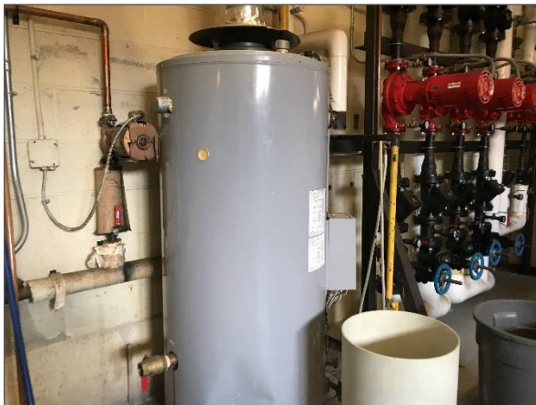
Non-asbestos fibreglass insulated hot water tank with metal jacketing.
