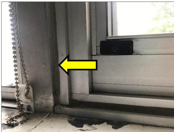
Asbestos-containing soft grey caulking on interior window frame.
