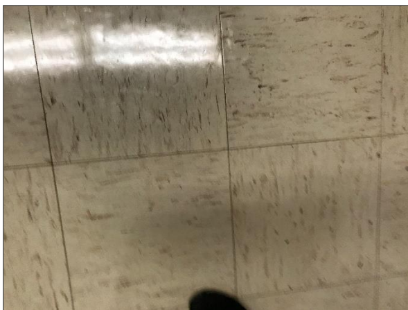
Asbestos-containing 12"x12" beige vinyl floor tiles with brown streaks.
