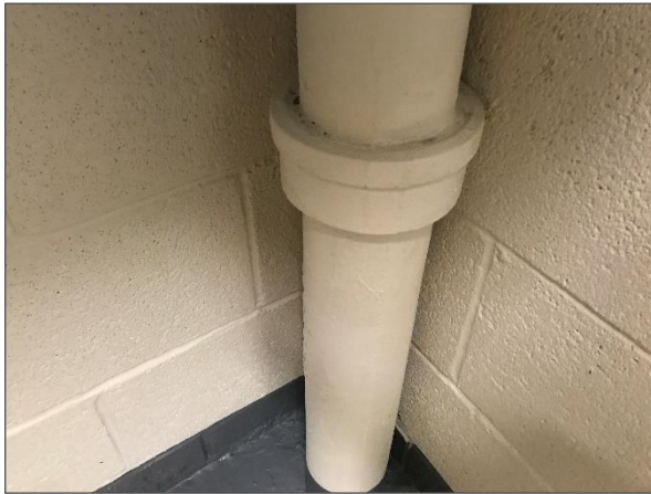
Lead caulking is present in fittings of bell and spigot fittings of cast iron pipes.
