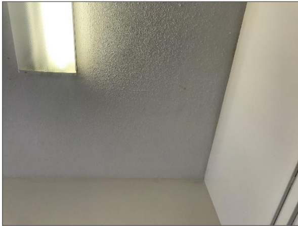
Asbestos-containing texture finish on plaster ceiling.
