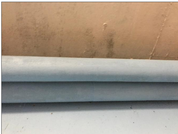
Asbestos-containing Aircell insulation on straight sections of pipes.
