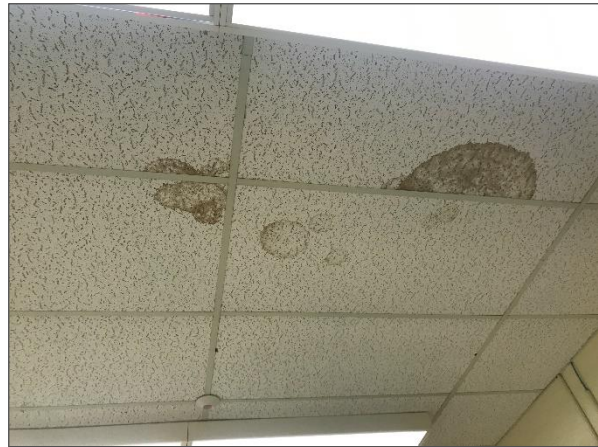
Water stained lay-in acoustic ceiling tiles in Classroom 212.
