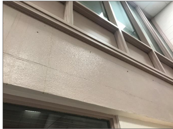
Non-asbestos textured plaster on wall.
