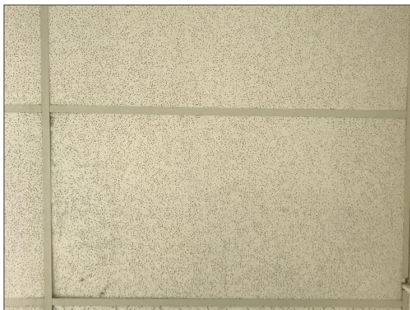
Non-asbestos 2'x4' acoustic ceiling tiles with dense small and medium pinholes.
