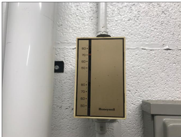
Liquid mercury is present in thermostat ampules.
