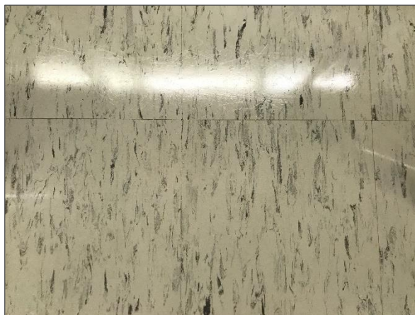
Non-asbestos 12"x12" off-white vinyl floor tiles with black and grey streaks.
