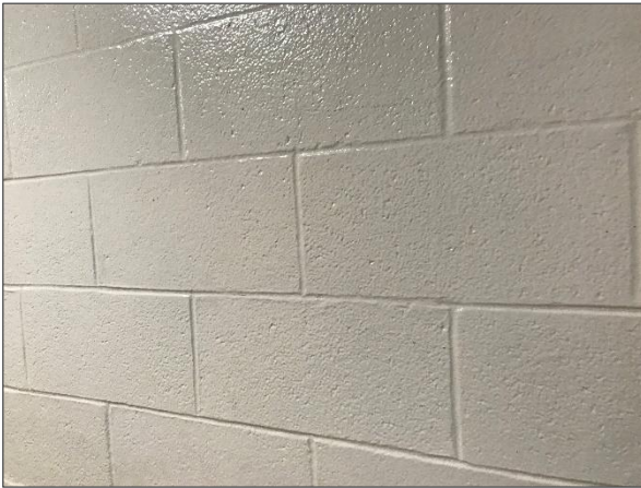
Asbestos-containing paint present on concrete block wall.
