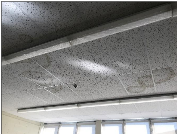
Water stained lay-in acoustic ceiling tiles in Classroom 112.
