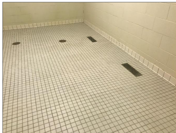
Presumed asbestos-containing thinset present behind ceramic tiles on floor.
