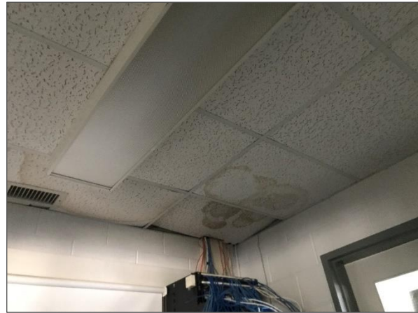
Water stained lay-in acoustic ceiling tiles in Storage 227.
