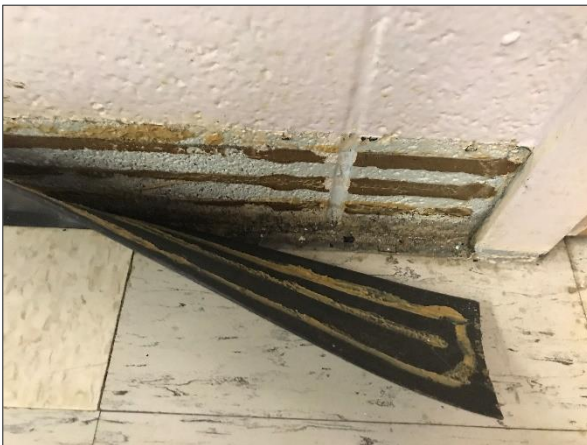
Non-asbestos adhesive present behind rubber baseboard.
