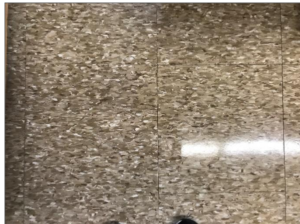
Non-asbestos 12"x12" beige vinyl floor tiles with white and beige blotches.
