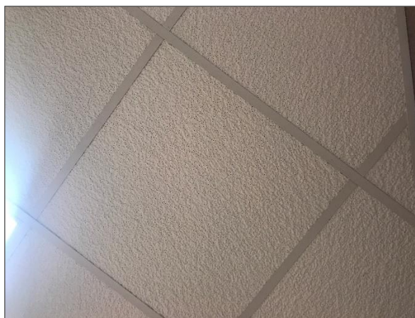
Non-asbestos 2'x2' textured acoustic ceiling tiles with pinholes.
