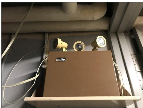
Lead-acid batteries are present in emergency lights.
