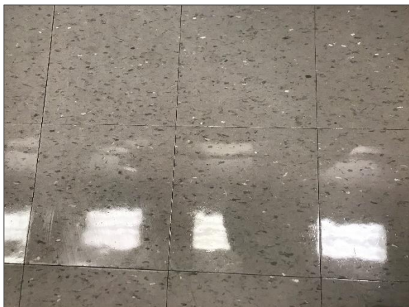
Non-asbestos 12"x12" grey vinyl floor tiles with white and grey flecks.
