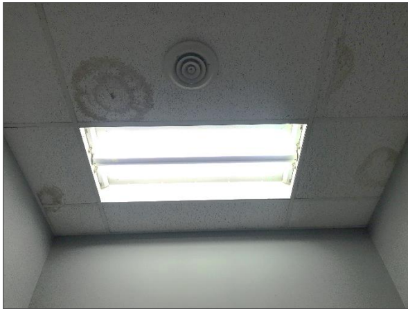
Water stained lay-in acoustic ceiling tiles in Office 129A.
