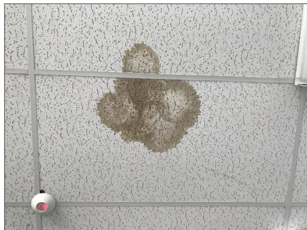
Water stained lay-in acoustic ceiling tiles in Classroom 217.
