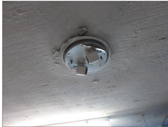
Asbestos-containing heat shield.
