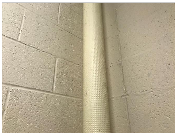
Presumed asbestos-containing Transite pipe.
