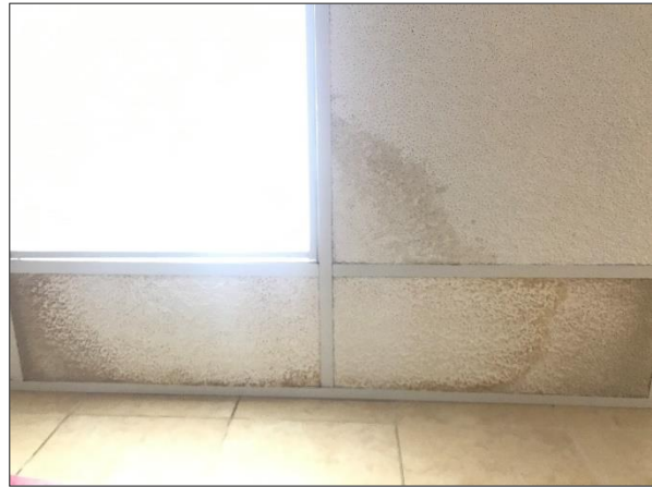
Water stained lay-in acoustic ceiling tiles in Washroom 128.
