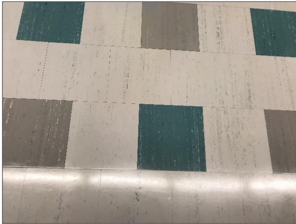
Asbestos-containing 9"x9" vinyl floor tiles of various colours.
