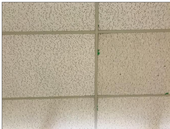
Non-asbestos 2'x4' acoustic ceiling tiles with dense short widthwise fissures.
