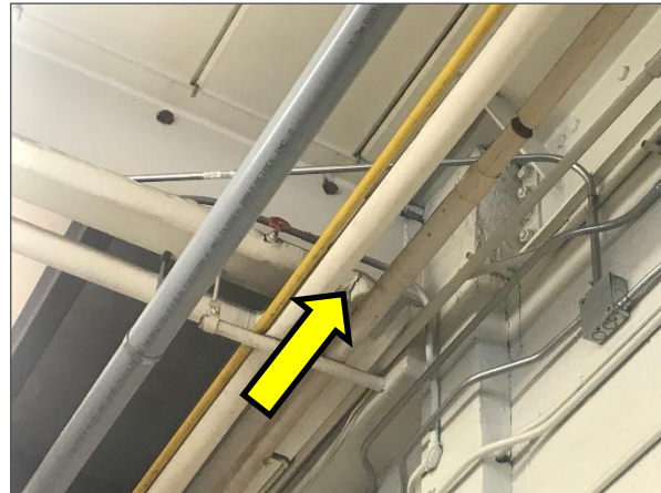
Damaged asbestos-containing paring cement insulation present on pipe elbow in Automotive Shop 153.
