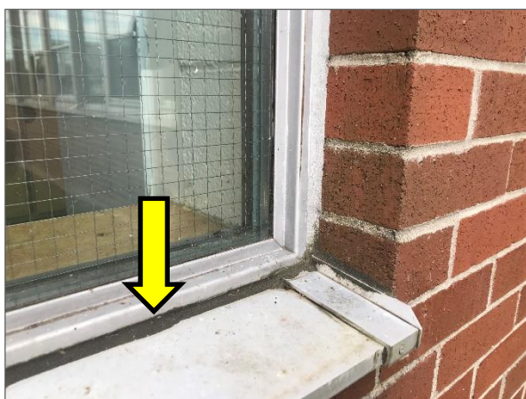
Asbestos-containing beige caulking on exterior window frame.
