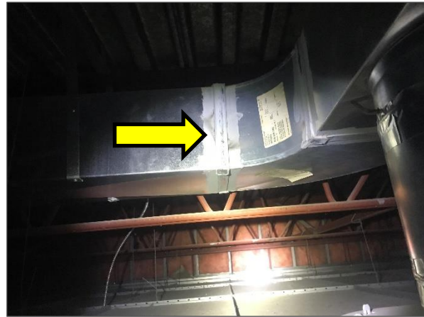
Non-asbestos light grey duct mastic.
