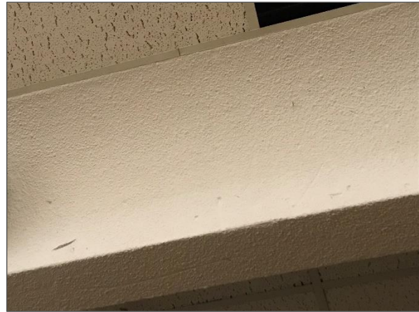
Asbestos-containing texture finish on bulkhead.
