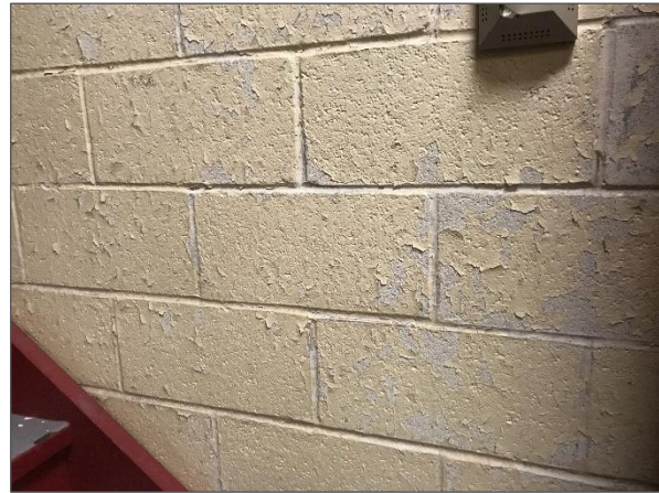
Damaged asbestos-containing paint on concrete block wall in Storage Room 139.
