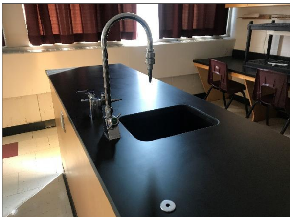
Presumed asbestos-containing Transite board present as countertops.
