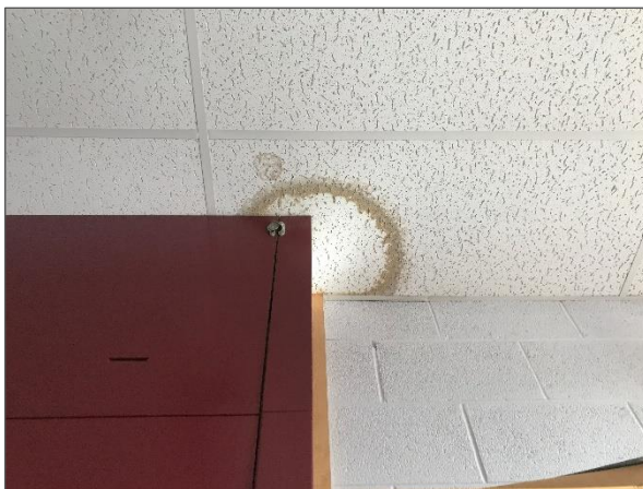
Water stained lay-in acoustic ceiling tiles in Classroom 217.
