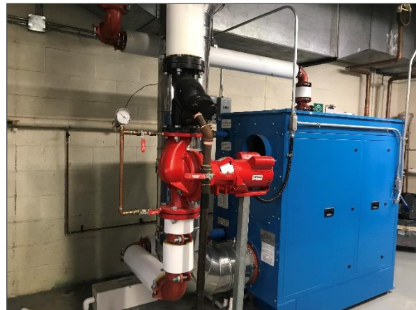
Non-asbestos fibreglass insulated boiler with metal jacketing.
