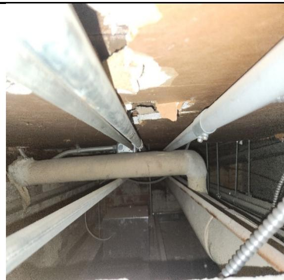
**Photograph 2:** View of the asbestos-containing paper material identified above the metal deck of the elevator shaft at the Subject Location.
