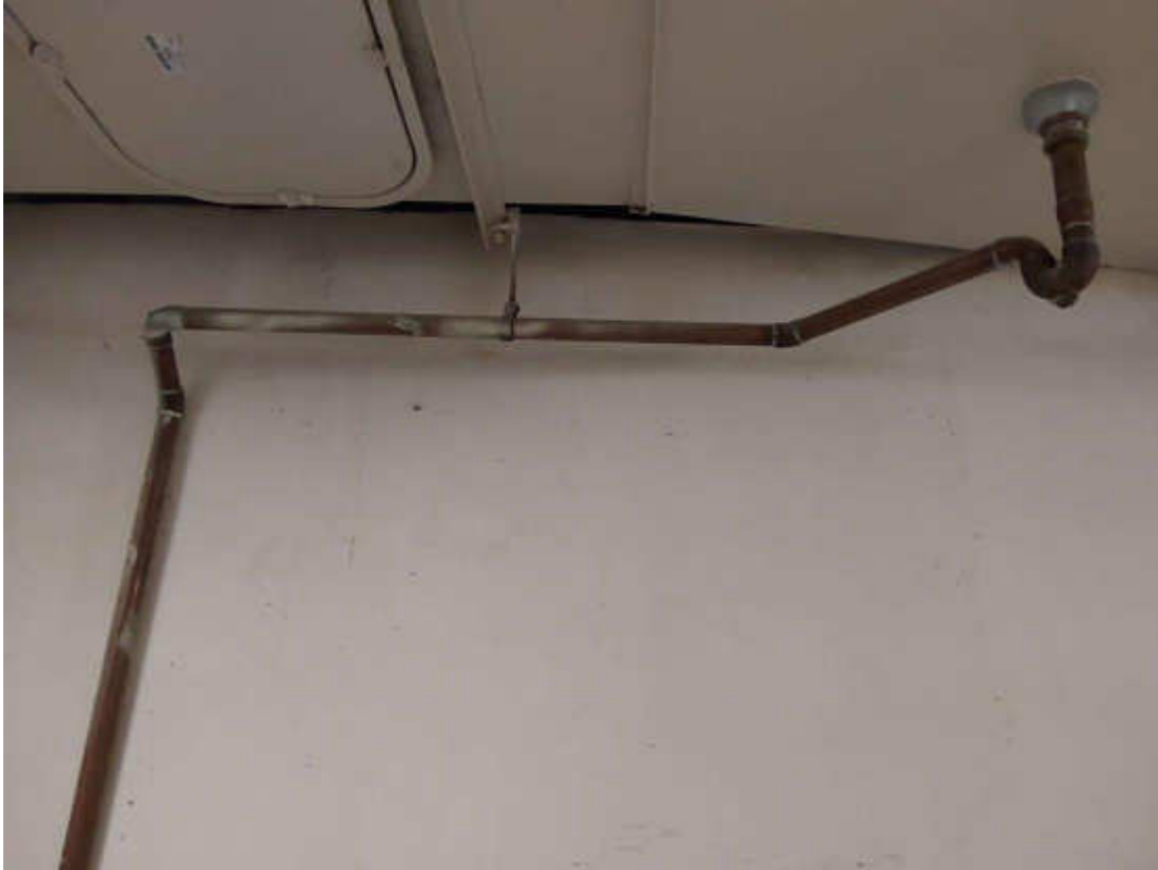
Piping, Not Insulated, Mechanical Room (Location #: 2)
