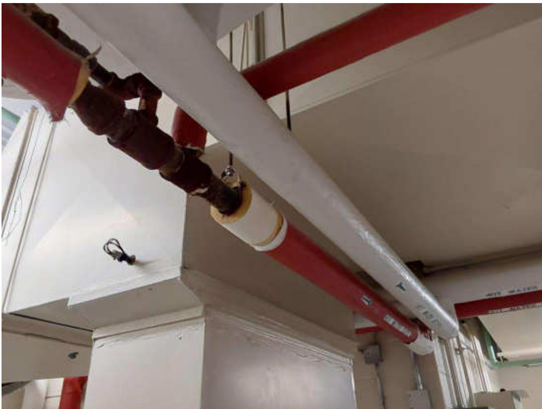
Fiberglass insulated, Piping, Fibreglass, Mechanical Room (Location #: 2)
