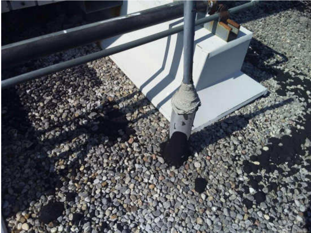
S0003C (None), Grey caulking over black Air Handling Unit conduit isolation, Roof Sections 1A and 1B (Location #: 1)
