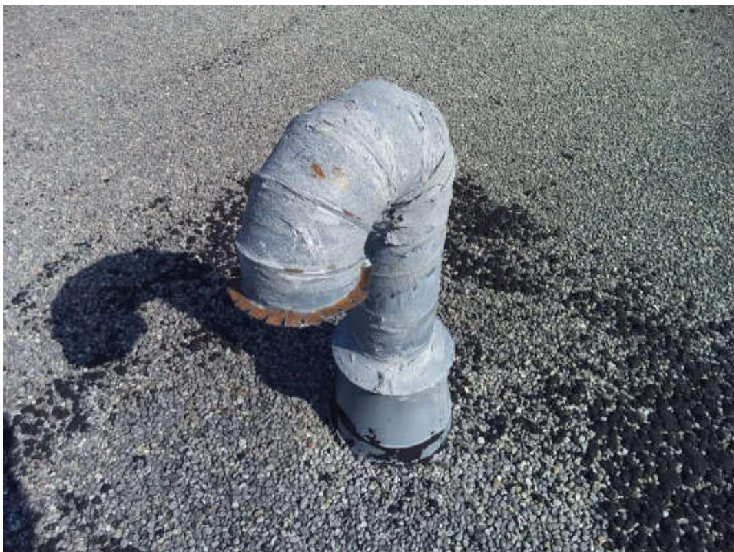
S0004A (None), Grey mastic with gold flake exhaust, Duct, Mastic, Grey, Roof Sections 1A and 1B (Location #: 1)
