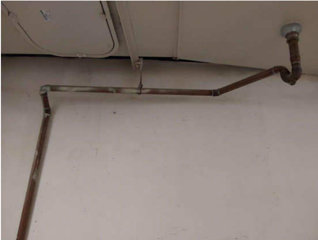
Piping, Not Insulated, Mechanical Room (Location #: 2)
