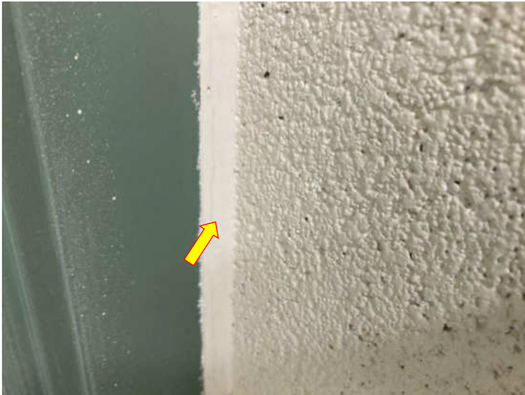
S0007C (None), Grey caulking on door frames, Other, Caulking, Mechanical Room (Location #: 2)
