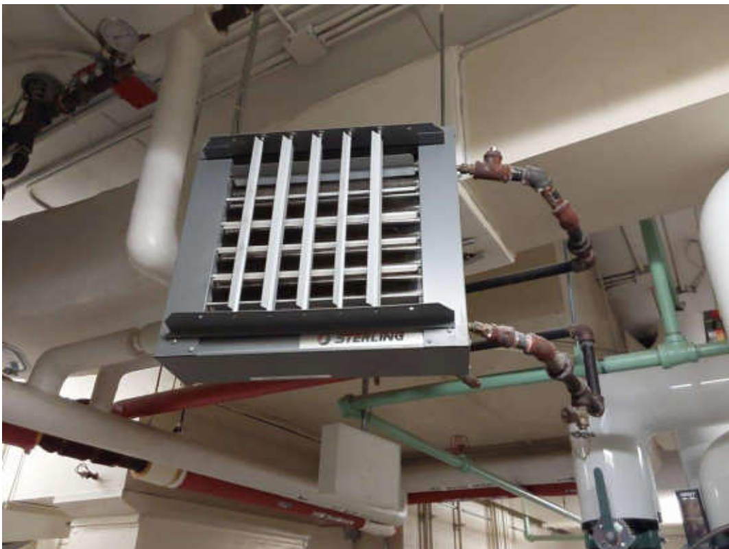
V0000 (None), Mechanical Equipment, Unit Heater, Not Insulated, Mechanical Room (Location #: 2)
