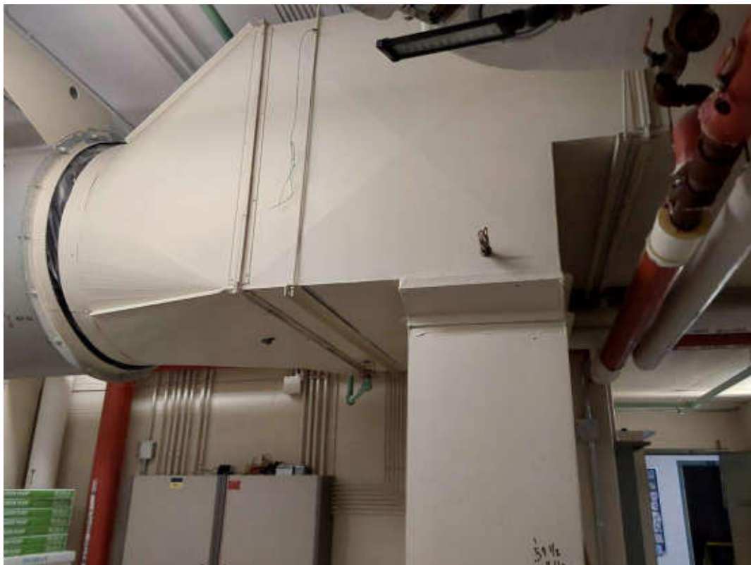
Duct, All, Not Insulated, Mechanical Room (Location #: 2)
