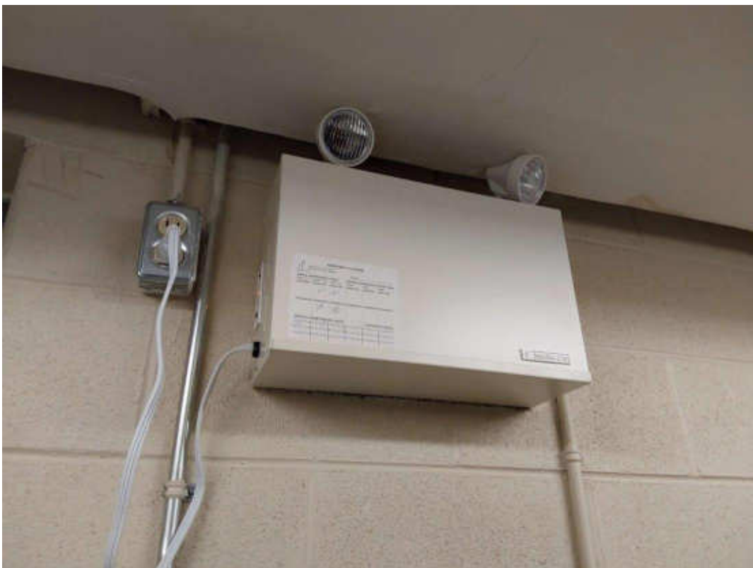
Pb Products, V9500(Presumed), BATTERIES IN EMER. LIGHTS, Mechanical Room (Location #: 2)
