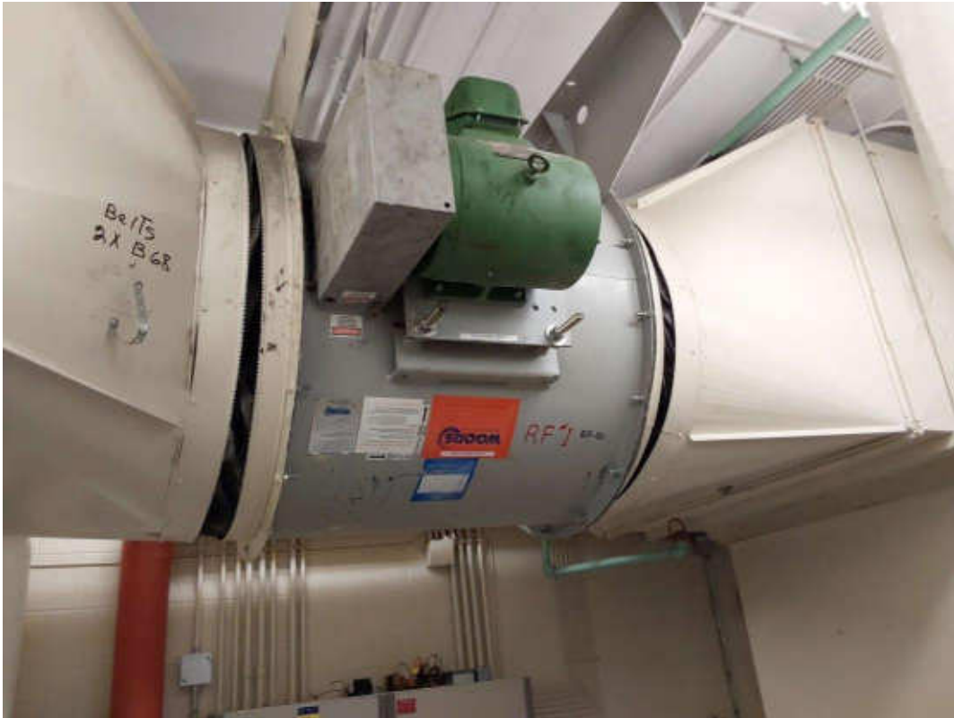
V0000 (None), Black rubber vibration damper, Duct, Duct Connector, Rubber, Mechanical Room (Location #: 2)
