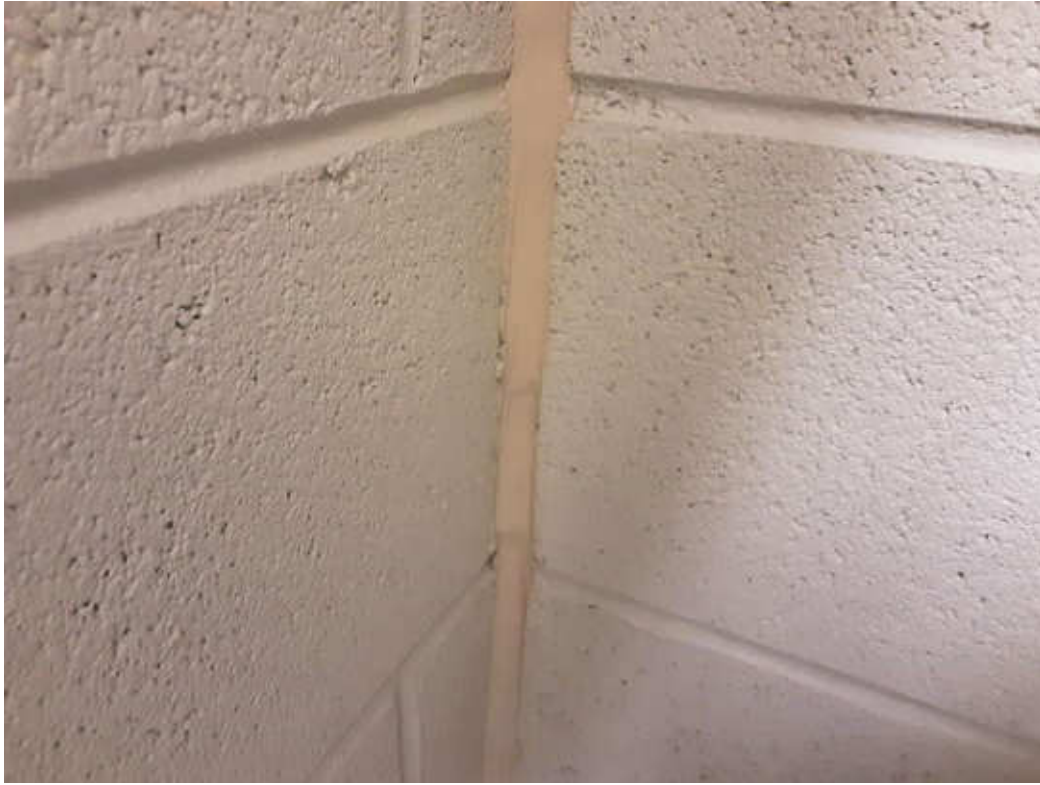
S0005C (None), White/beige caulking, Other, Caulking, Mechanical Room (Location #: 2)
