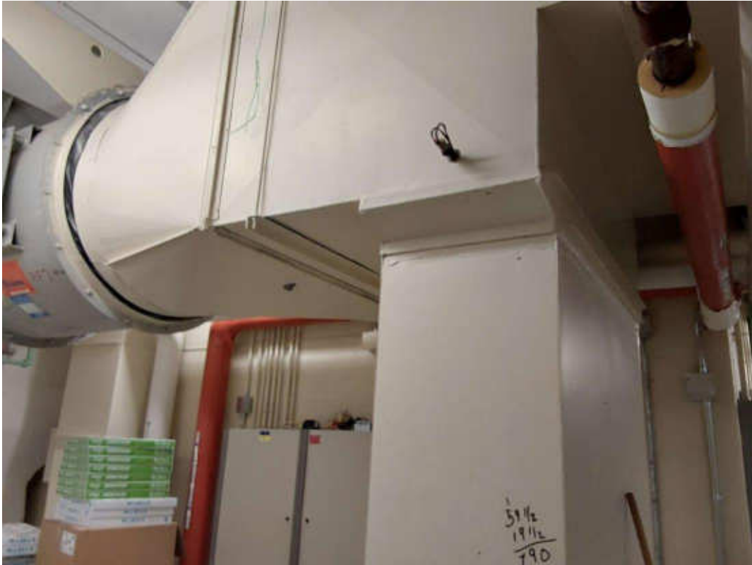
L0002(Lead, High), Beige paint on metal ducts, Duct, Mechanical Room (Location #: 2)
