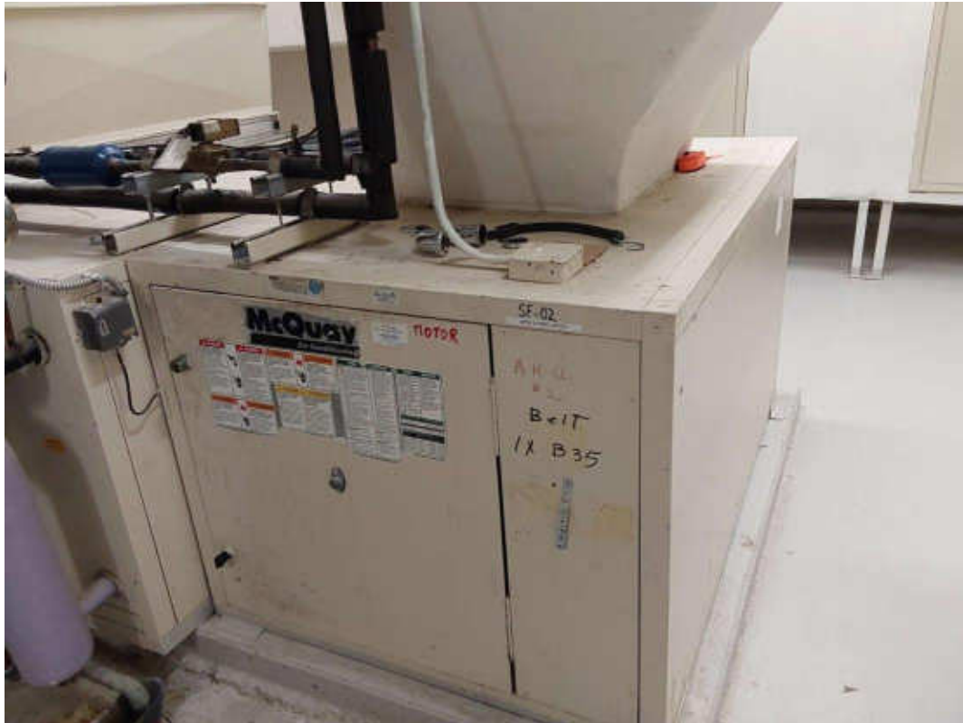
Mechanical Equipment, Air Handling Unit, Not Insulated, Mechanical Room (Location #: 2)
