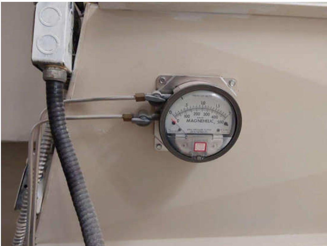
Mercury, V0000(No), MANOMETER, Non-mercury fluid, Mechanical Room (Location #: 2)
