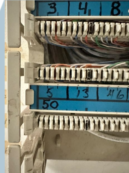
Cat6 voice termination into the Bell Bix block
