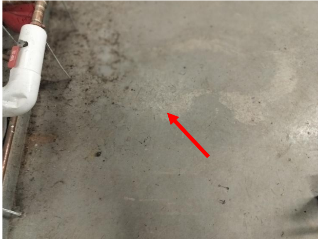
Photo 1: View of the lead containing grey paint (see arrow) observed to be in good condition on the concrete floor within Mechanical Room 2009.
