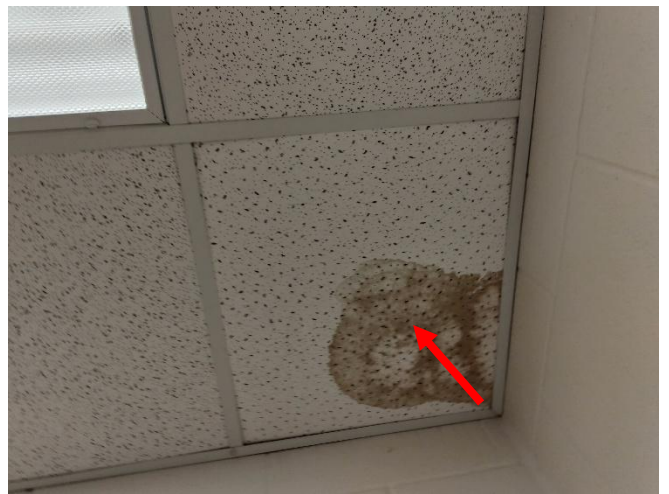
Photo 4: View of the apparent water staining on an acoustic ceiling tile (see arrow) observed in Science Classroom 2015.
