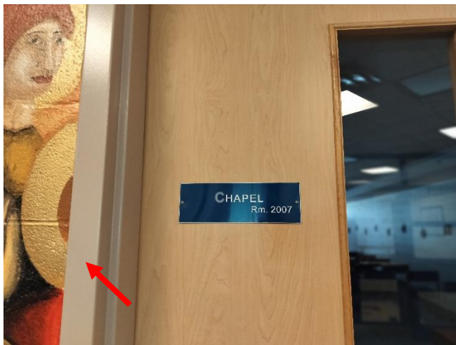
Photo 3: View of the lead containing dark beige paint (see arrow) observed to be in good condition on the door frame of Chapel Rm. 2007.
