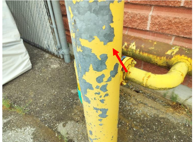
Photo 2: View of the lead containing yellow paint (see arrow) observed to be in fair condition on the concrete poles outside receiving doors.
