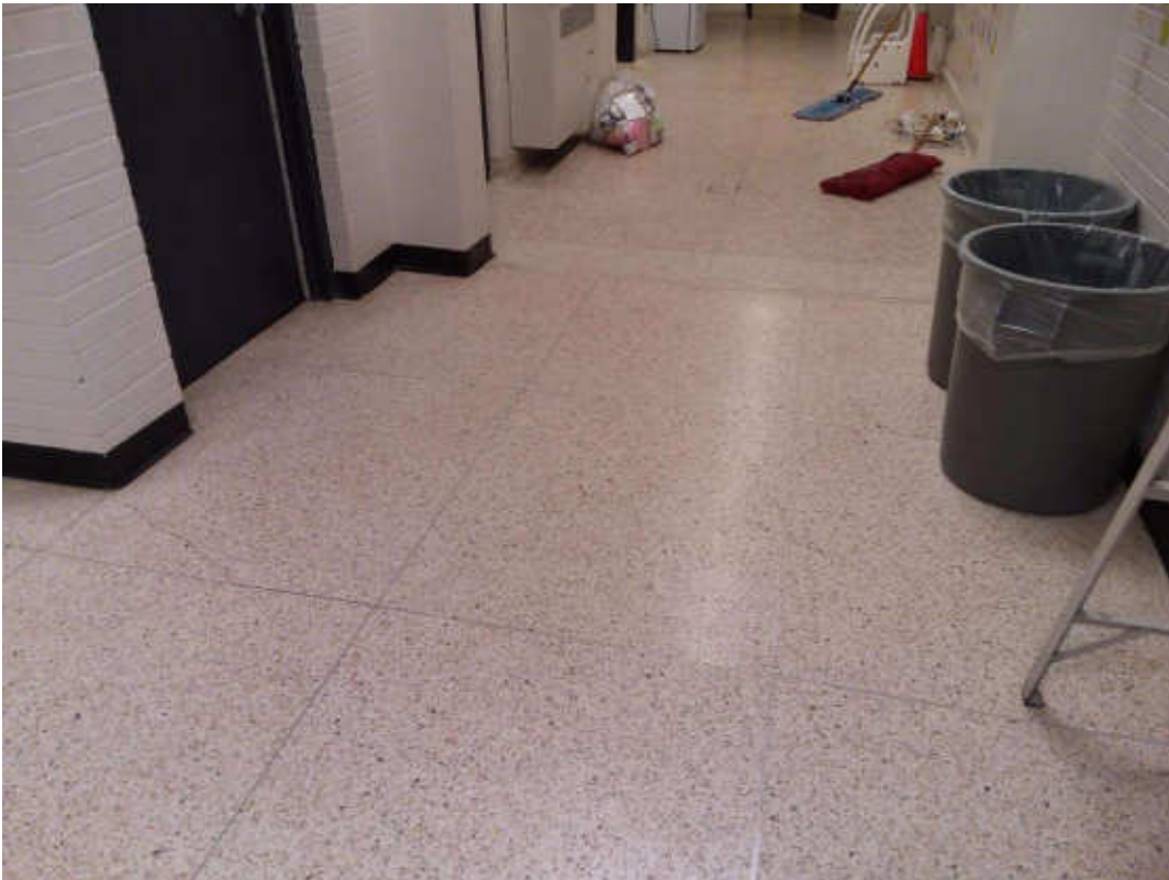
V9500 (Presumed Asbestos), Floor, Terrazzo, Ramp & Corridor (Location #: 35)
