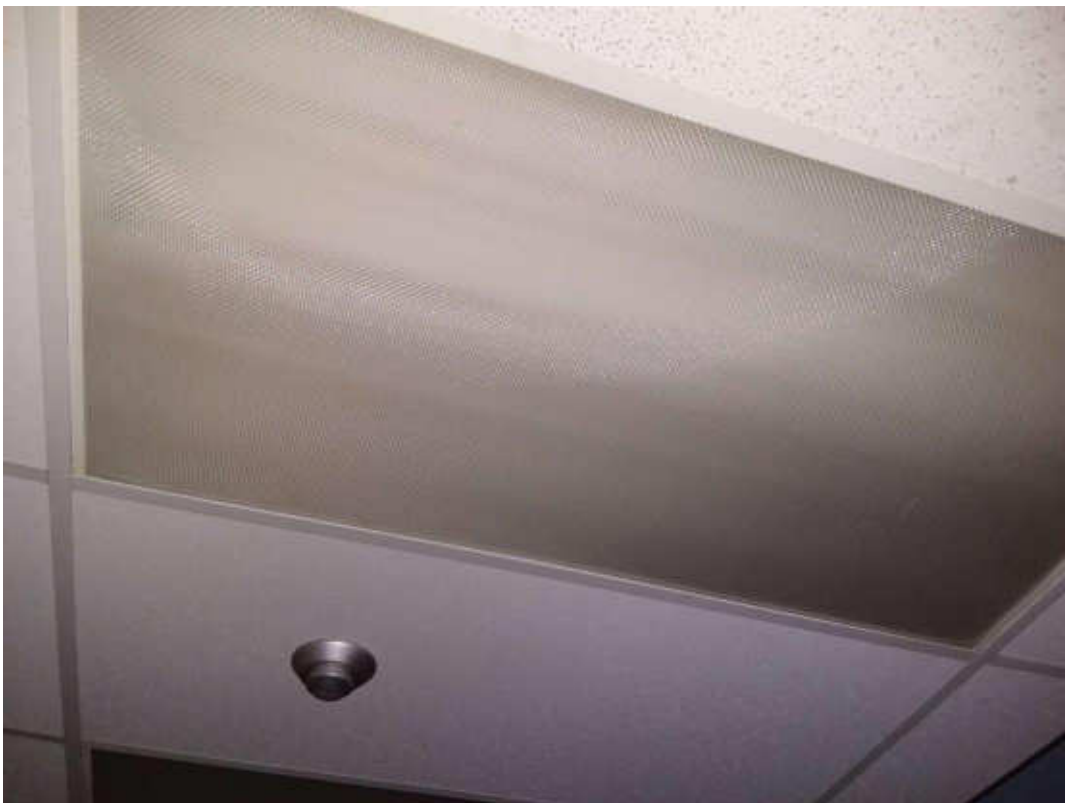
PCB, V9500(Presumed), LIGHT BALLASTS, Copier Room (Location #: 15)
