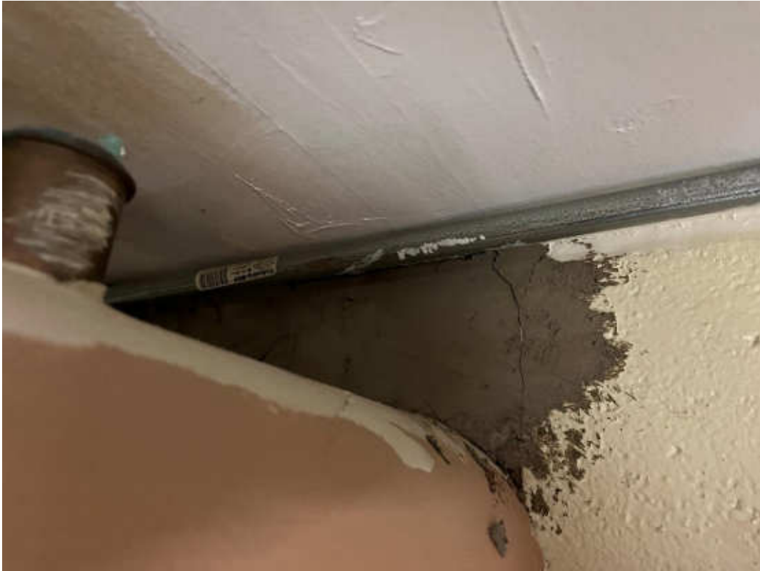
S0072C (None), Cementitious Firestopping, Other, Boiler Room (Location #: 1)
