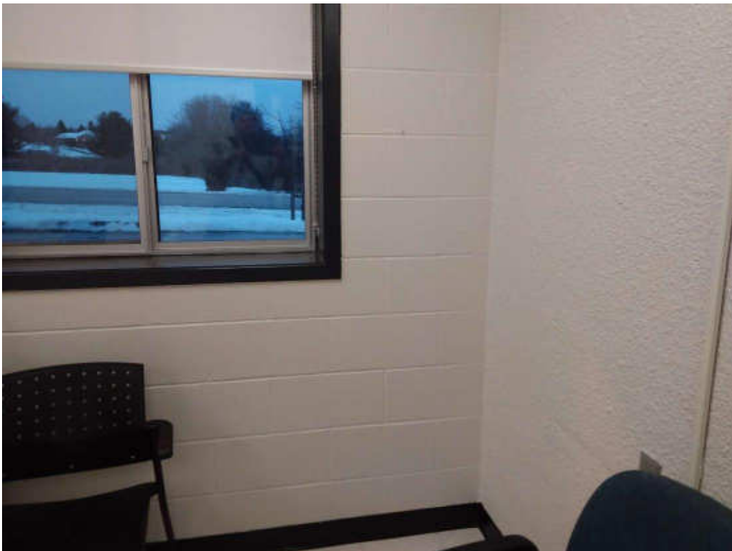
S0067A (Confirmed Asbestos), Beige/white paint on masonry, Wall, Paint, Meeting Room (Location #: 12)
