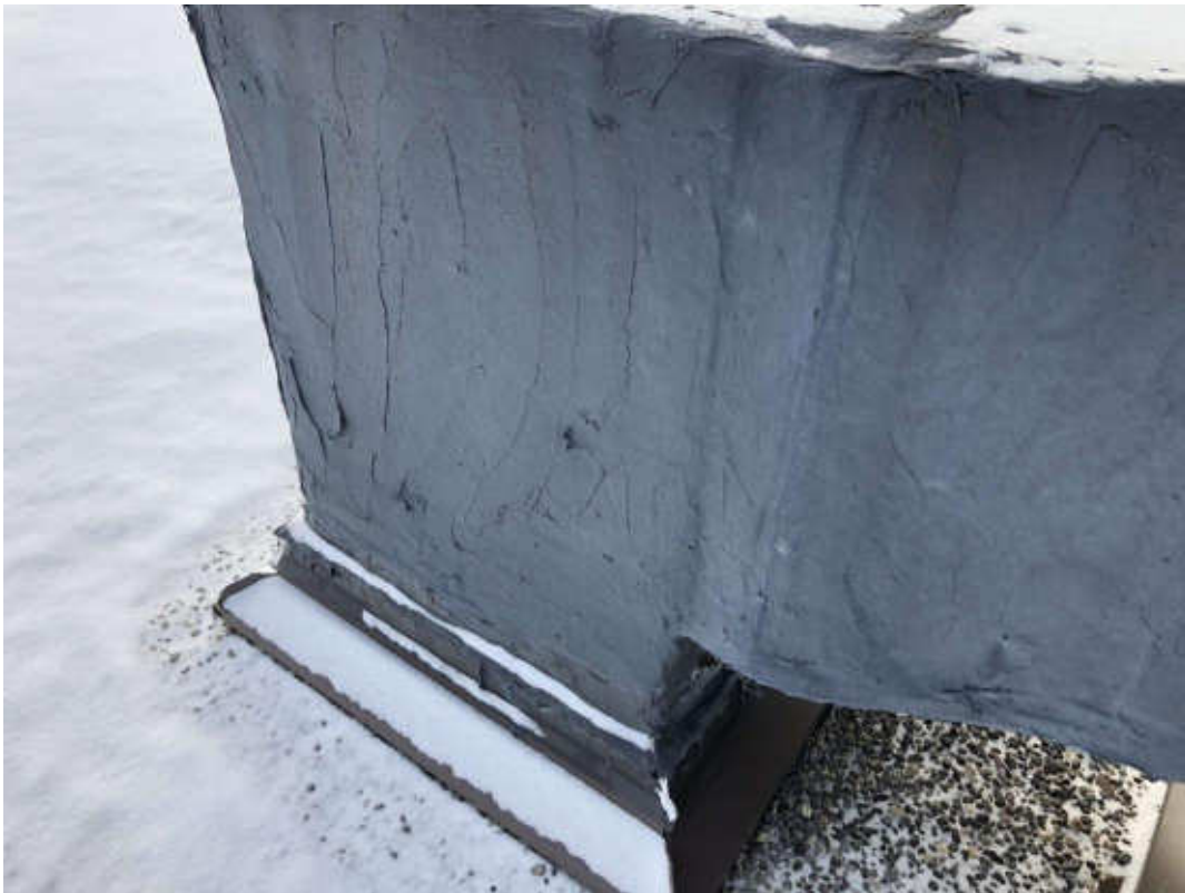
S0069C (Confirmed Asbestos), Tar On AHU Ducting, Mechanical Equipment, Air Handling Unit, Tar, Roof (Location #: 65)
