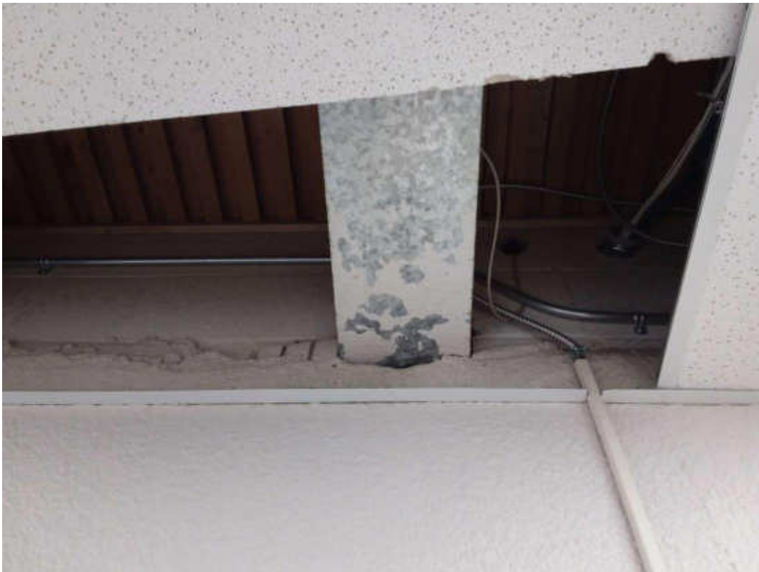
V0002 (Confirmed Asbestos), Texture coat overspray, Duct, Overspray, Meeting Room (Location #: 12)
