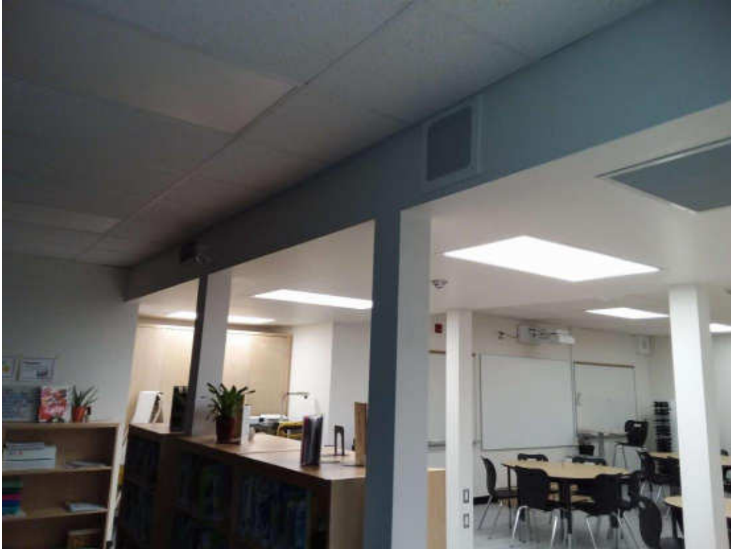
S0038A (Confirmed Asbestos), DJC ceiling/bulkhead, Ceiling, All, Drywall and joint compound, Library/Resource Room (Location #: 33)
