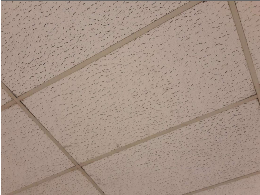
V0000 (None), Ceiling, Ceiling Tiles (lay-in), 2'x4' lay-in, fissures across length, 204 (Location #: 2040) Previous samples ASB-103.1-3
