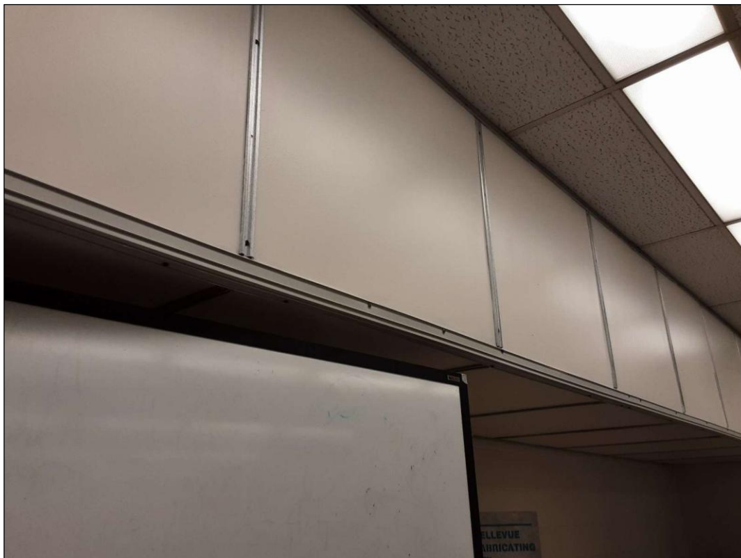
L0009(Lead, None), Ceiling, Drywall (no compound), Off-white, 204 (Location #: 2040)
