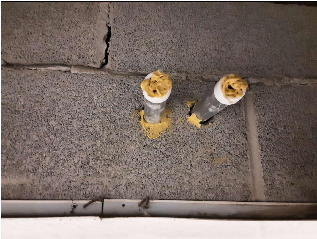
S0023A (None), Other, Firestopping (mastic), Yellow, 204 (Location #: 2040)
