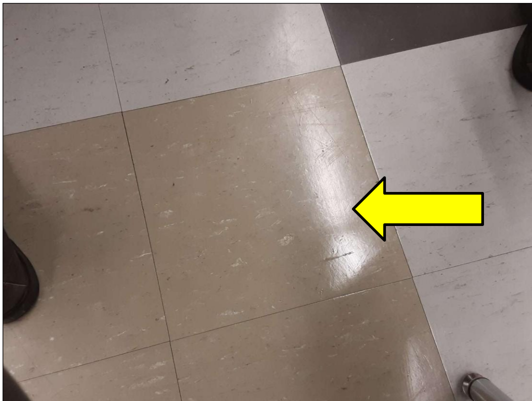
V9000 ( Confirmed Asbestos ), , Vinyl Floor Tile, VT-5, 12x12 pale green, Floor 204 (Location #: 2040) Previous samples ASB-125.1-3
