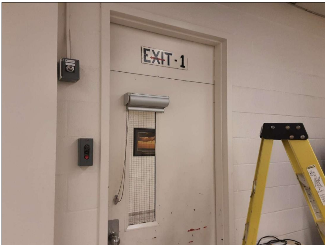
L0010(Lead, High), Wall, Metal, Red/white on door and frame, 204 (Location #: 2040)
