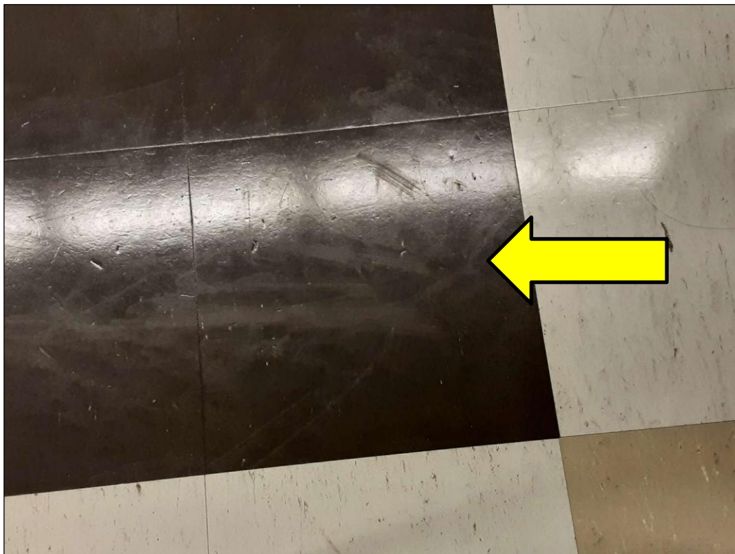
V9000 (Confirmed Asbestos), Floor, Vinyl Floor Tile, VT-10, 12x12 grey, 204 (Location #: 2040) Historic Data
