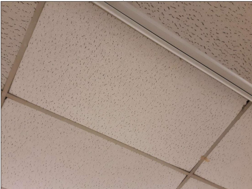
V0000 (None), Ceiling, Ceiling Tiles (lay-in), 2'x4' lay-in, fissures across width, 204 (Location #: 2040) Previous samples ASB-104.1-3
