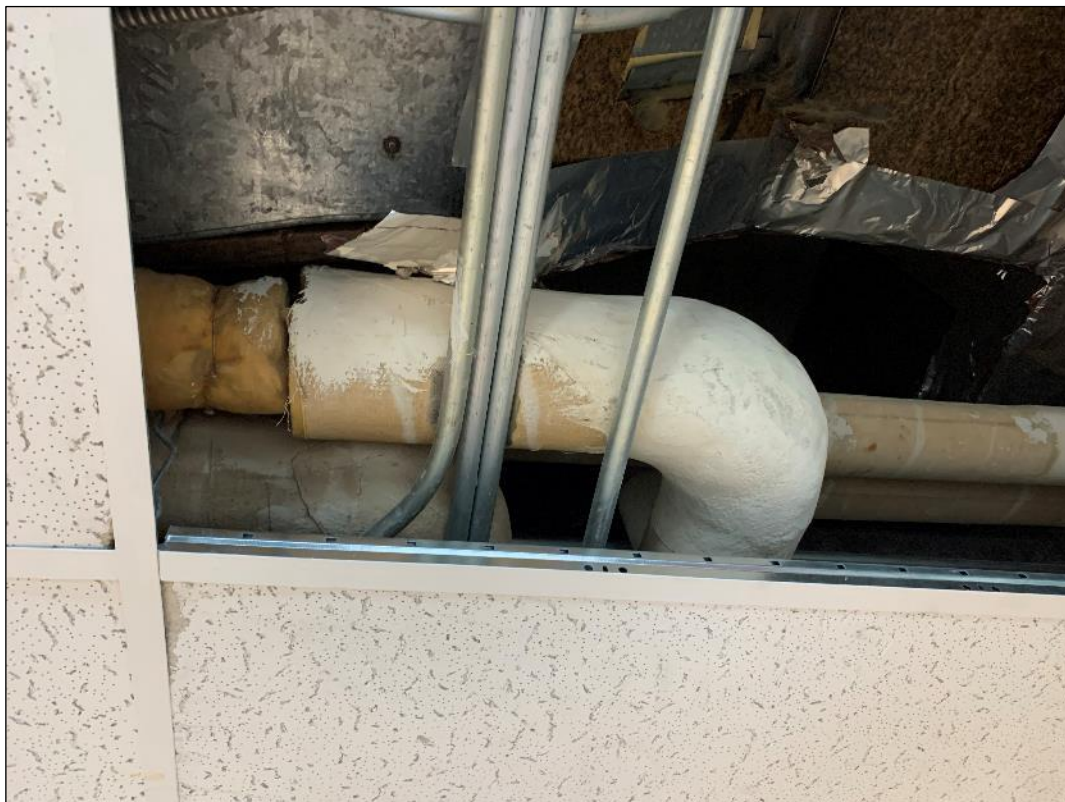
Damaged asbestos-containing parging cement insulation present on pipe end in Room 134A (Location #1870).
