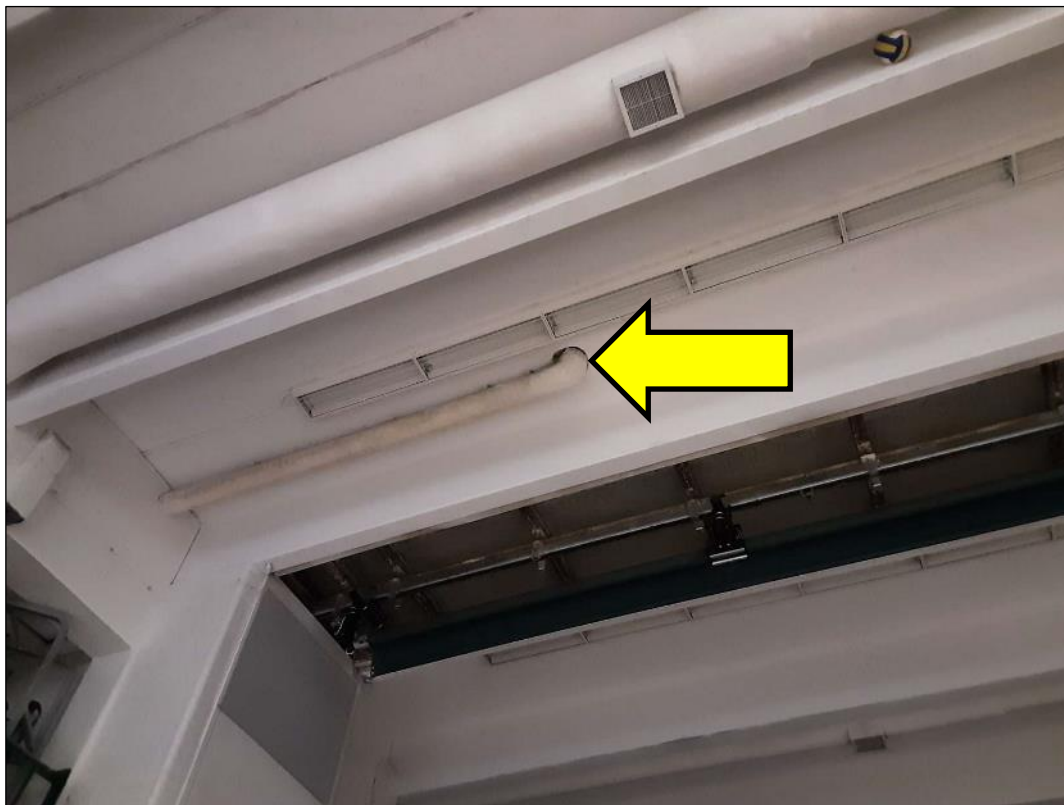
V0006 - (Confirmed Asbestos) Piping, Parging Cement, Gym 148 (Location #: 1620)
