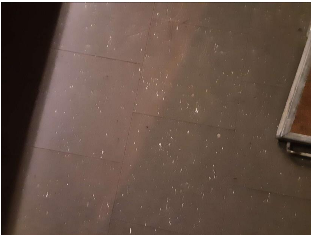
V9000 - (Confirmed Asbestos), Vinyl Floor Tile, VT-9, 12"x12" Off-White, 113 (Location #: 1100) Historic data
