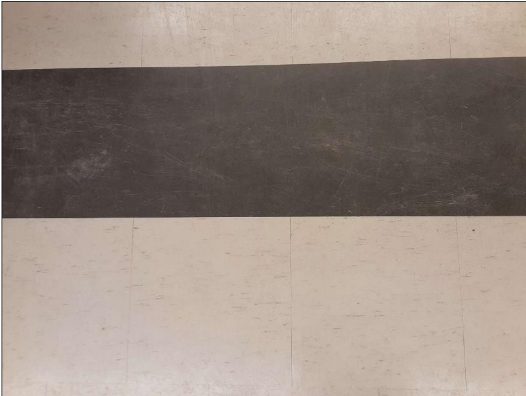
V9000 - (Confirmed Asbestos), Vinyl Floor Tile, VT-9, 12"x12" Off-White, 113 (Location #: 1100) Historic data
