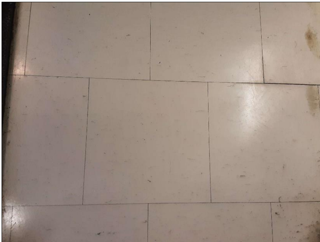
V9000 - (Confirmed Asbestos), Vinyl Floor Tile, VT-1, 12"x12", Off-White with Fine Black Streaks, 152F (Location #: 1774) Historic data
