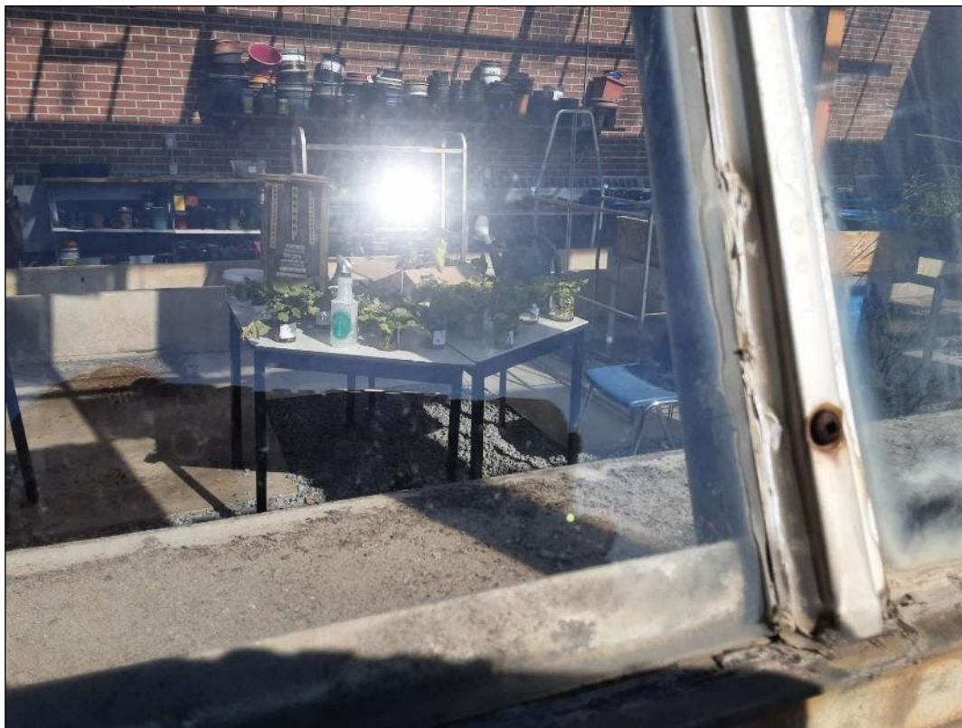
V9000 - (Confirmed Asbestos), Window, Putty, White, 160 (Location #: 1670) Greenhouse, Historical data
