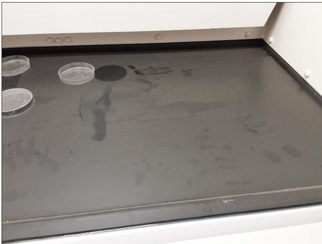
V9500 - (Presumed Asbestos) Other, Countertop, Cement Product (Transite), 156 (Location #: 1690)
