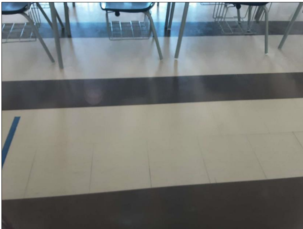
V9000 - (Confirmed Asbestos), Vinyl Floor Tile, VT-1, 12"x12", Off-White with Fine Black Streaks, 152F (Location #: 1774) Historic data
