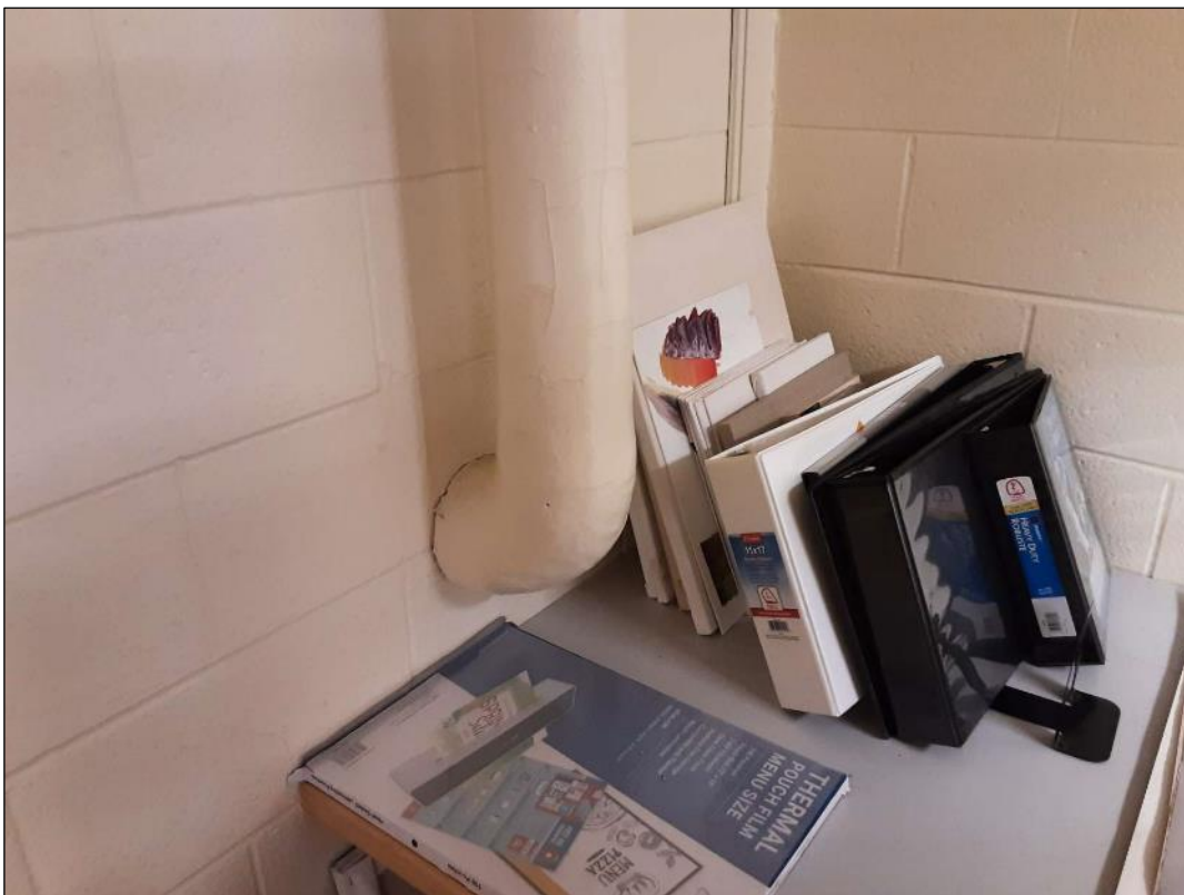
V0006 - (Confirmed Asbestos) Piping, Parging Cement, 136 (Location #: 1851)
