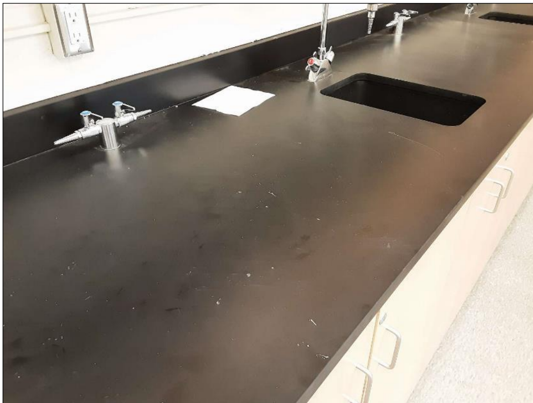
V9500 - (Presumed Asbestos) Other, Countertop, Cement Product (Transite), 156 (Location #: 1690)
