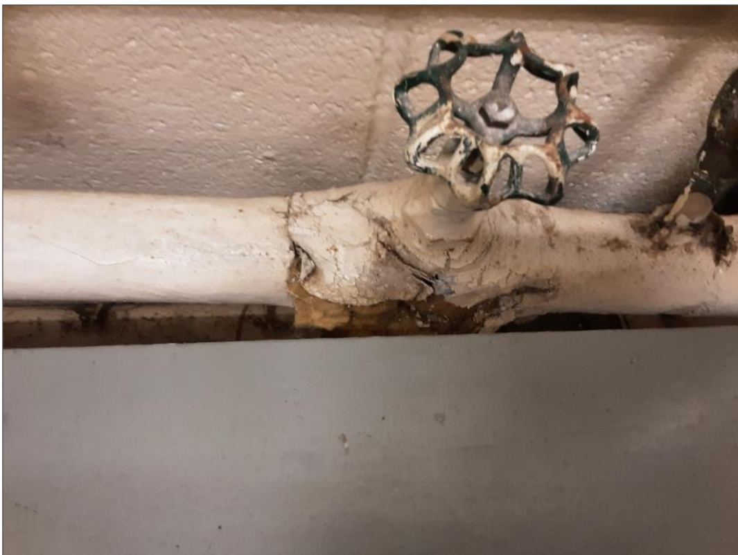
Damaged asbestos-containing parging cement insulation present on valve in Room 120A (Location #1433).
