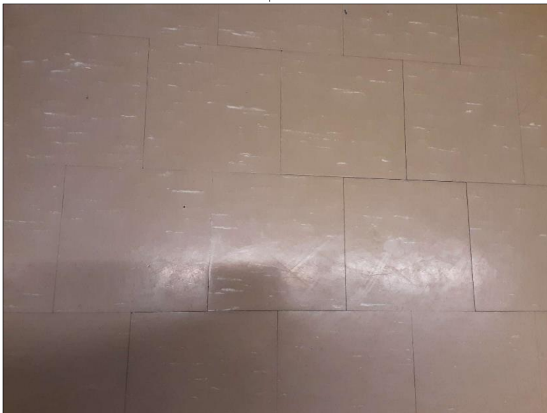
V9000 - (Confirmed Asbestos), Vinyl Floor Tile, VT-2, 9"x9", Dark Grey, 164 (Location #: 1650) Previous samples ASB-121.1-3
