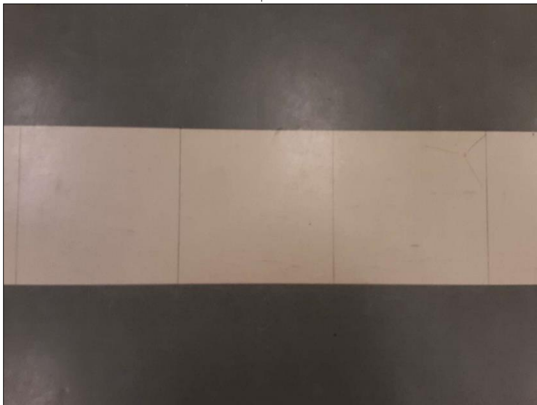
V9000 - (Confirmed Asbestos), Vinyl Floor Tile, VT-8, 12"x12", Tan with White and Brown Marks, 150 (Location #: 1640) Previous samples ASB-131.1-3
