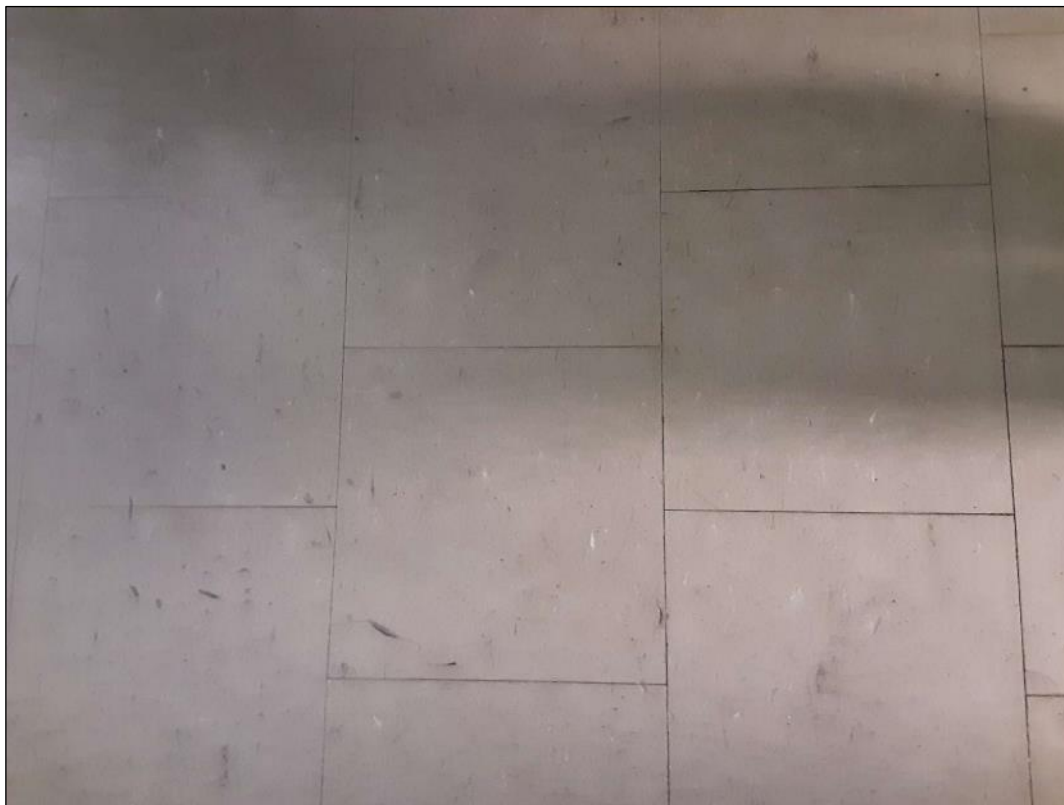
V9000 - (Confirmed Asbestos), Vinyl Floor Tile, VT-8, 12"x12", Tan with White and Brown Marks, 150 (Location #: 1640) Previous samples ASB-131.1-3
