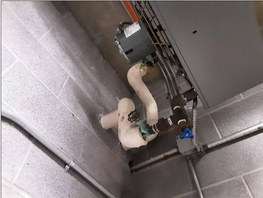
V0006 - (Confirmed Asbestos) Piping, Parging Cement, 240A (Location #: 2661)
