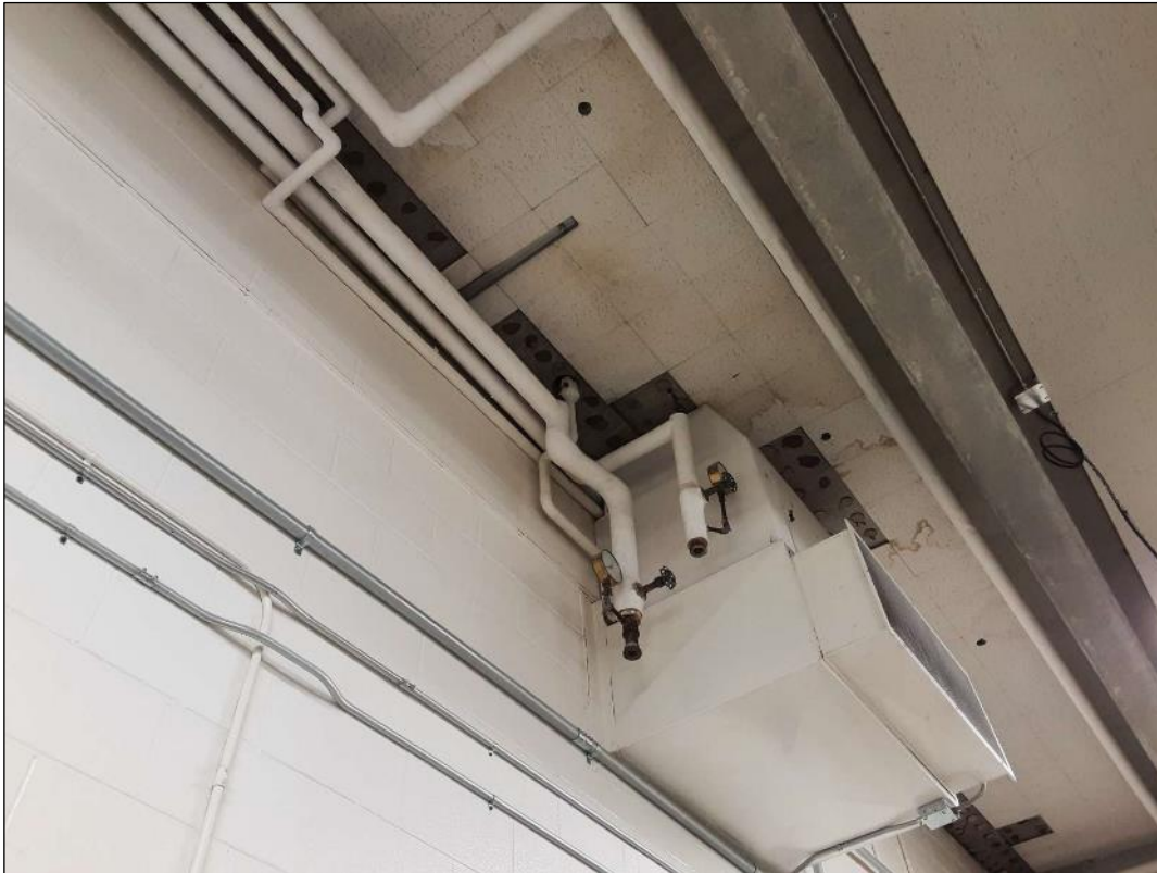
V0006 - (Confirmed Asbestos) Piping, Parging Cement, 136 (Location #: 1851)
