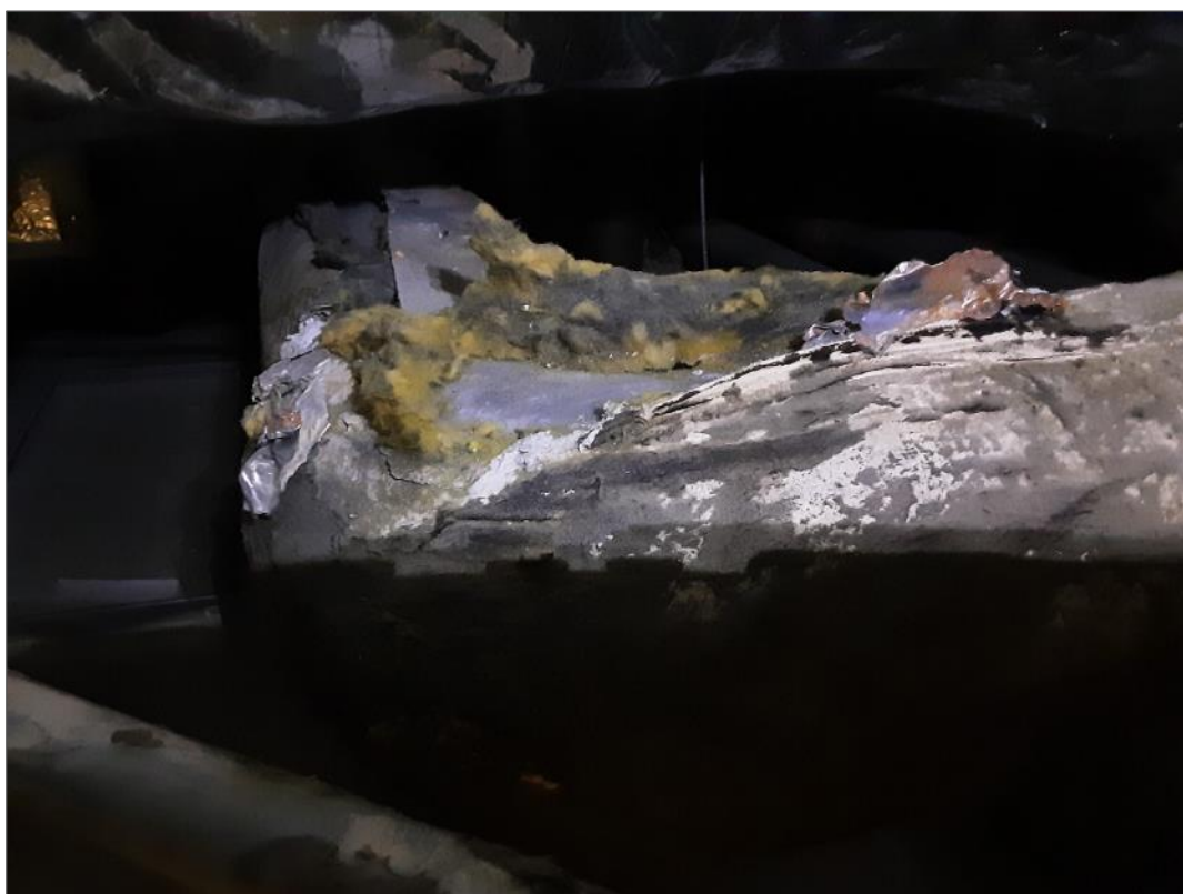
Damaged asbestos-containing parging cement insulation present on pipe end in Room 134A (Location #1870).
