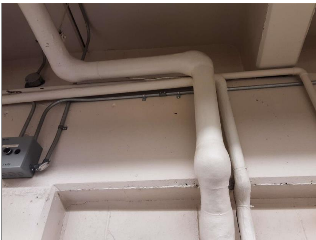
V0006 - (Confirmed Asbestos) Piping, Parging Cement, Gym 148 (Location #: 1620)
