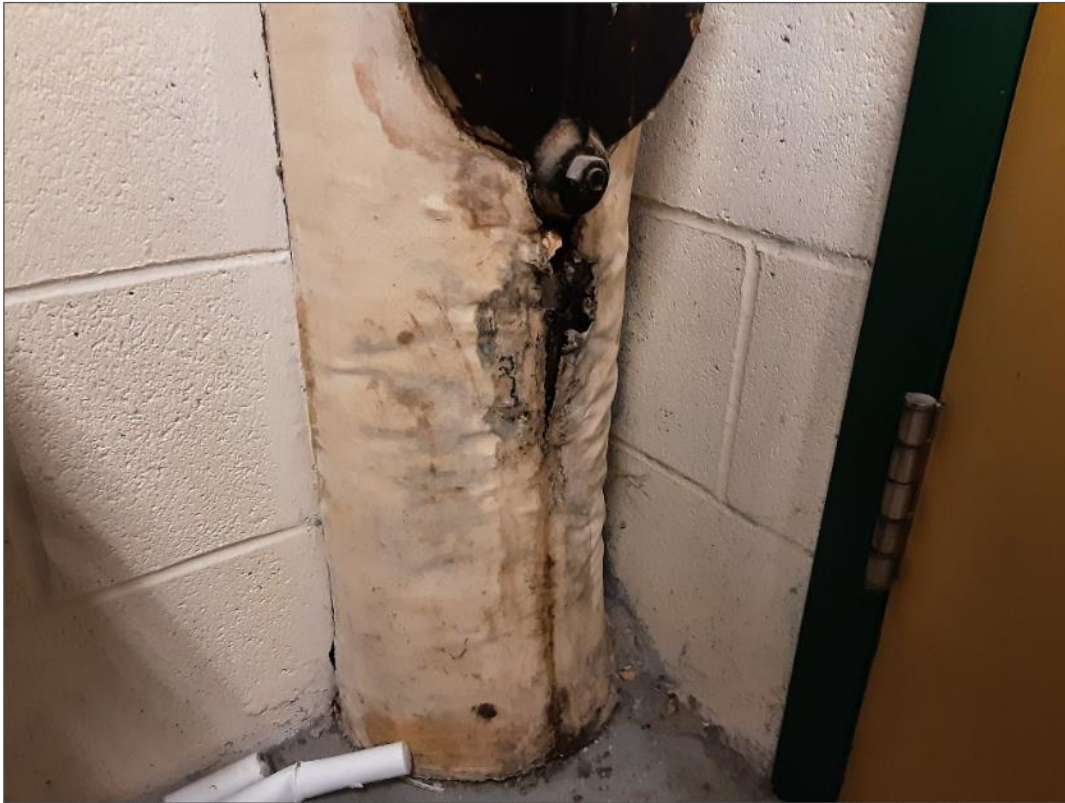
Damaged asbestos-containing parging cement insulation present on valve in Room 120A (Location #1433).
