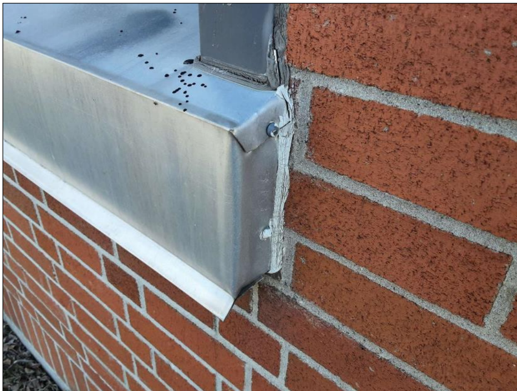
V9000 - (Confirmed Asbestos), Window, Caulking, Grey/White, South and West, Exterior (Location #: 0) Historic Data
