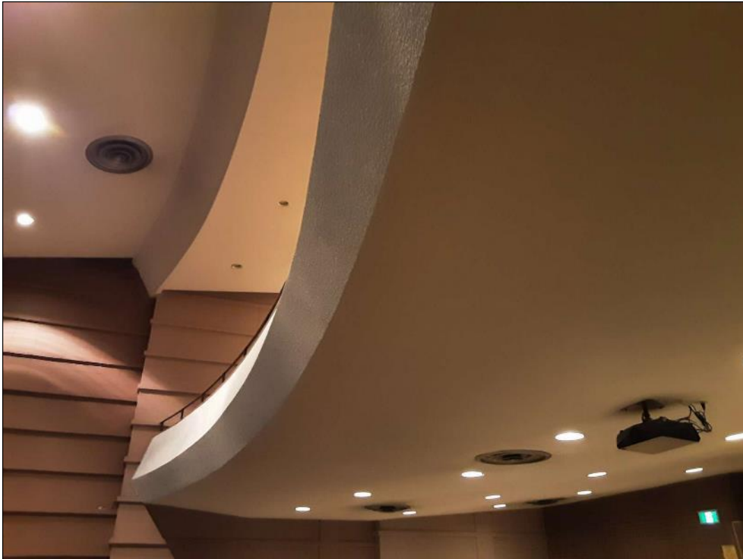
S0005A - (Confirmed Asbestos) Ceiling, Texture Coat, 101 (Location #: 1610)
