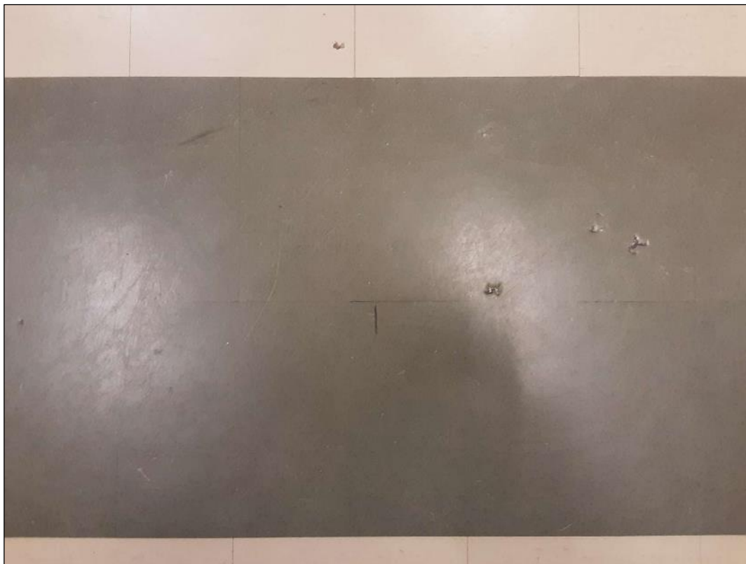
V9000 - (Confirmed Asbestos), Vinyl Floor Tile, VT-2, 9"x9", Dark Grey, 164 (Location #: 1650) Previous samples ASB-121.1-3
