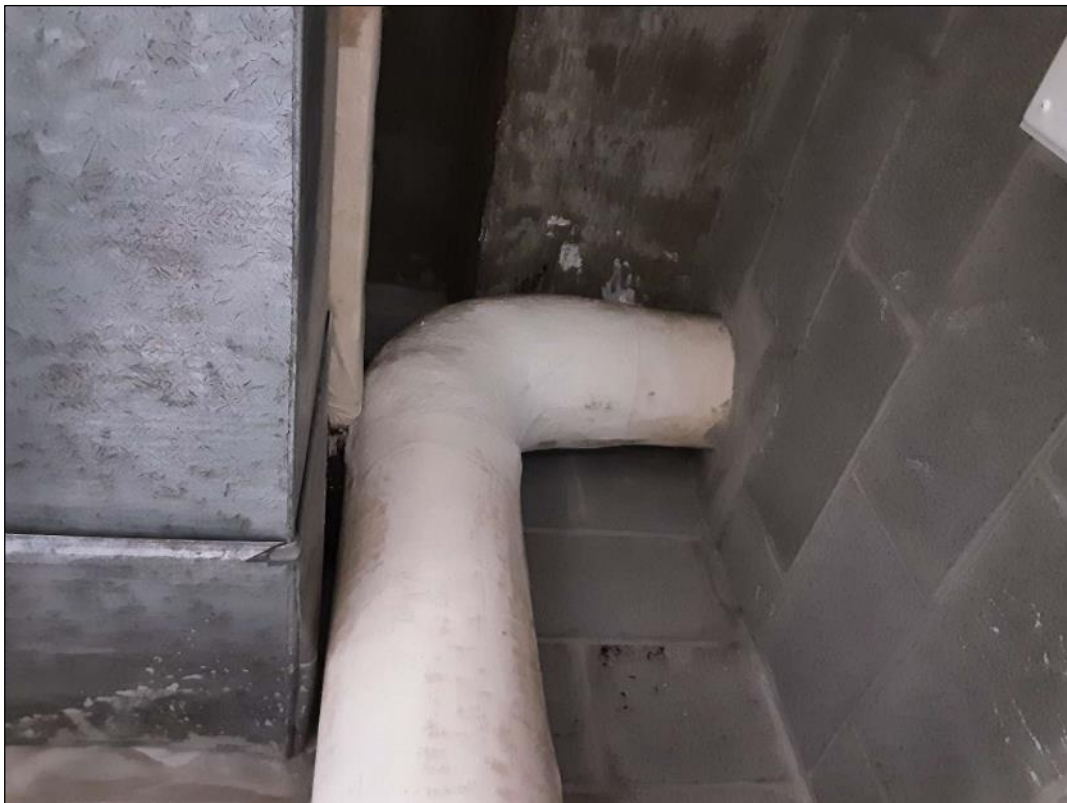
V0006 - (Confirmed Asbestos) Piping, Parging Cement, 240A (Location #: 2661)
