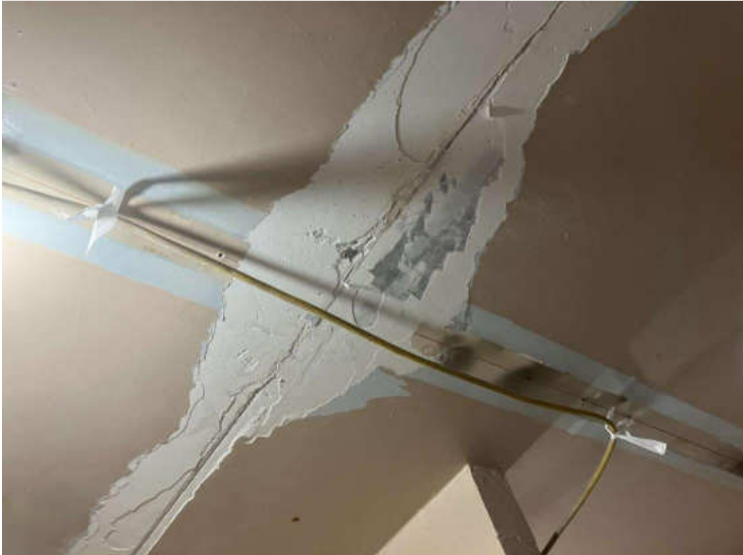
S0109A (None), Drywall on ceilings, Kitchen (Location #: 140)
