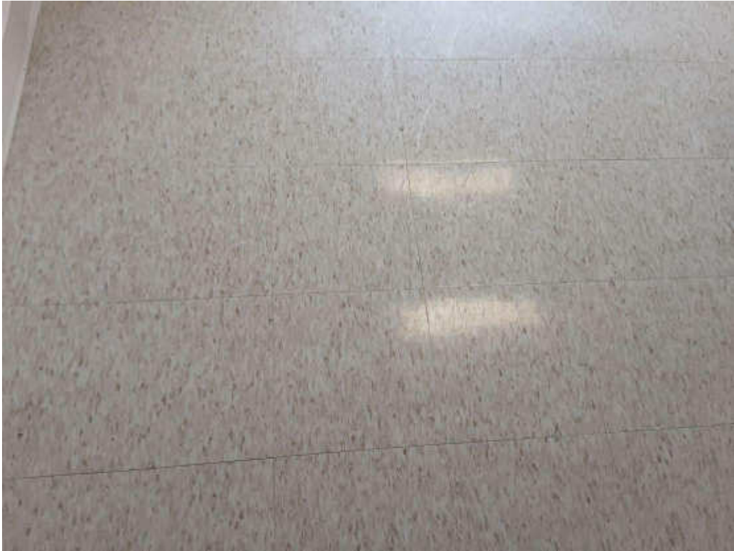
S0070A (None), Floor, Vinyl Floor Tiles and Mastic, Office (Location #: 161)
