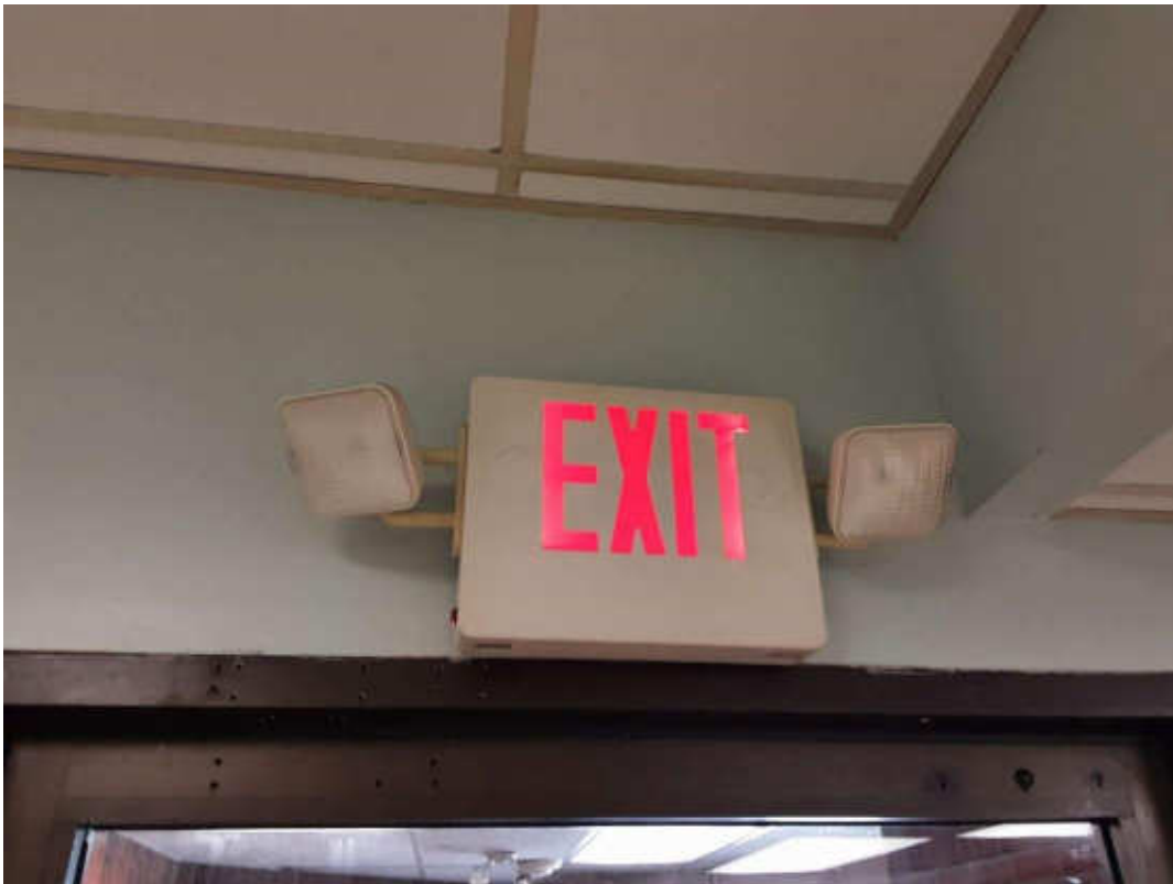
Pb Products, Lobby (Location #: 4)
