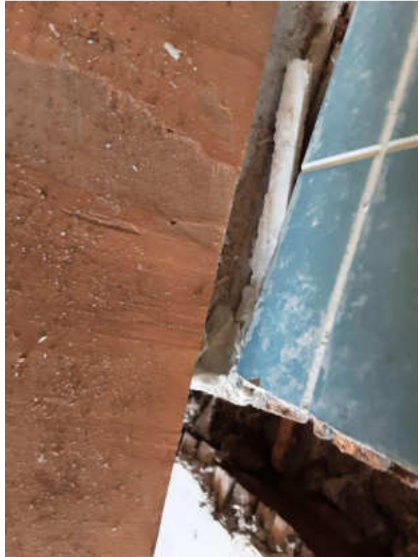
PCB, Old House - 2nd Floor (Location #: 178)
