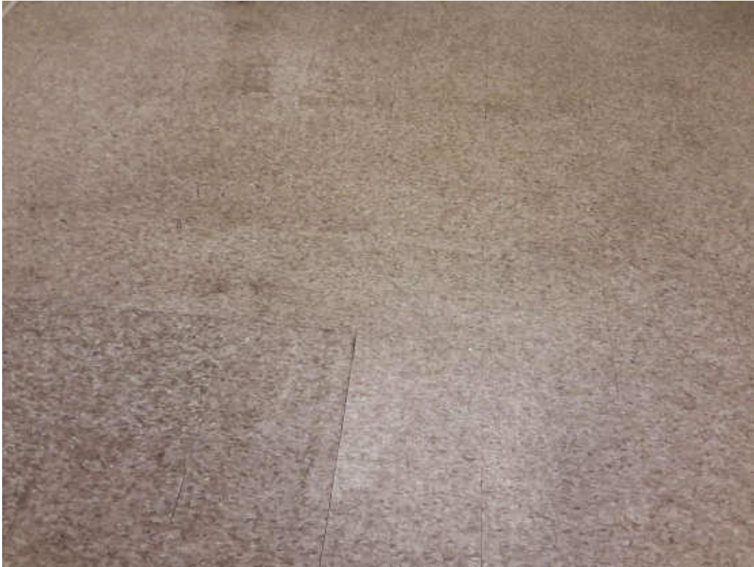
V0003 (None), Floor, Vinyl Floor Tiles and Mastic, Main Office (Location #: 5)
