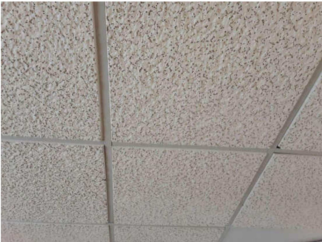
S0013A (None), Ceiling, Ceiling Tiles (lay-in), Office (Location #: 10)
