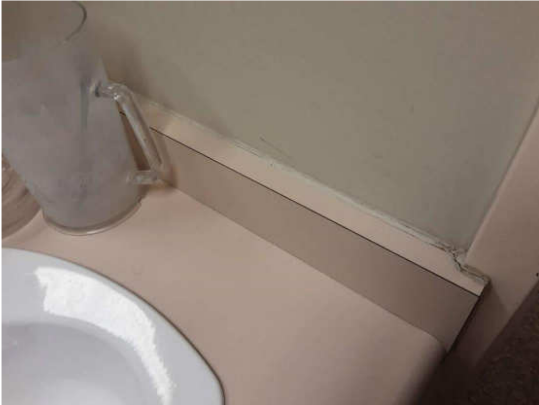
S0012A (None), Other, Caulking, Office (Location #: 9)
