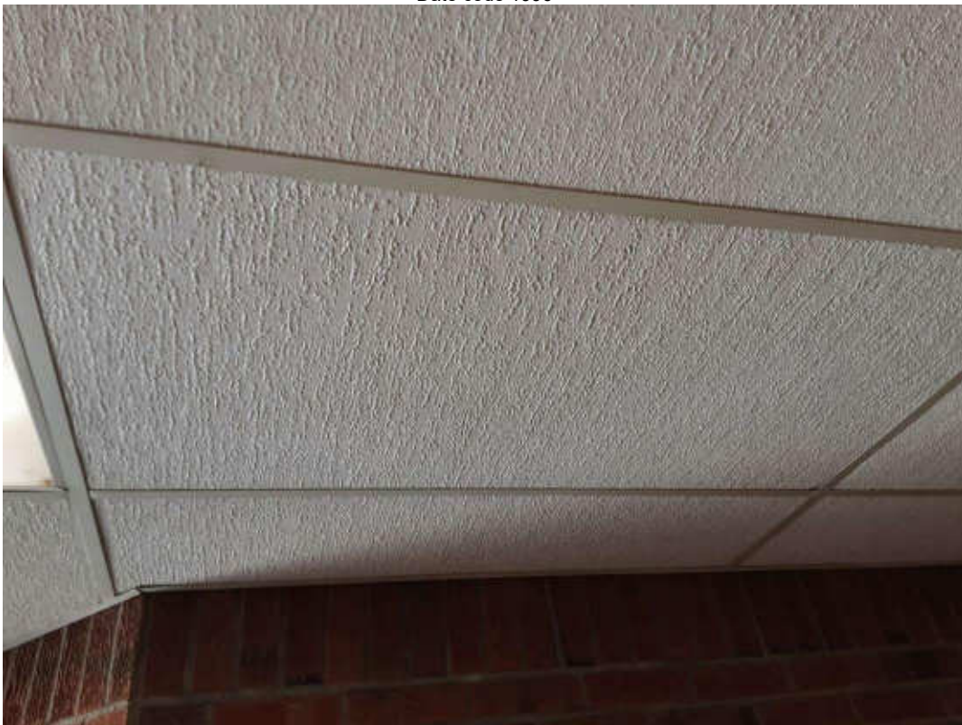
V0000 (None), Ceiling, Ceiling Tiles (lay-in), Vestibule (Location #: 3) Fiberglass
