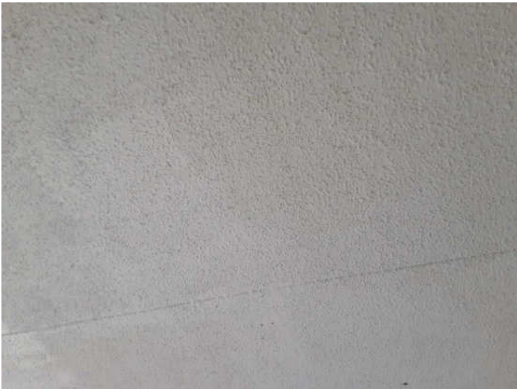
S0051A (None), Ceiling, Texture Coat, Medical Supply (Location #: 174)
