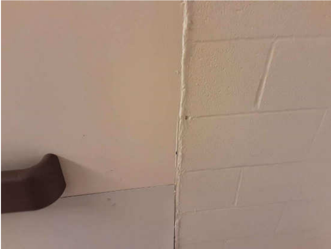
S0049C (None), Wall, Expansion Joint, Caulking, North Corridor (Location #: 106)
