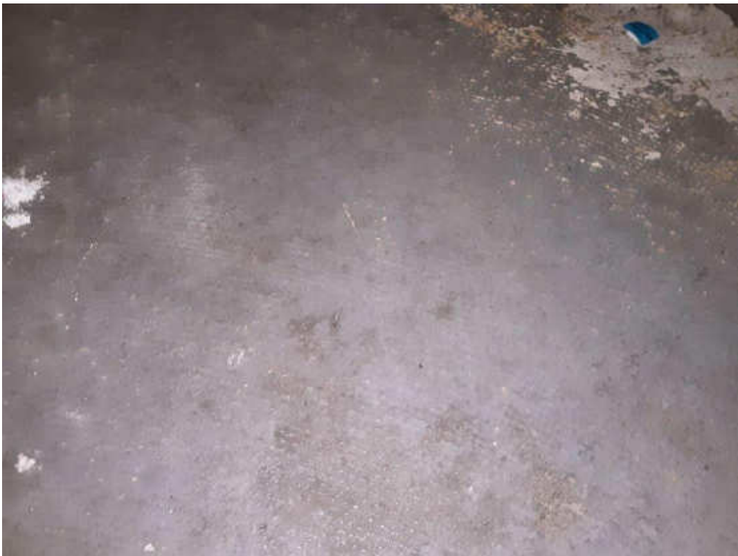
S0058C (None), Floor, Mastic, Storage (Location #: 163)
