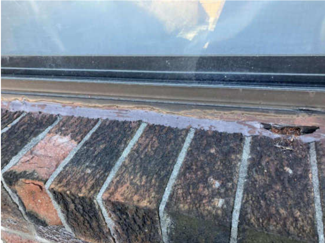
S0097C (None), Light grey caulking along exterior windows, Other, Caulking, Exterior (North Wing) (Location #: 1)
