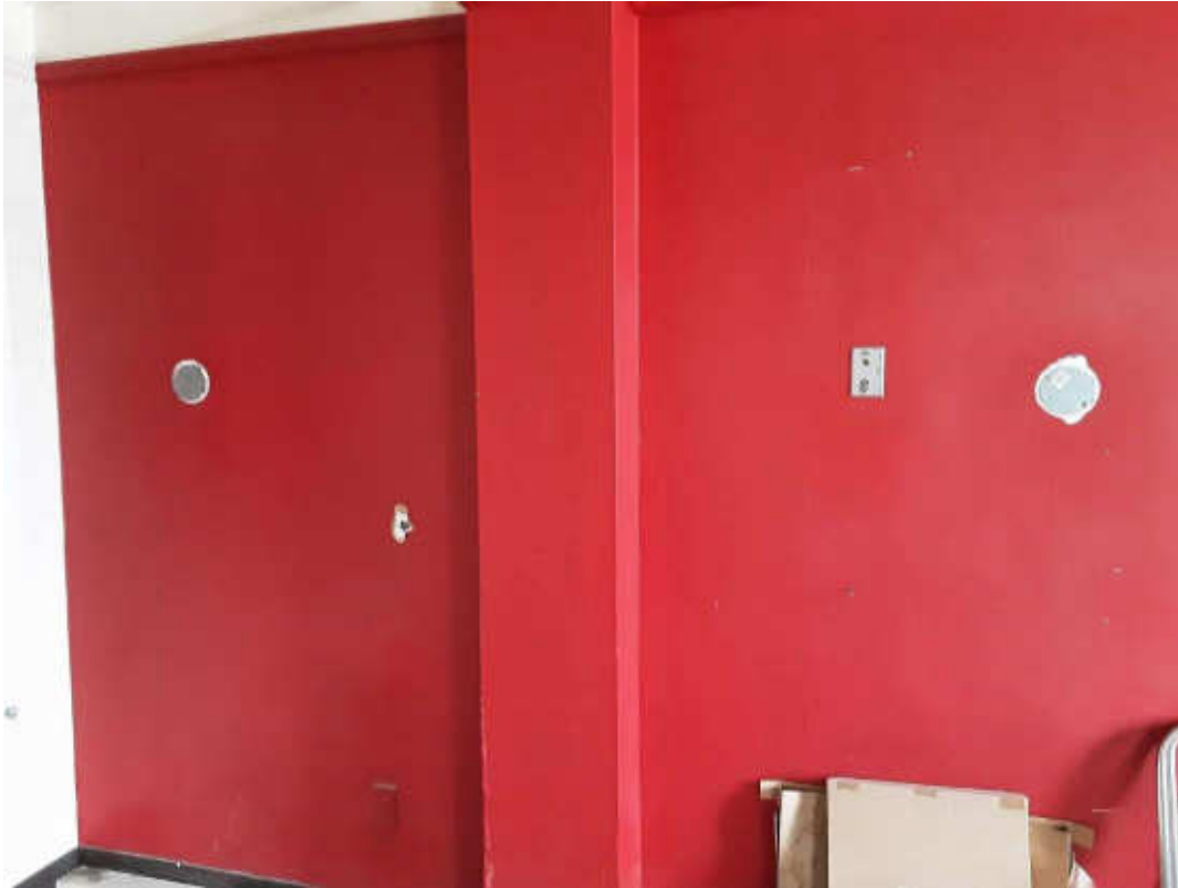
Drywall and joint compound, Red, L0017(Lead (High)), Old House - Ground Floor (Location #: 177)
