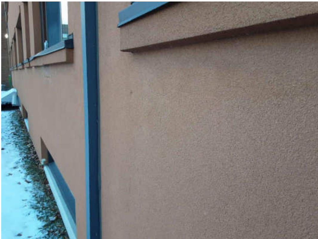
S0086G (None), Brown stucco, Wall, Stucco, Exterior (Location #: 1)
