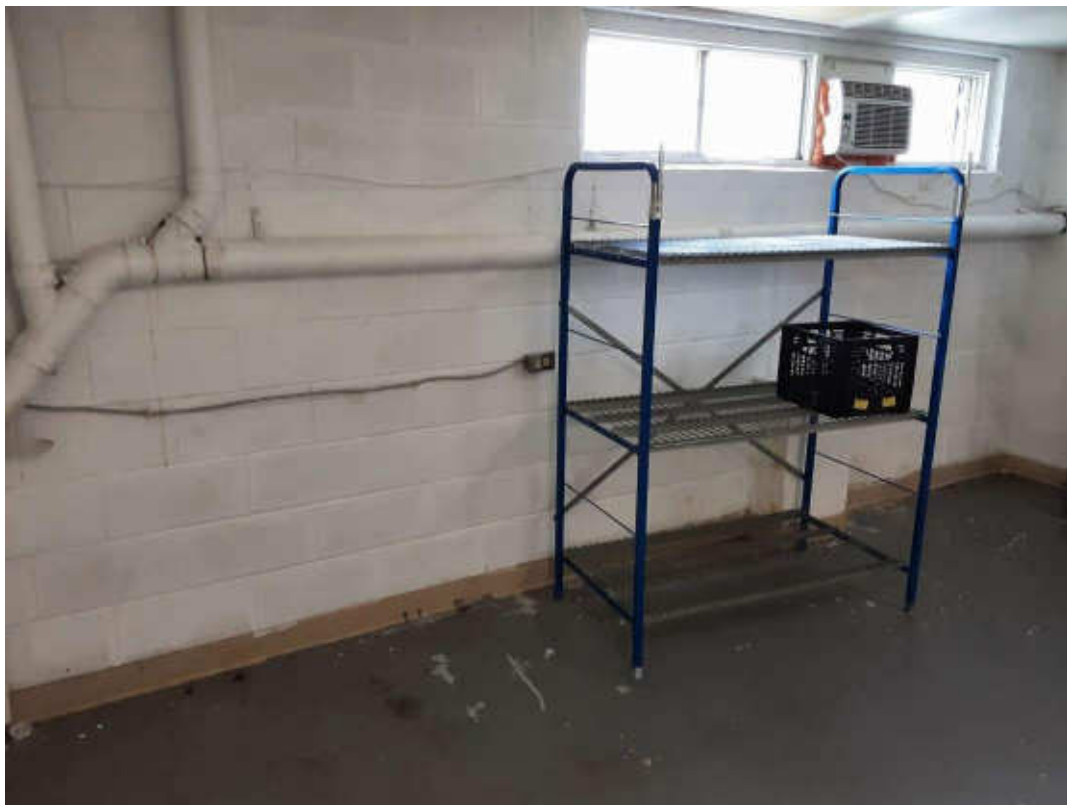
V9000 (Confirmed Asbestos), Piping, Rainwater Leader, Transite Cement, Dietary Storage (Location #: 130)
