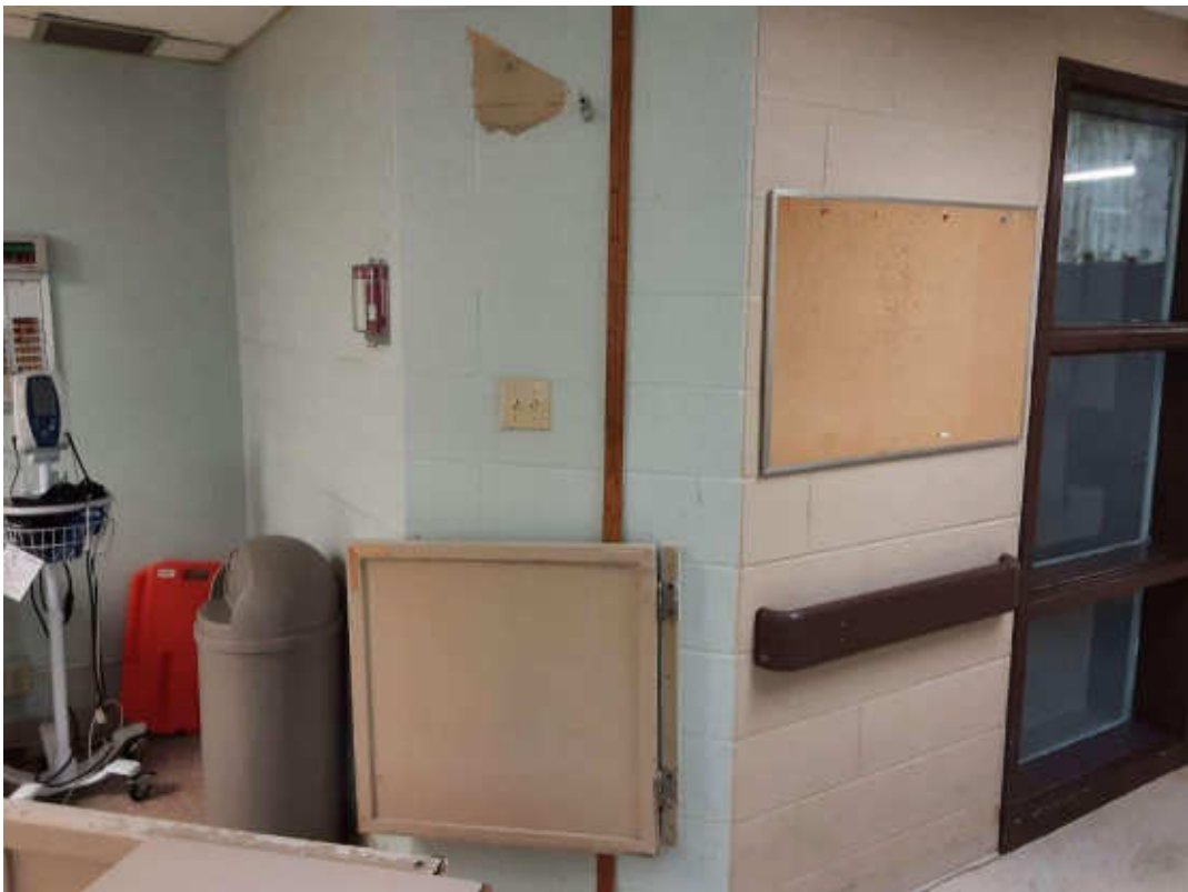
S0007A (None), Wall, Paint, Lobby (Location #: 4)
