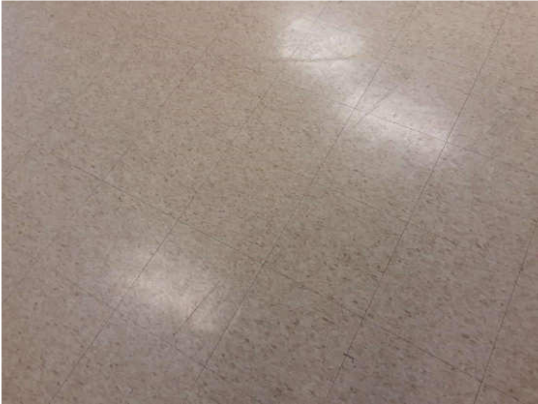
S0001A (None), Floor, All, Vinyl Floor Tiles and Mastic, Lobby (Location #: 4)
