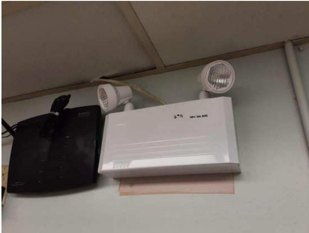
Pb Products, Lobby (Location #: 4)
