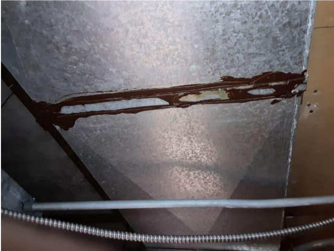
S0029A (None), Duct, Caulking, North Corridor (Location #: 57)
