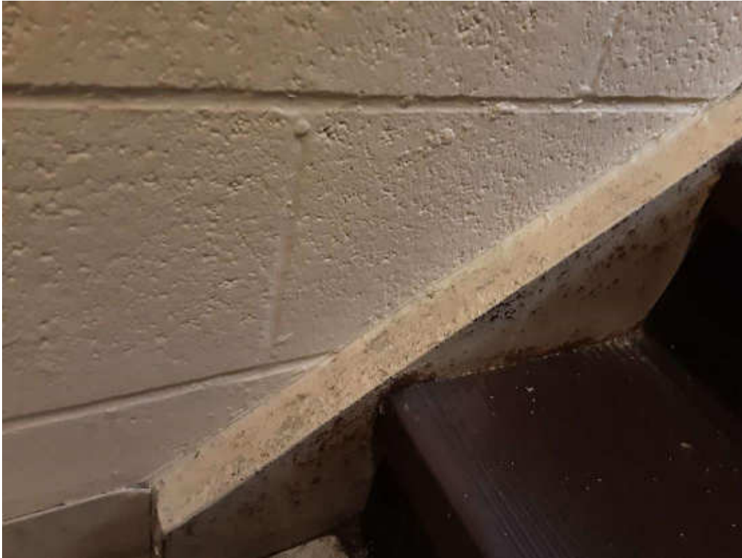
S0047A (None), Structure, Caulking, South Stairwell (Location #: 143)
