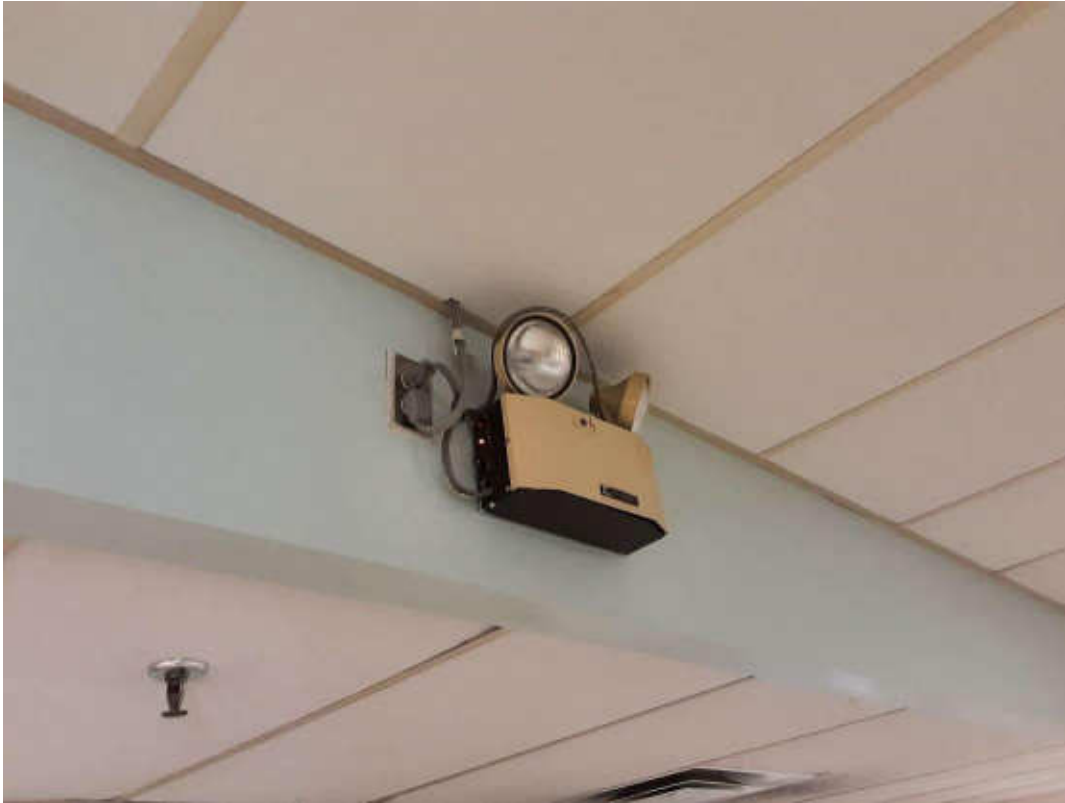
Pb Products, Lobby (Location #: 4)
