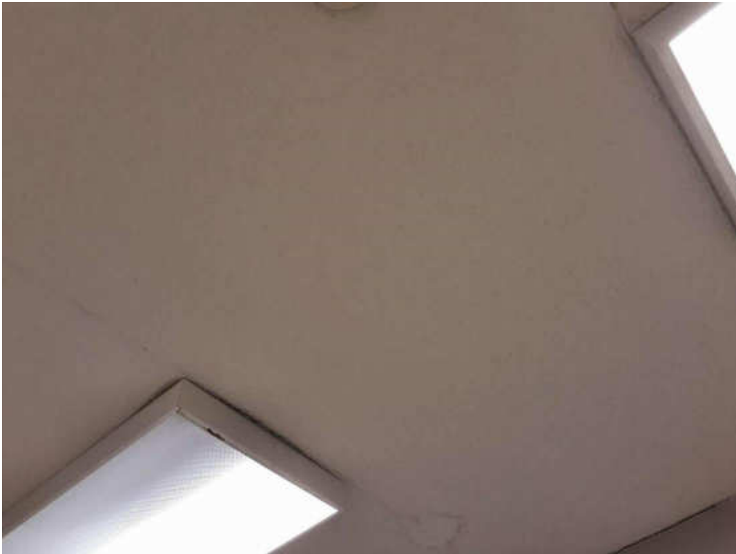
S0008A (None), Ceiling, Texture Coat, Main Office (Location #: 5)
