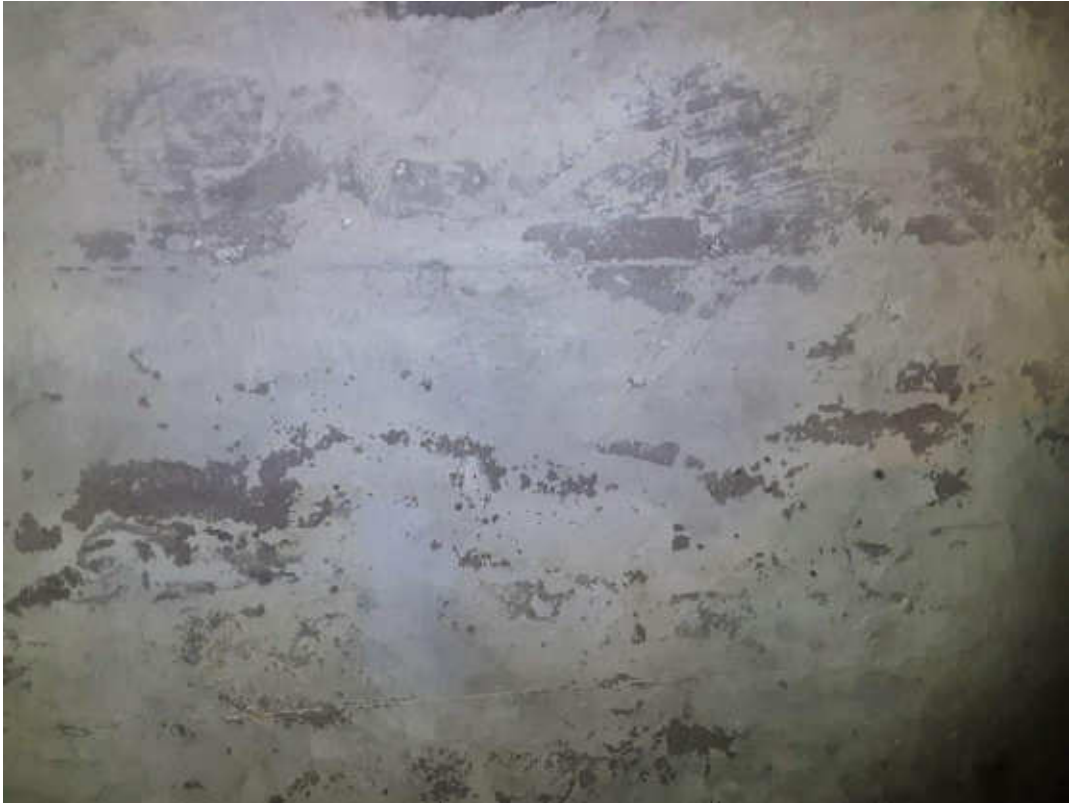
S0041A (None), Wall, Plaster, Old House - Basement (Location #: 135)
