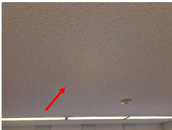
Photo 2: View of the asbestos containing white texture coating (see arrow) observed to be in good condition throughout the 1967 section of the Subject Building.
