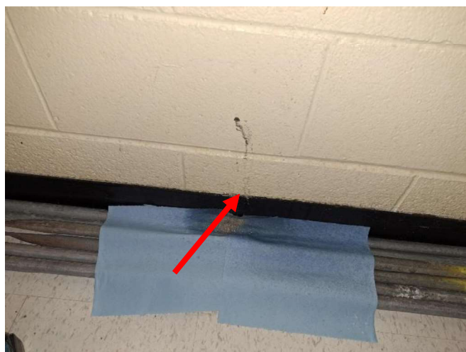
Photo 11: View of the concrete block wall during the vermiculite investigation and drilling activities (see arrow) within Classroom 8 of the 1962 section of the Subject Building.
