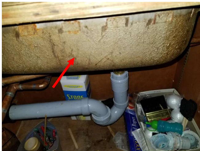
Photo 4: View of the asbestos containing gold sink coating (see arrow) observed to be in good condition within Classroom 3 of the 1967 section of the Subject Building.
