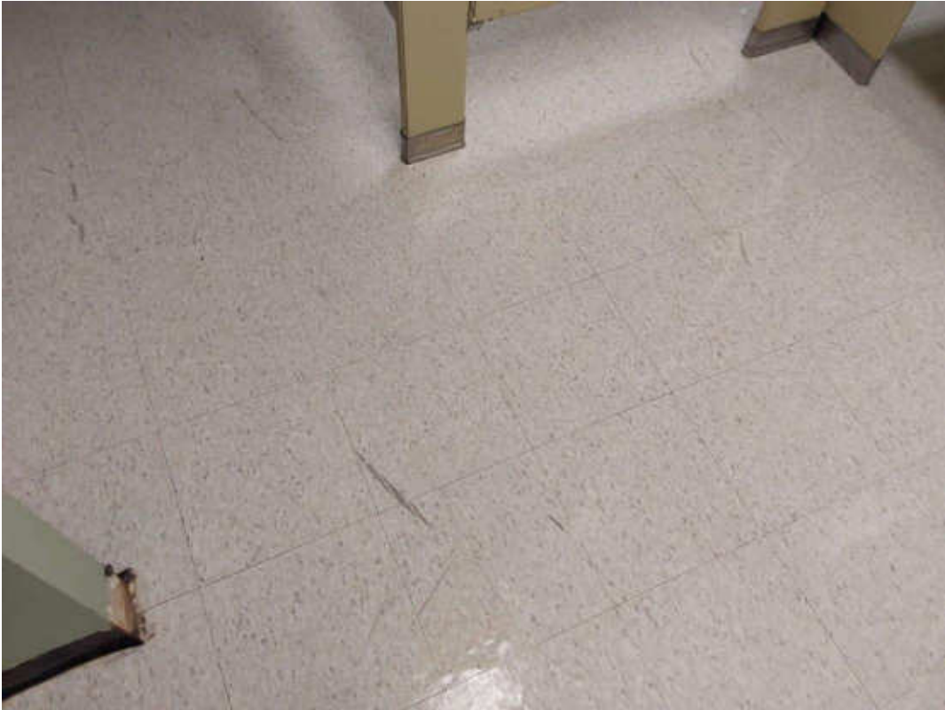
S0001B (None), 12" x 12" grey mottled, Floor, Vinyl Floor Tile and Mastic, Men's Washroom (Location #: 1)
