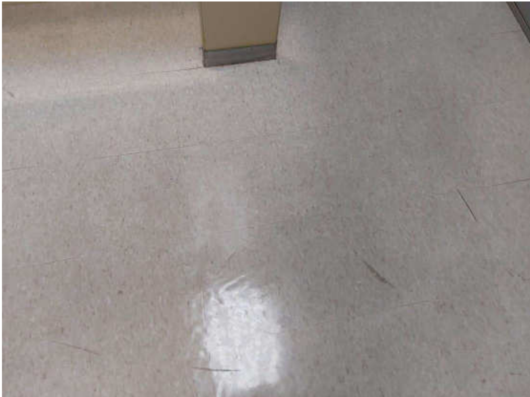
S0006C (None), 12" x 12" grey with light grey streaks, Floor, Vinyl Floor Tile and Mastic, Women's Washroom (Location #: 2)
