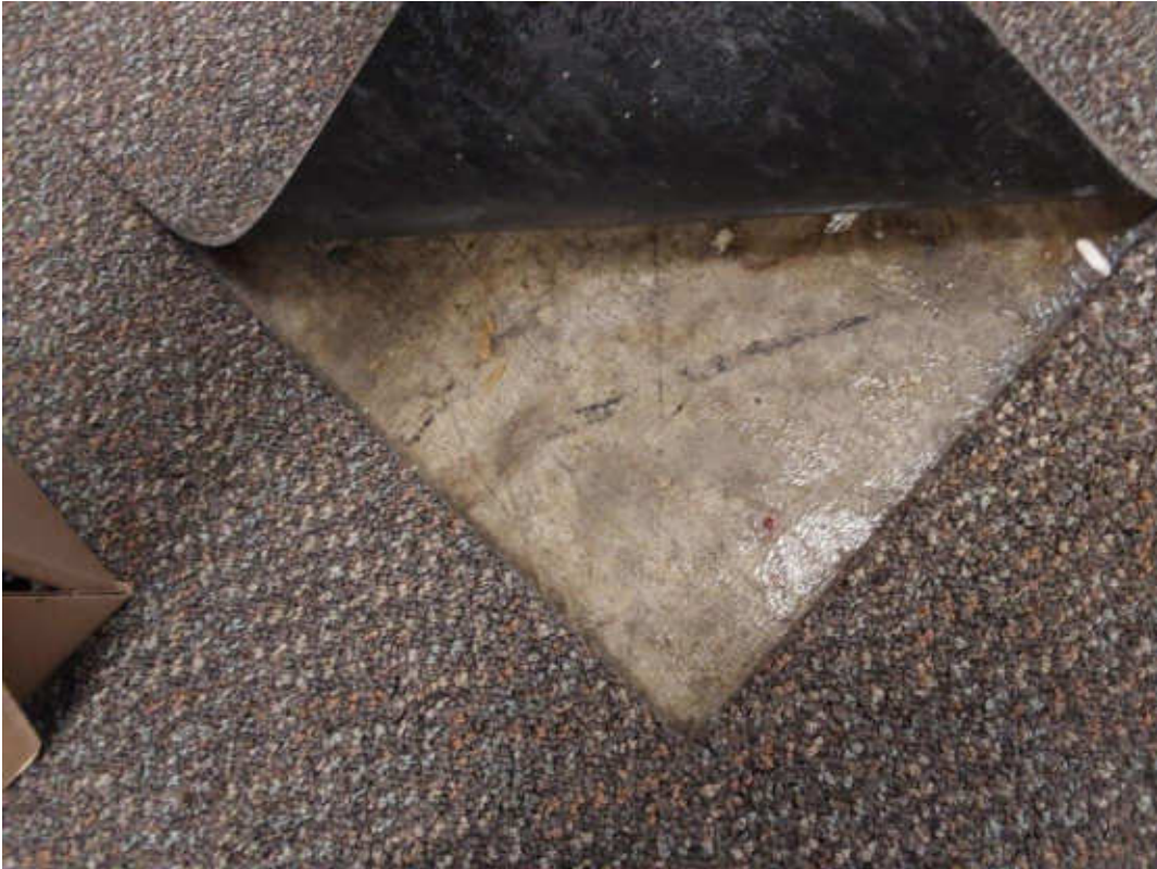
S0009C (None), Clear carpet mastic, Floor, Adhesive/mastic, Filing Room (Location #: 6)
