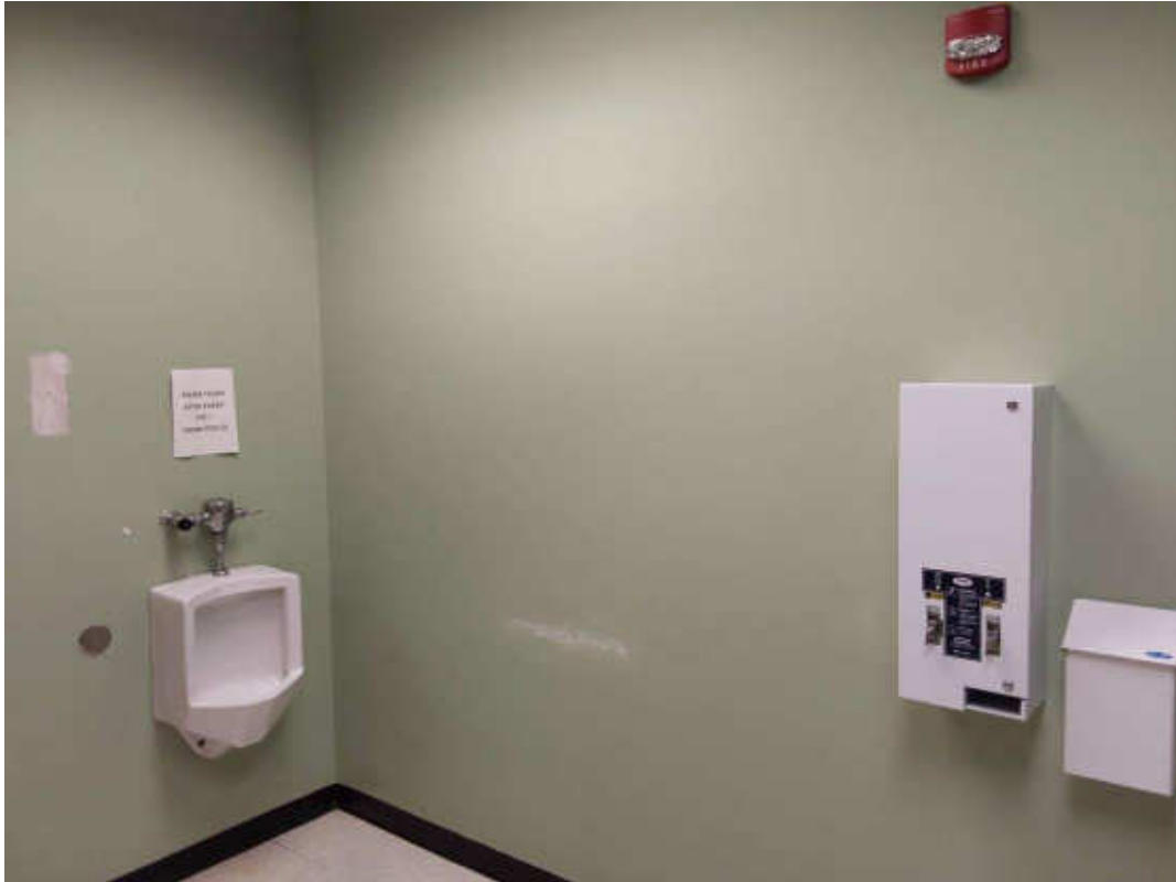
S0003B (None), Drywall on walls, Wall, Drywall and joint compound, Men's Washroom (Location #: 1)
