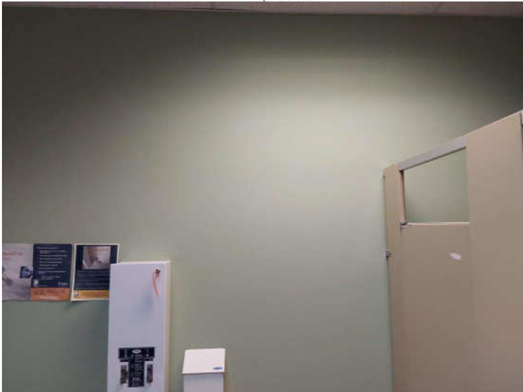
L0001(Lead, None), Light green paint on drywall, Wall, Women's Washroom (Location #: 2)
