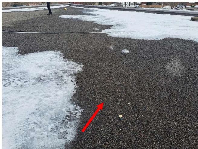
Photo 10: A view of the non-asbestos containing built-up roofing system (see arrow) observed throughout the Roof of the Subject building.
