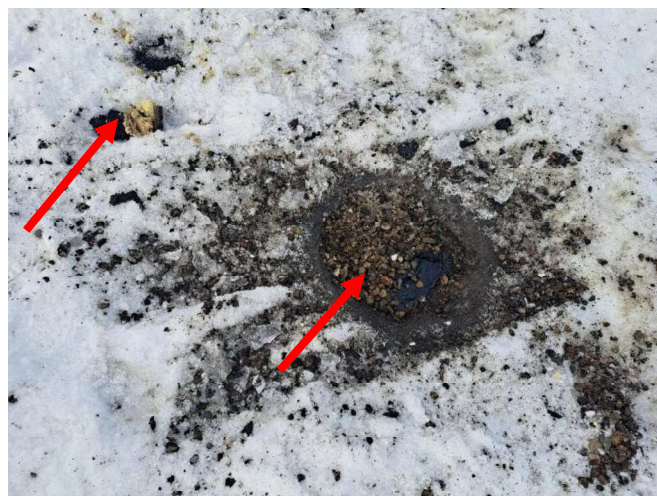
Photo 9: View of a typical roof core sample (see left arrow) and roof core sample location following repair (see right arrow) on the Roof of the Subject Building.
