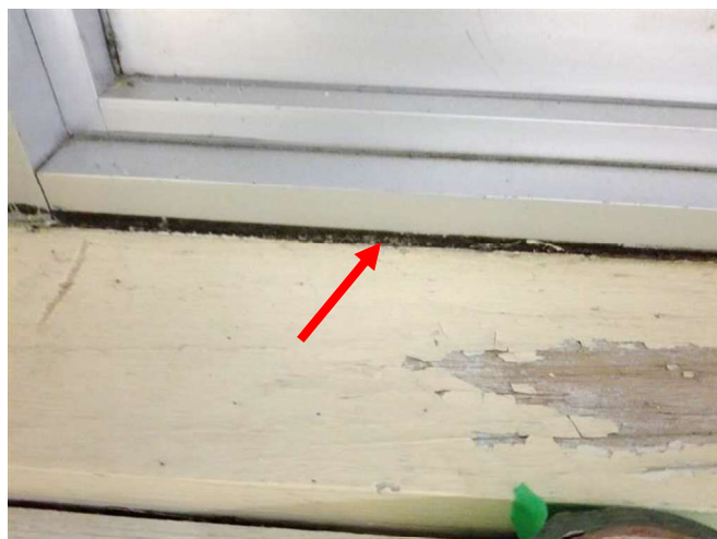
Photo 1: View of the asbestos containing white/grey caulking (see arrow) observed to be in good condition within Classroom 8 of the 1962 section of the Subject Building.
