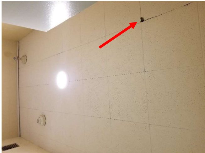
Photo 1: View of asbestos containing 1'x1' white acoustic ceiling tiles with small pinholes observed to be in fair condition (see arrow) observed within Room 111.
