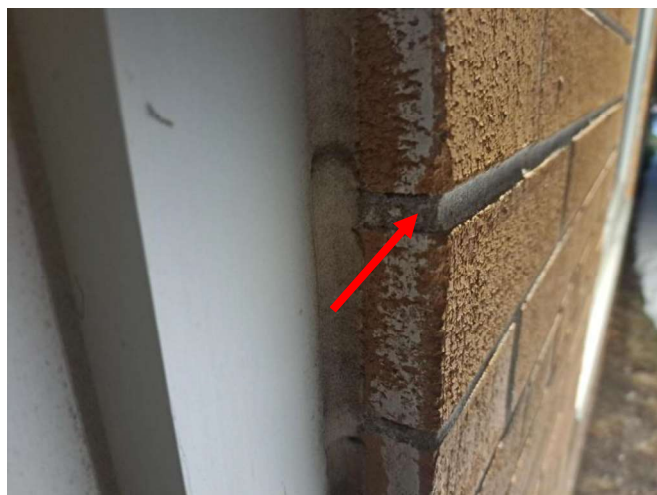
Photo 13: View of the non-asbestos containing white exterior caulking (see arrow) observed on the windows of the Subject Building.
