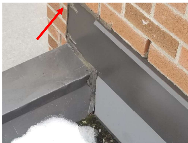
Photo 12: View of the non-asbestos containing black caulking (see arrow) adjacent to the flashing observed on the 1967 section of the Roof of the Subject Building.
