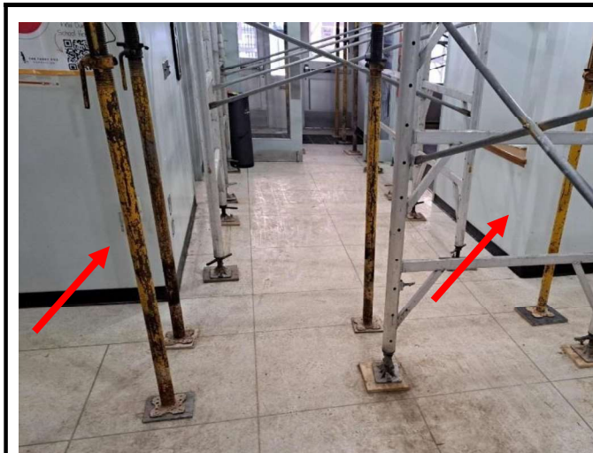
Photo 5: View of the asbestos containing plaster (see arrows) observed to be in good condition throughout the 1967 section of the Subject Building
