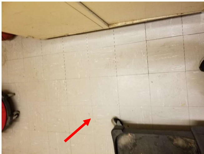
Photo 3: View of asbestos containing 9"x9" grey with light and dark streaks vinyl floor tiles (see arrow) observed to be in good condition within Room 113 of the Subject Building.
