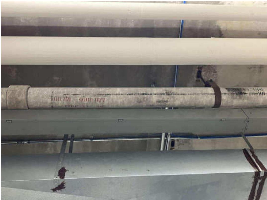
V9000 (Confirmed Asbestos), Piping, Cement Product, Hydraulics Lab (Location #: 261)
