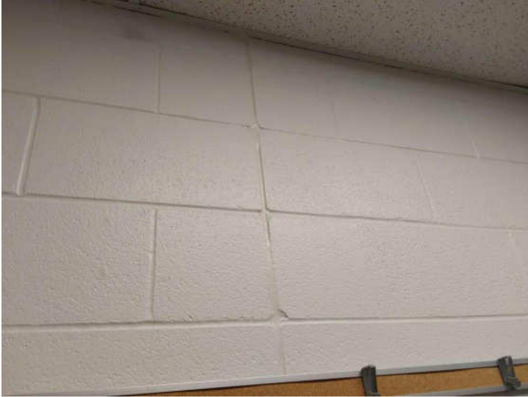
S0045C (None), Beige expansion joint caulking, Wall, Expansion Joint, Caulking, Classroom (Location #: 259)
