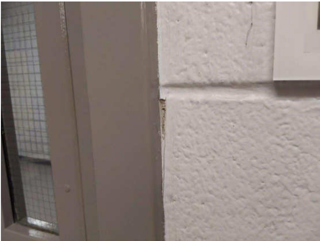
PCB, P0006(No), CAULKING, Caulking on door frames, Electrical Lab (Location #: 347)
