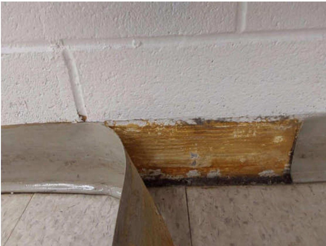
S0046C (None), Yellow baseboard mastic, Wall, Base, Adhesive/mastic, Classroom (Location #: 259)
