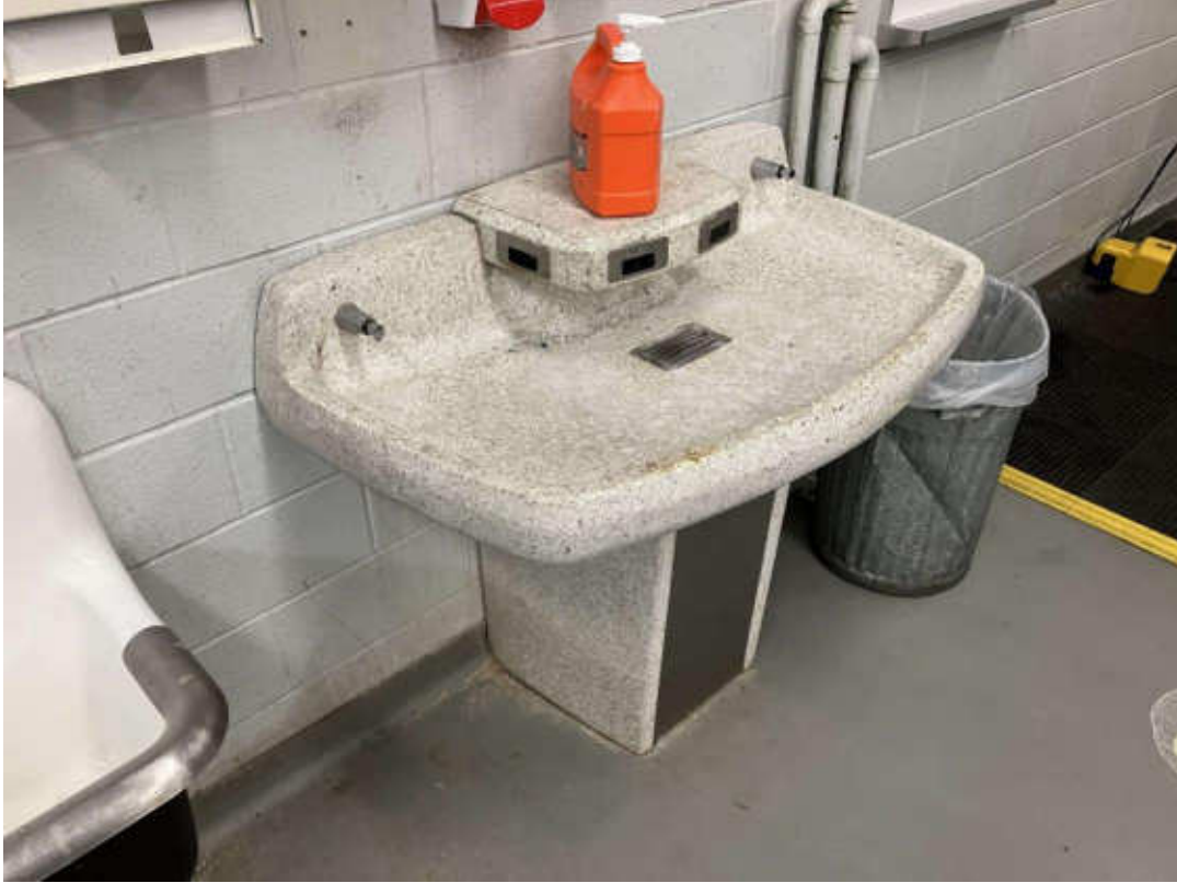
V9500 (Presumed Asbestos), Other, Sink, Terrazzo, Hydraulics Lab (Location #: 261) Bradley sink
