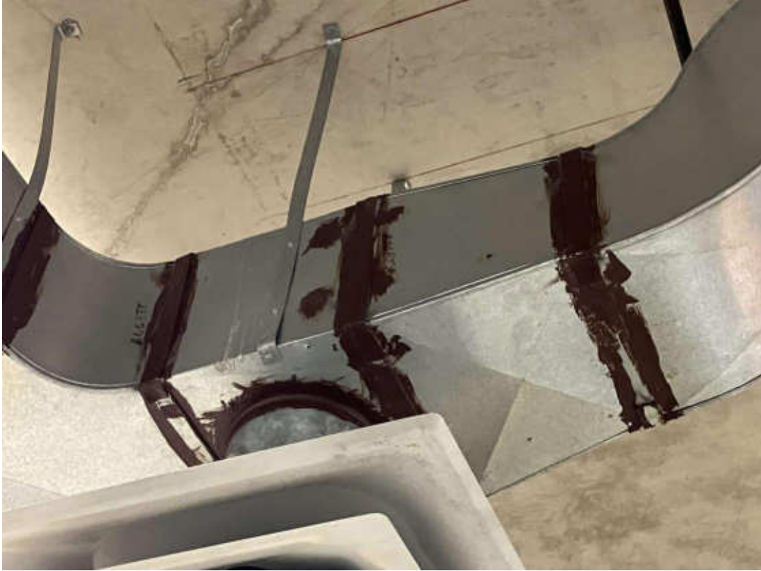
S0053C (None), Brown duct mastic, Duct, Mastic, Hydraulics Lab (Location #: 261)
