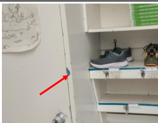
Photo 1: View of lead containing blue paint (layer 2) (see arrow) observed behind the non-lead containing beige paint on the closet and storage cupboard within Classroom 101 of the Subject Building.
