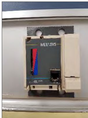
Photo 13 – Non-mercury thermostat present in assessed room.
