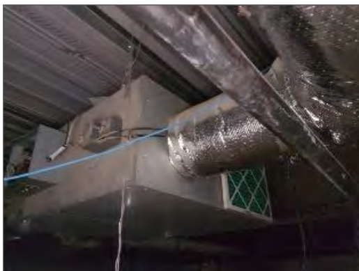
Photo 3 – Fiberglass insulated flex duct above lay-in ceiling tiles in room 104.
