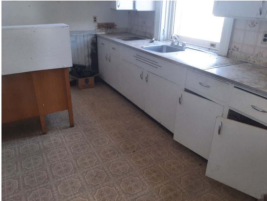
Photo 1 – Asbestos-containing beige square pattern vinyl sheet flooring.
