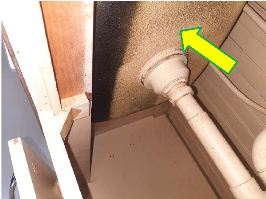
Photo 2 – Asbestos-containing sink coating.
