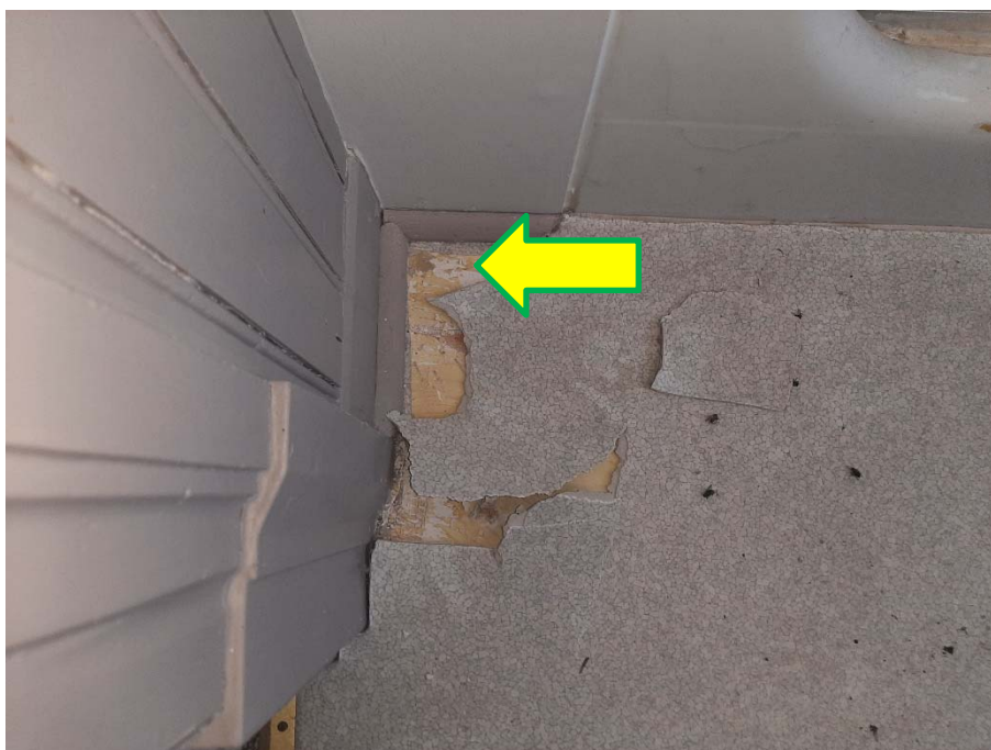
Photo 4 – Asbestos-containing white vinyl sheet flooring concealed beneath non-asbestos grey vinyl sheet flooring.
