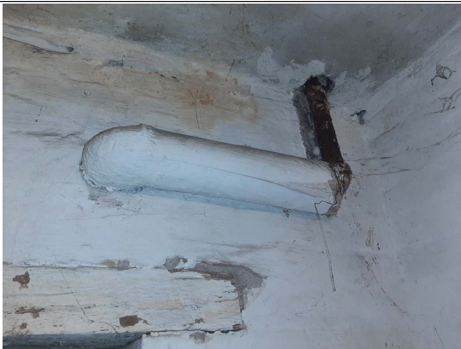
Photo 3 – Asbestos-containing parging cement and Aircell pipe insulation.
