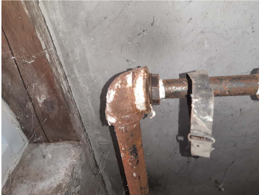
Photo 5 – Asbestos-containing residual parging cement pipe insulation.
