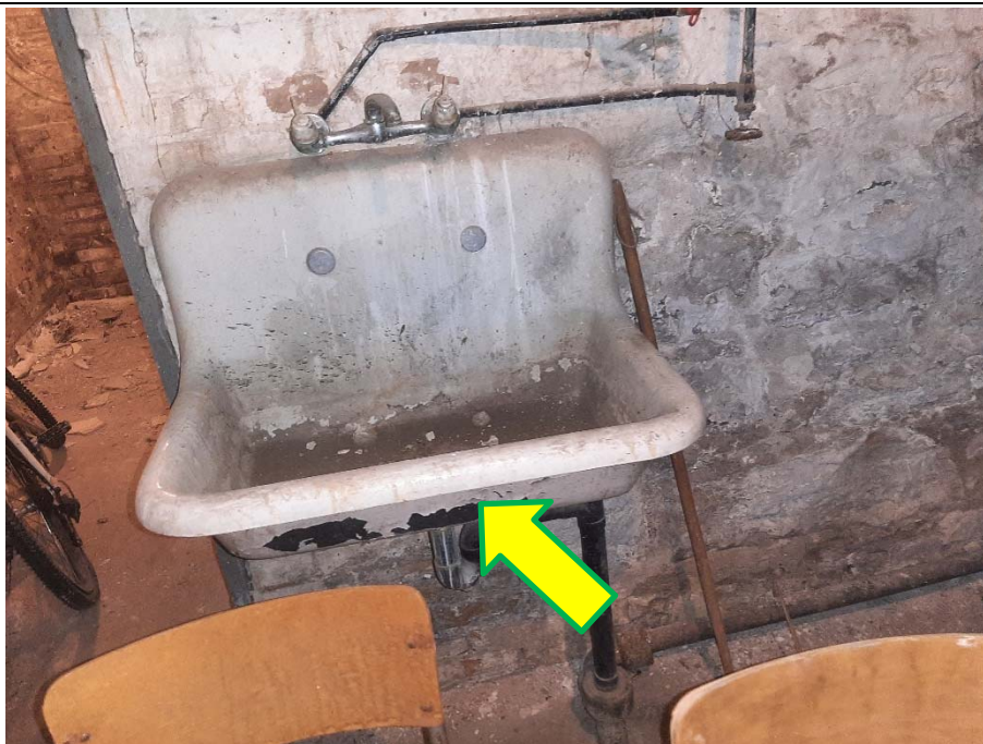
Photo 7 – Asbestos-containing sink coating in the basement.
