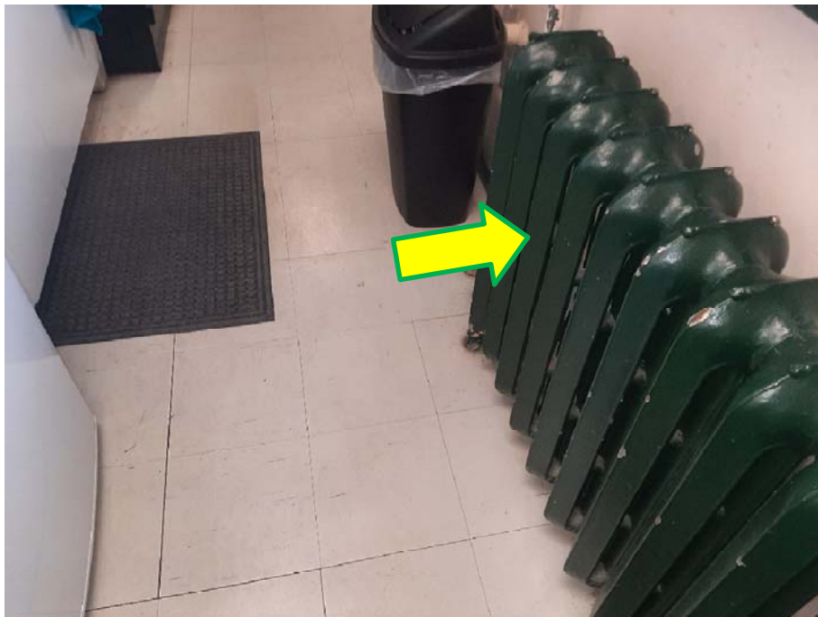
Photo 6 – Lead-based green paint.
