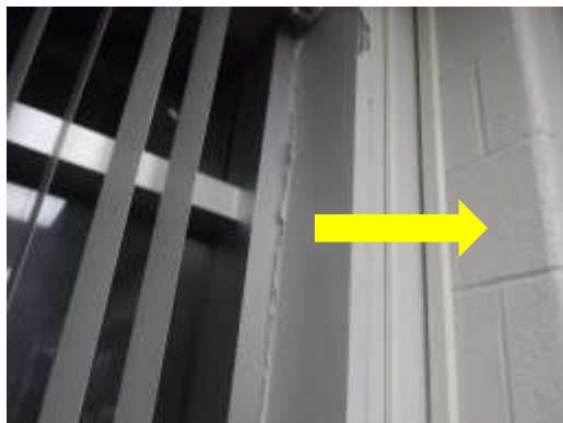
Asbestos-containing paint on the masonry walls is present in the 1963 phase of construction.
