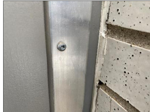
Non-asbestos white caulking on 1970 phase exterior door frame
