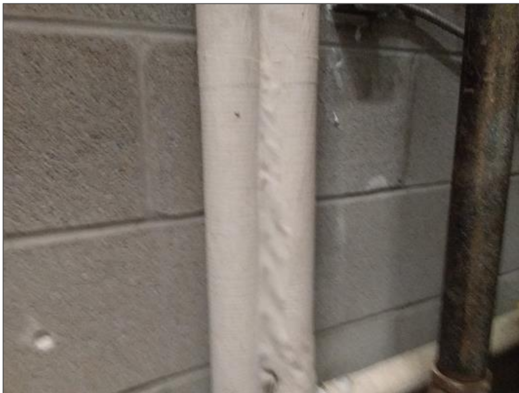
V0000 (None), Piping, All, Fibreglass, Meter Room (Loc. 3).
