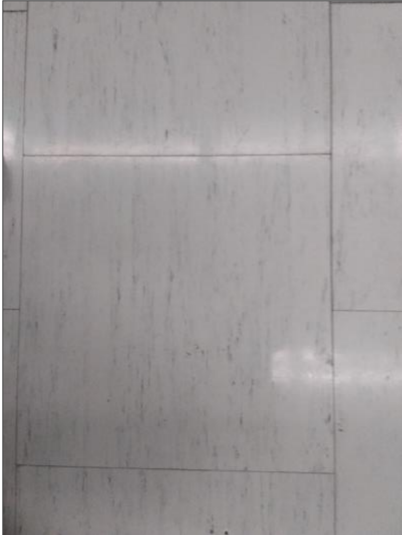
S0016 (Confirmed Asbestos), Floor, Vinyl Floor Tile and Mastic, Classroom # 10 (Loc. 40).
