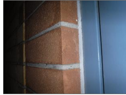
Photo 2 – Asbestos-containing grey caulk is present on the north Exit B doors.
