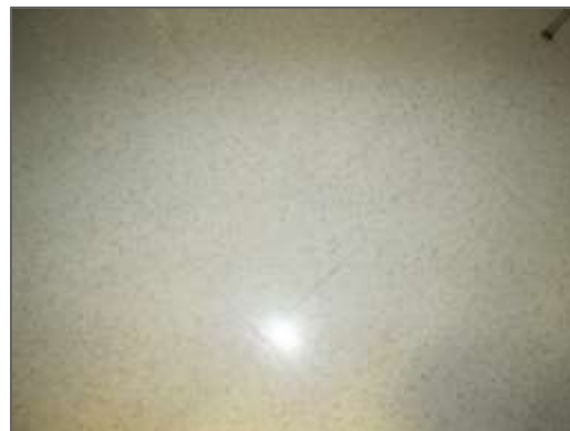
Non-asbestos 12" x 12" off-white vinyl floor tile with grey spots located in the Kitchenette (Location 20).
