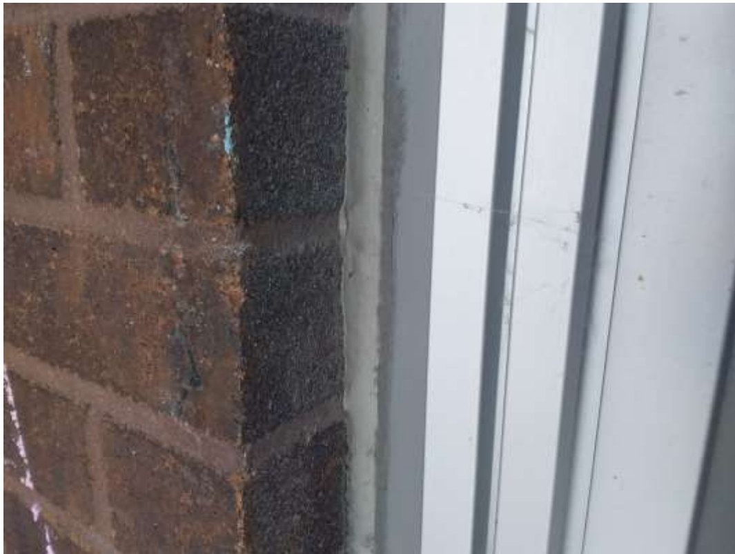
V9500 (Presumed Asbestos), Other, Caulking, Vestibule (Loc. 2)
