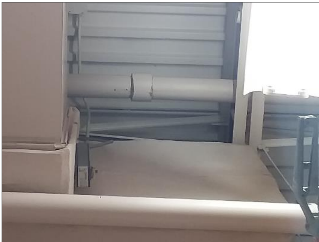
V9000 (Confirmed Asbestos), Piping, Cement Product, MEC1 (Loc. 52).
