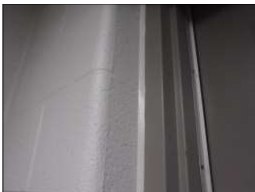
Non-asbestos white caulking on interior door frames of the 2001 phase of construction.
