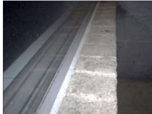
Non-asbestos light grey caulking on exterior window and door frames of the 1990 phase of construction.
