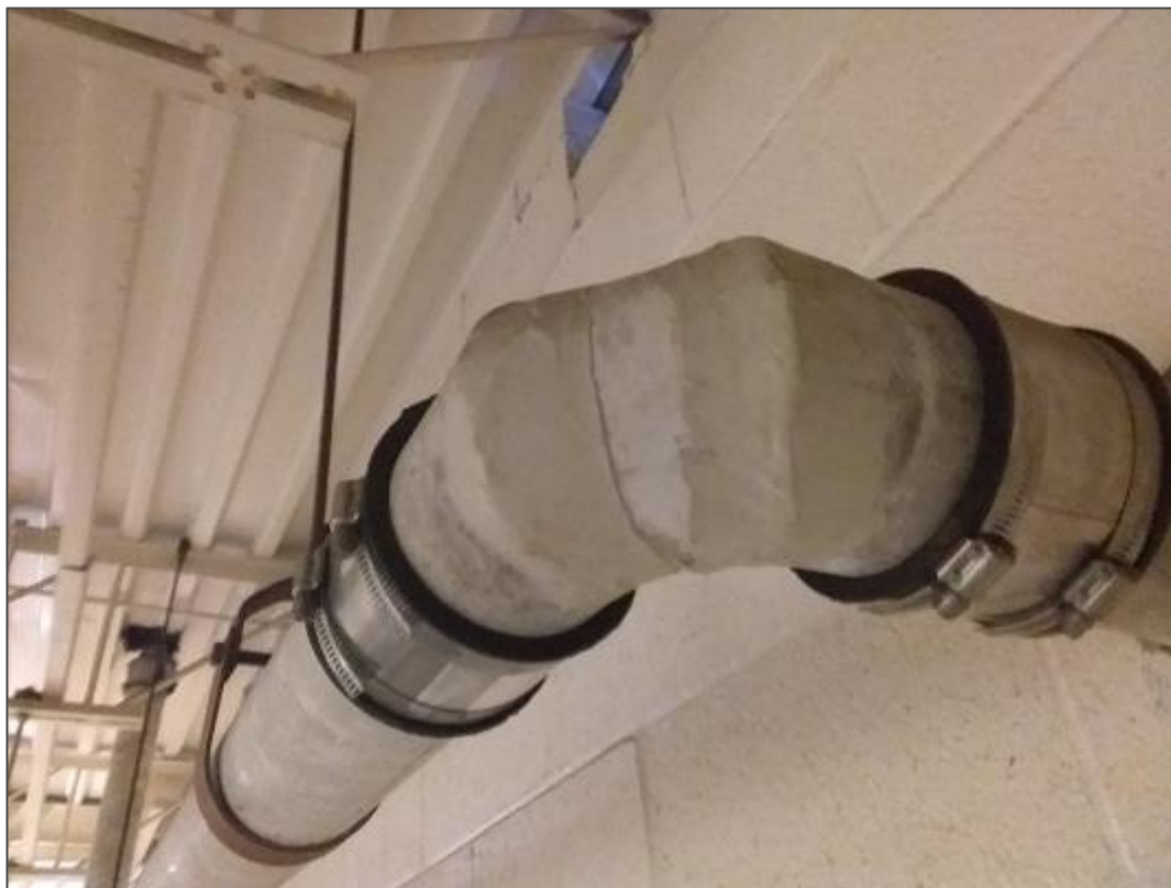
V9000 (Confirmed Asbestos), Other, Adhesive/mastic, BR01 (Loc. 53).
