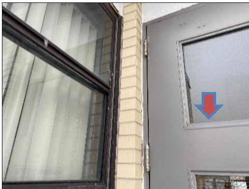
Non-asbestos putty on 1970 phase door frame
