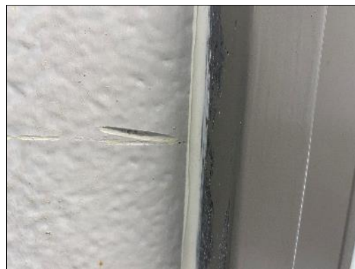
Presumed asbestos-containing white caulking on 1960 phase interior door frame
