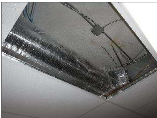
Non-asbestos fibre glass insulation on ventilation ducts present in assessed area.
