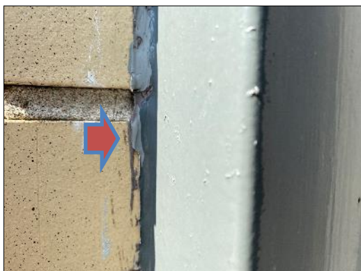
Asbestos-containing brown caulking present on exterior door frames
