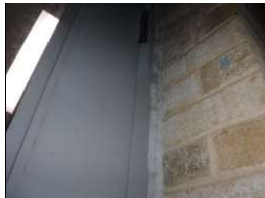
Non-asbestos dark grey caulking on exterior door frames of the 2001 phase of construction.
