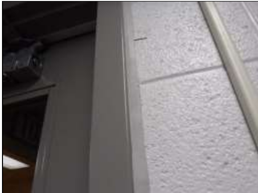
Non-asbestos light grey caulking on interior door frames of the 1990 phase of construction.
