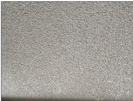
Texture finish, containing chrysotile asbestos, is present on the concrete soffit on the exterior (Location 25)
