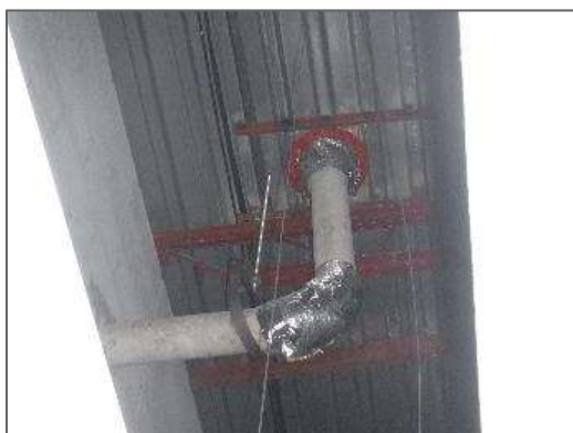
Transite pipe is present in the assessed area.
