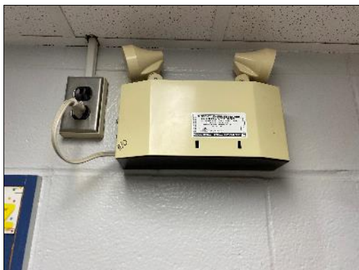
Lead-containing batteries are present in emergency lighting.
