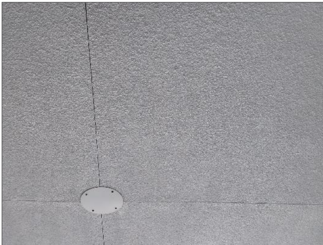
S0010 (Confirmed Asbestos), Other, Soffit, Texture Coat, Main Entrance Foyer & Exterior (Loc. 25).
