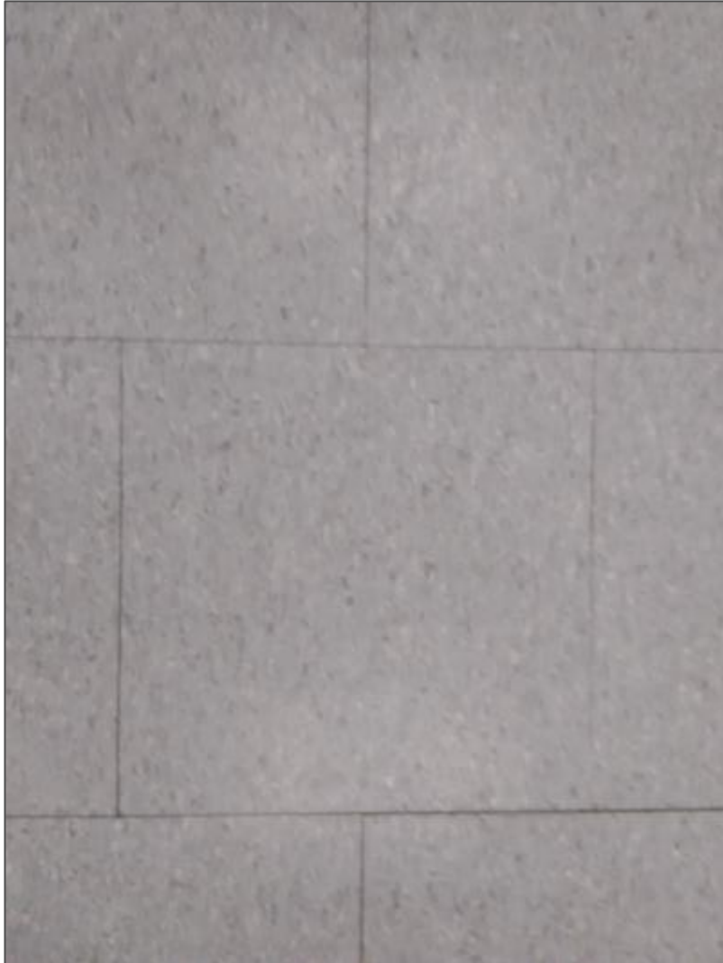
V9500 (Presumed Asbestos), Floor, Vinyl Floor Tile and Mastic, Classroom 9 (Loc. 4).
