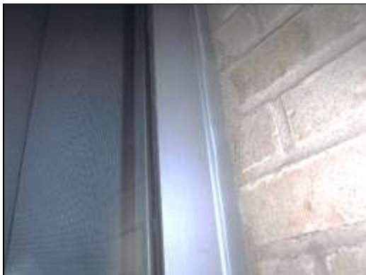
Non-asbestos light grey caulking on exterior window frames of the 2001 phase of construction.
