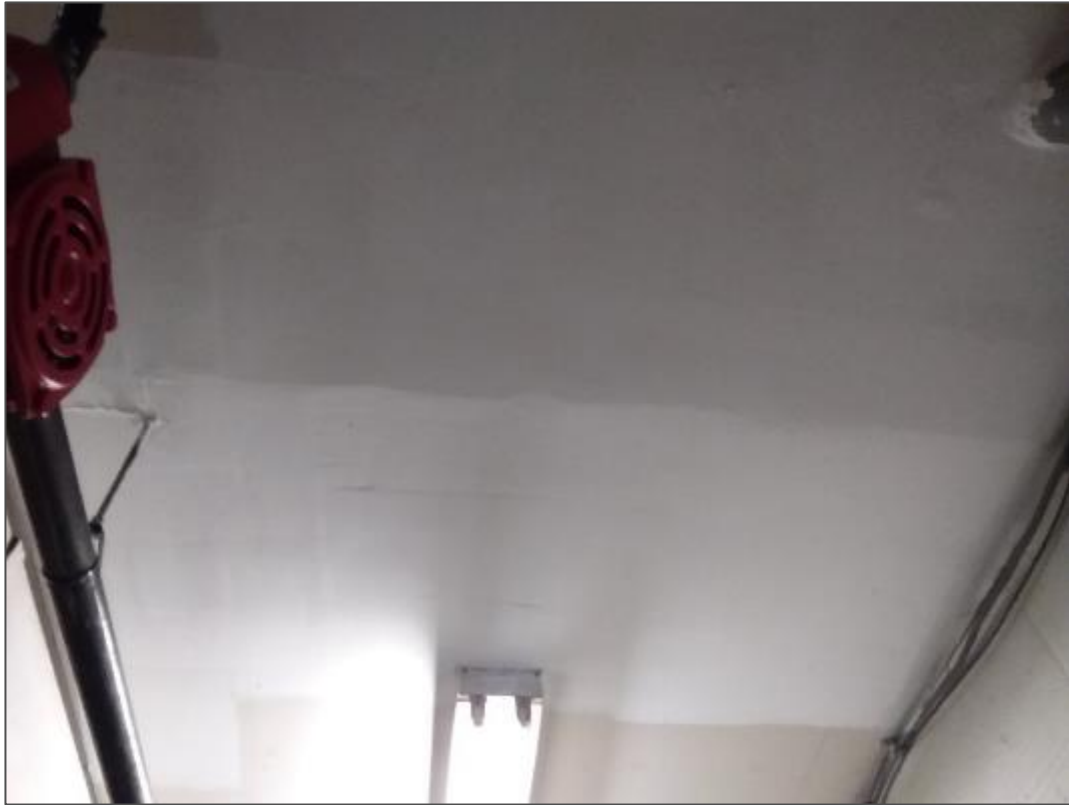
V9500 (Presumed Asbestos), Ceiling, Plaster, Boiler Room (Loc. 17).
