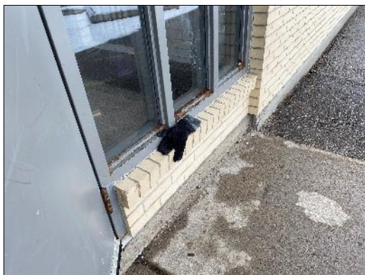
Non-asbestos grey caulking on exterior door frame
