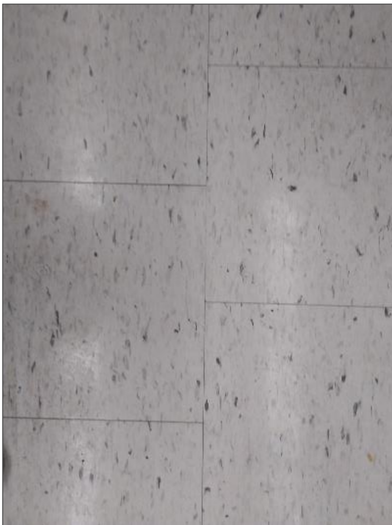
S0016 (Confirmed Asbestos), Floor, Vinyl Floor Tile and Mastic, Science Rm (Loc. 28).
