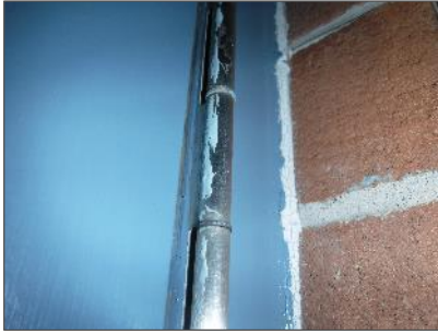
Photo 1 – Asbestos-containing white caulk is present on the west Exit 107 doors.
