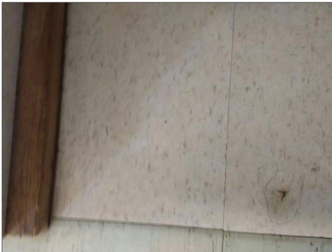
S0017 (Confirmed Asbestos), Floor, Vinyl Floor Tile and Mastic, Classroom # 10 (Loc. 40).
