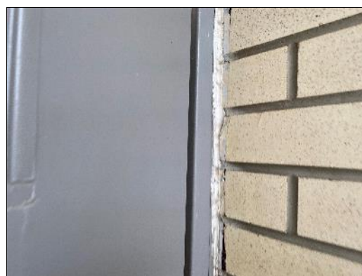
Non-asbestos white caulking on 1960 phase exterior door frame
