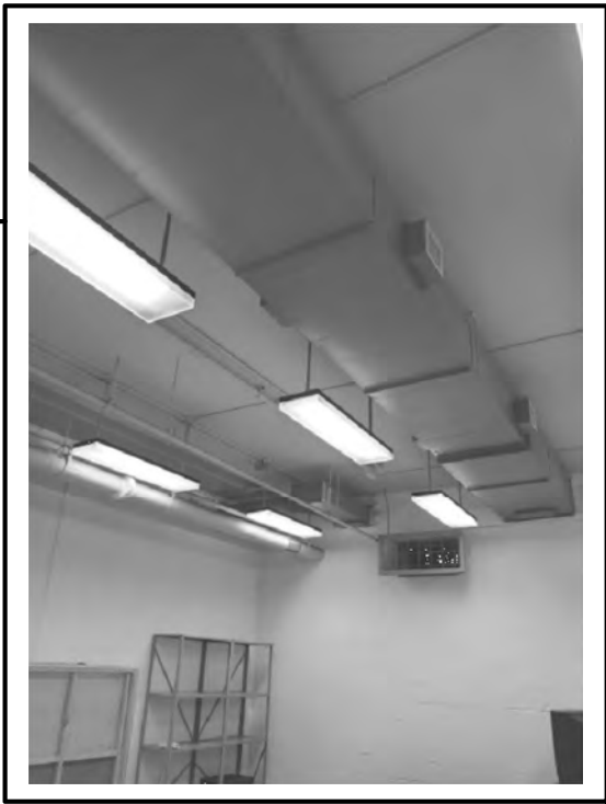
EXISTING ROOM EXHAUST AND SUPPLY DUCT
