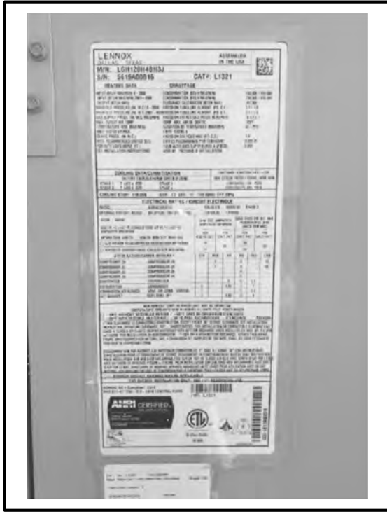
2.1 RTU NAMEPLATE UNIT BY : LENNOX
