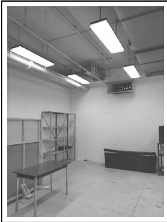
EXISTING SPACE SHOWING DUCTWORK TO BE DEMOLISHED
