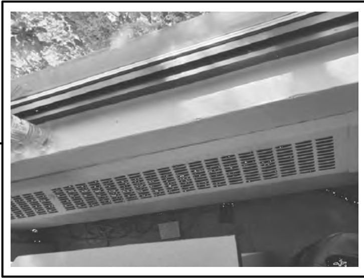
EXISTING HOT WATER PERIMETER HEATERS
