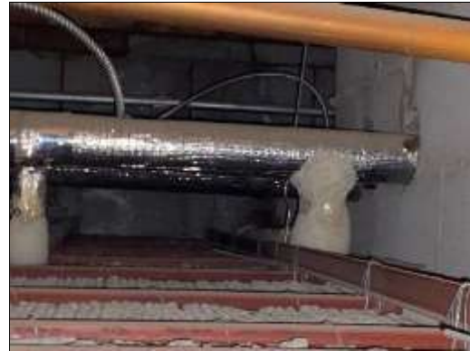
Presumed asbestos containing parging cement above ceiling.
