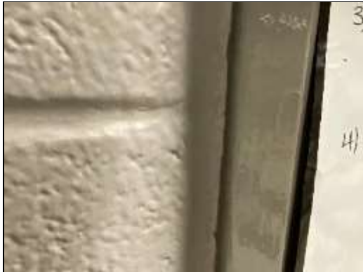
Asbestos containing brown caulking present on interior door frames.
