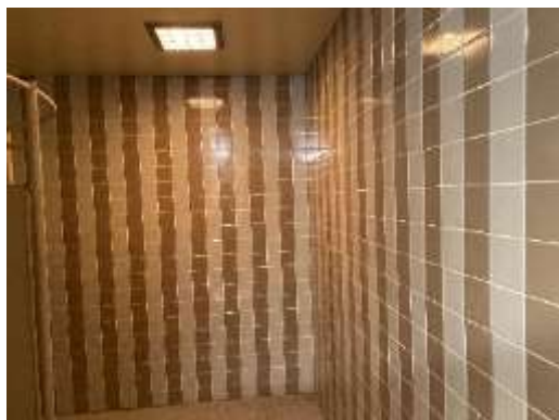
Non-asbestos thin set on walls within Girls Washroom/Change room/Shower (Location 8).
