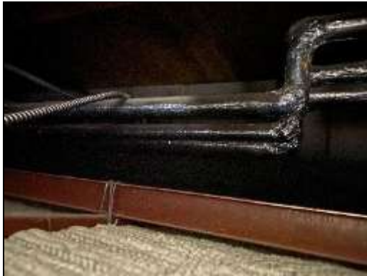
Pipes are insulated with non-asbestos fiberglass above ceiling.
