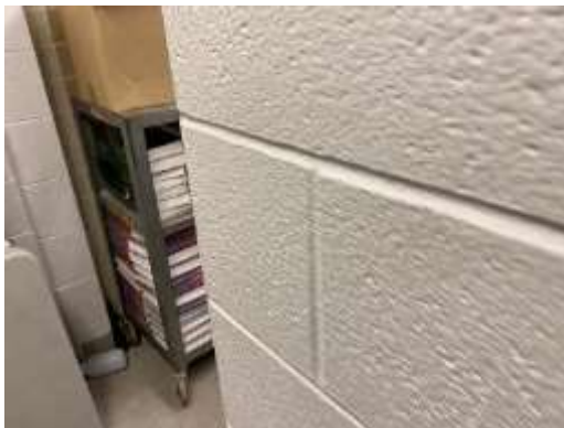
Non-asbestos white paint on concrete within Girls Washroom/Change room/Shower (Location 8).
