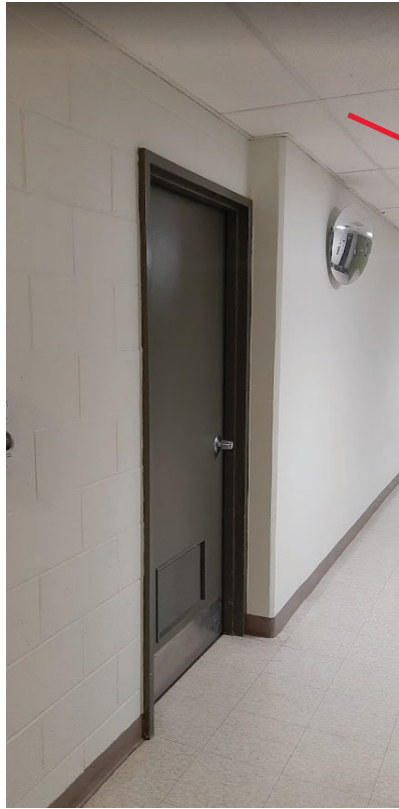
Photograph A - Image of Existing Door. See note 4 on 1/A201
