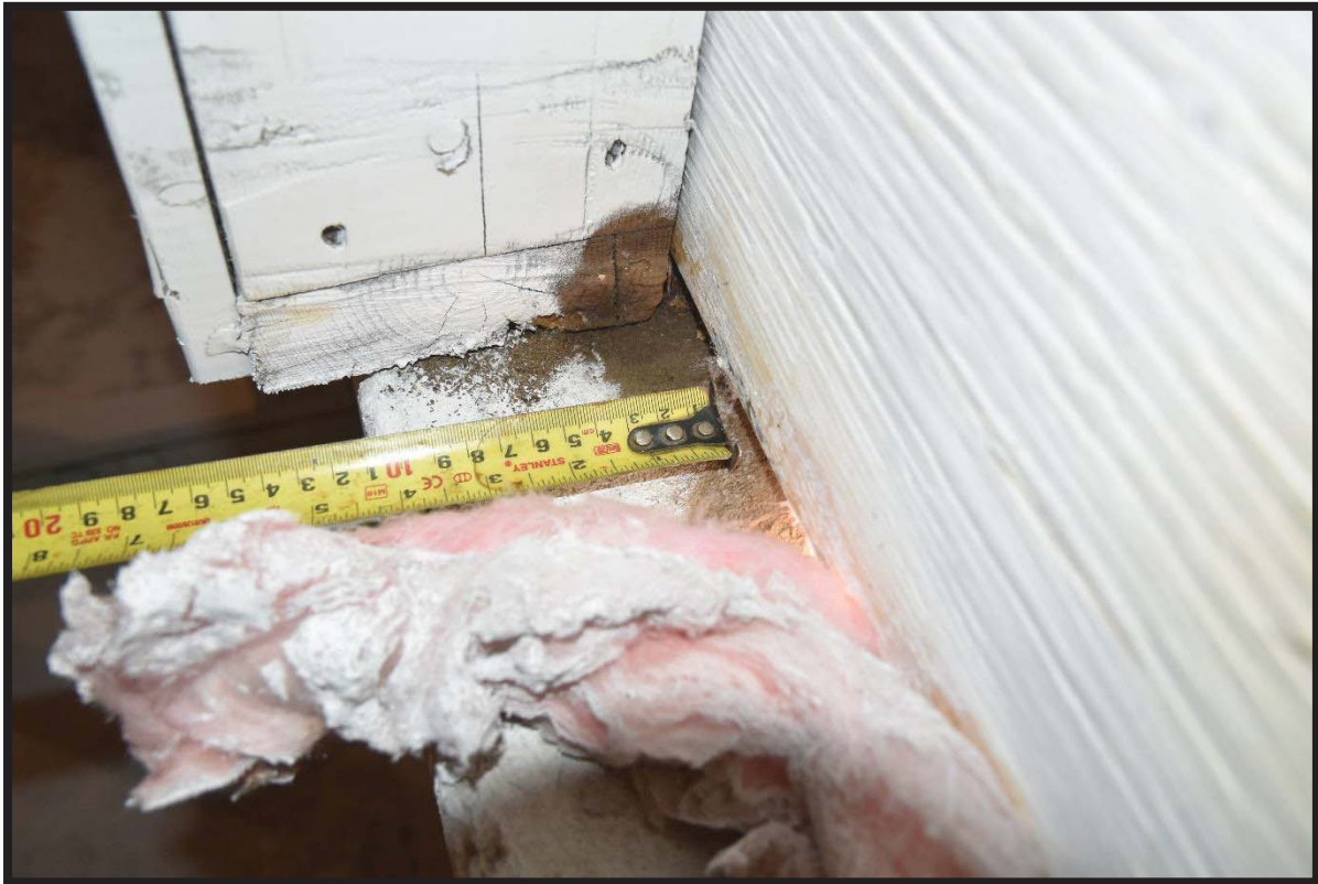
15. Wall frame offset from concrete block foundation wall.
