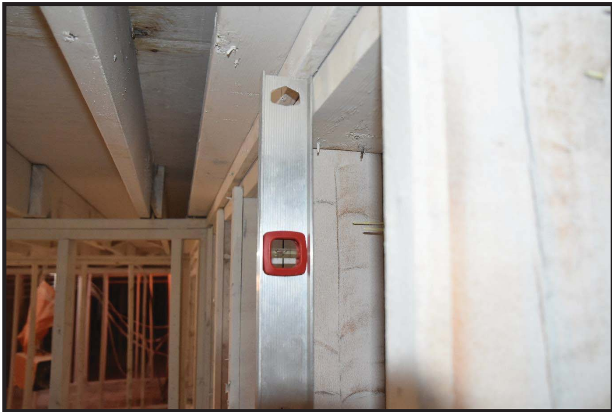
16. Exterior wall framing out of plumb.
