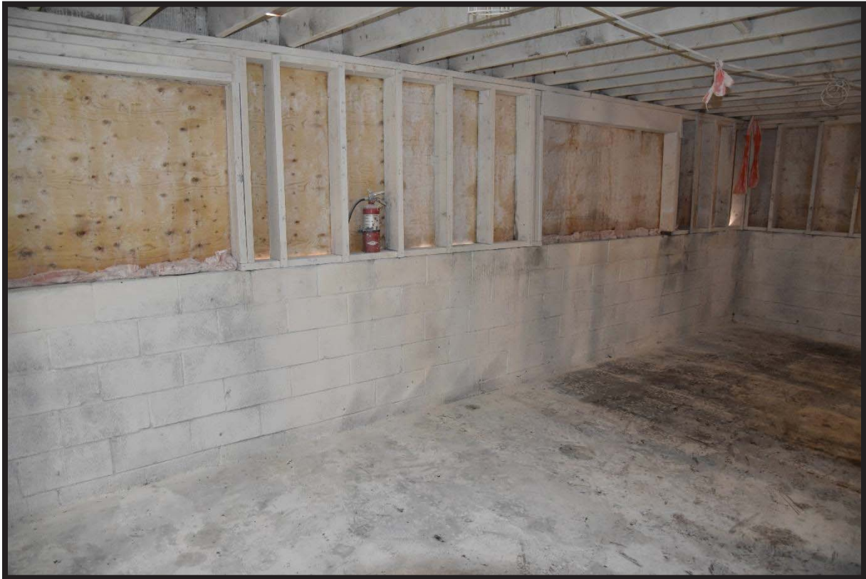
5. Structural elements remediated for smoke contamination and water damage.
