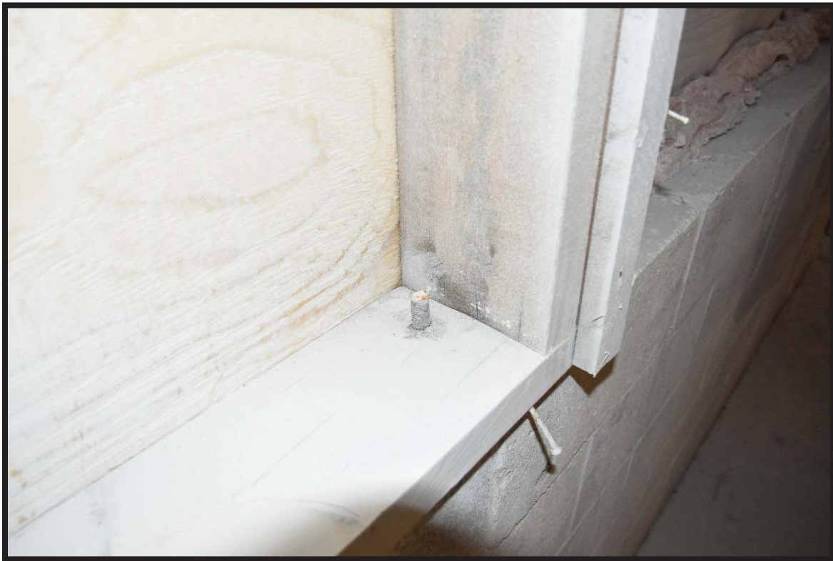
18. Unsecured anchor bolt (typical condition).
