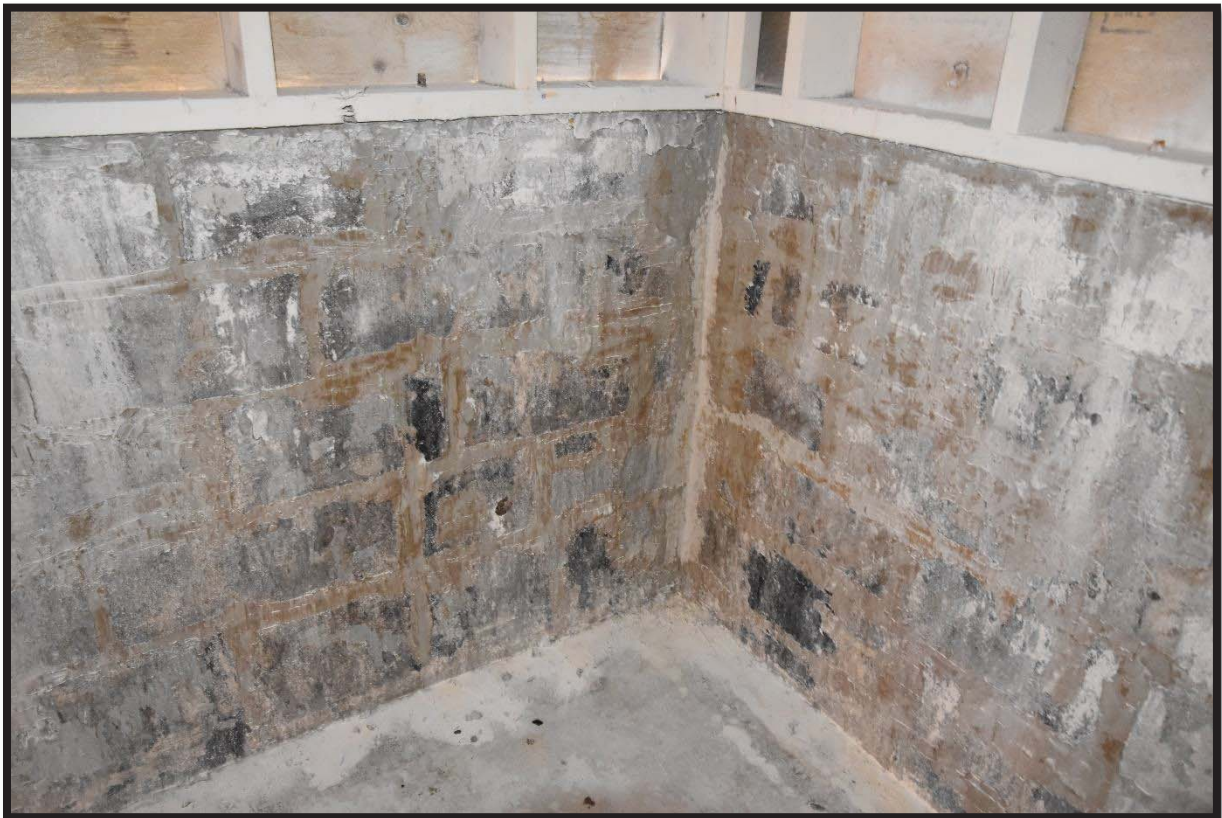
12. Aged moisture damage to foundation wall.
