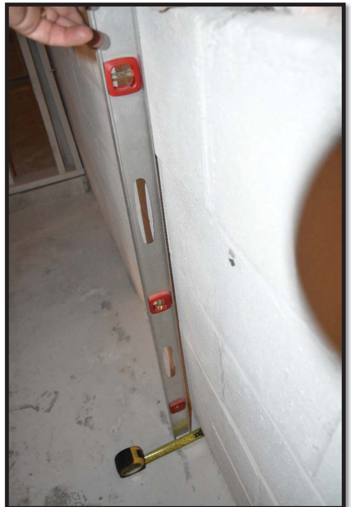
8. Foundation wall out of plumb.
