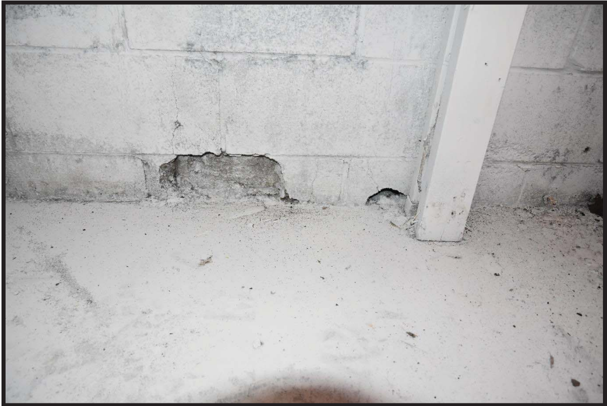
11. Cavity at base of foundation wall.
