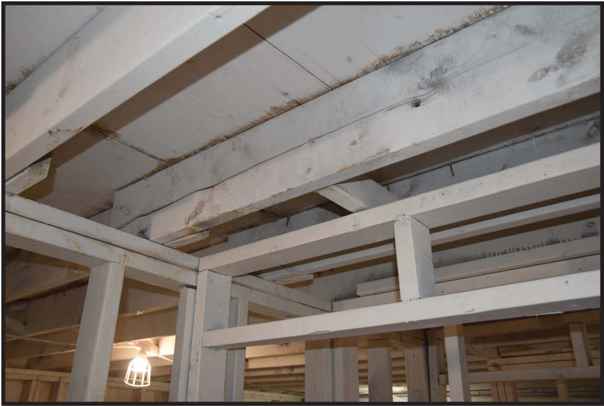
19. Cracked floor joist.
