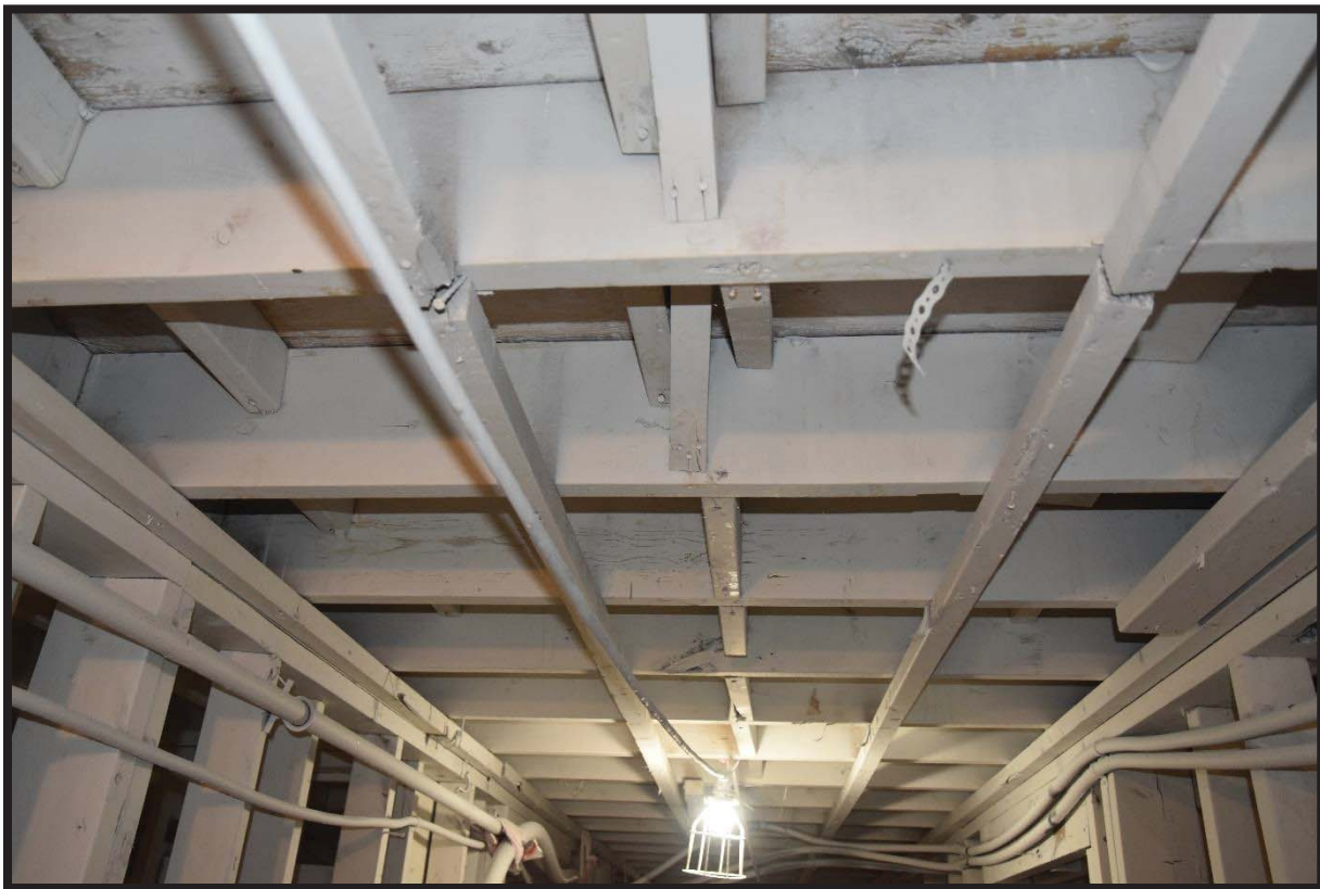
6. Remediated wood framing.
