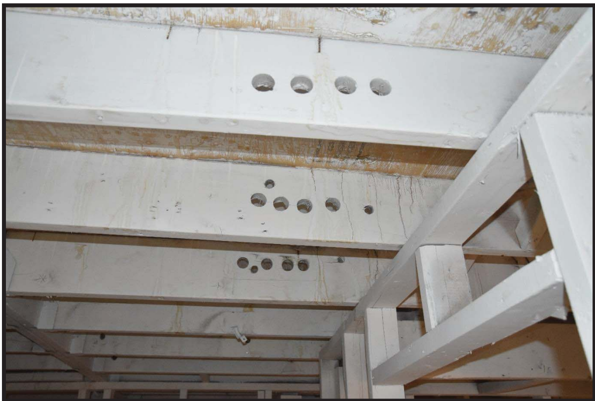
20. Holes in floor joists (for services).
