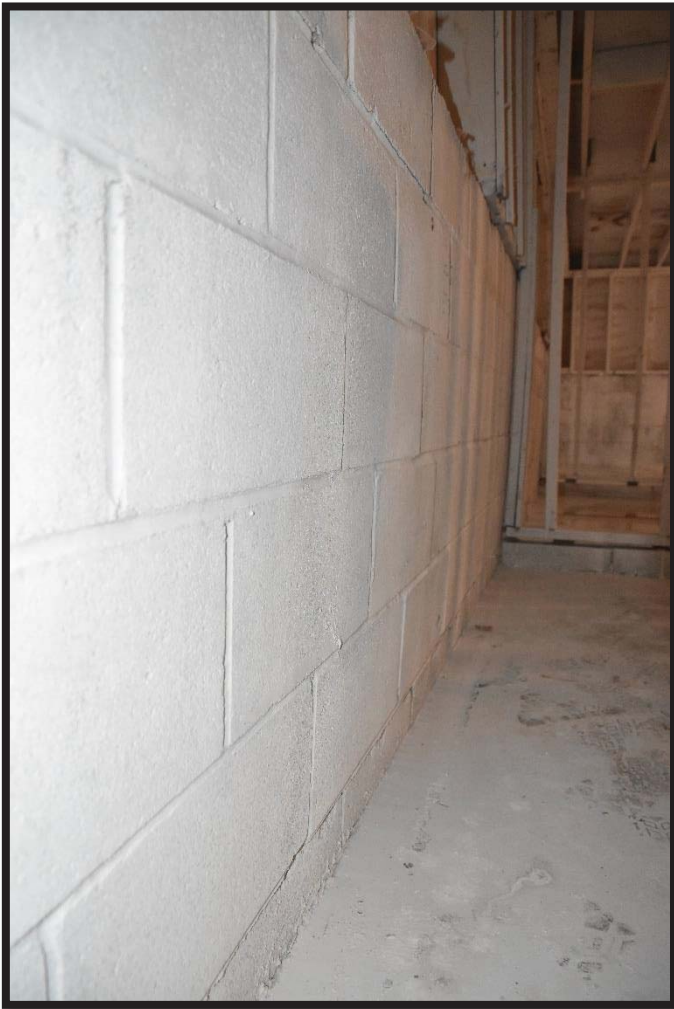
7. Foundation wall out of plumb.
