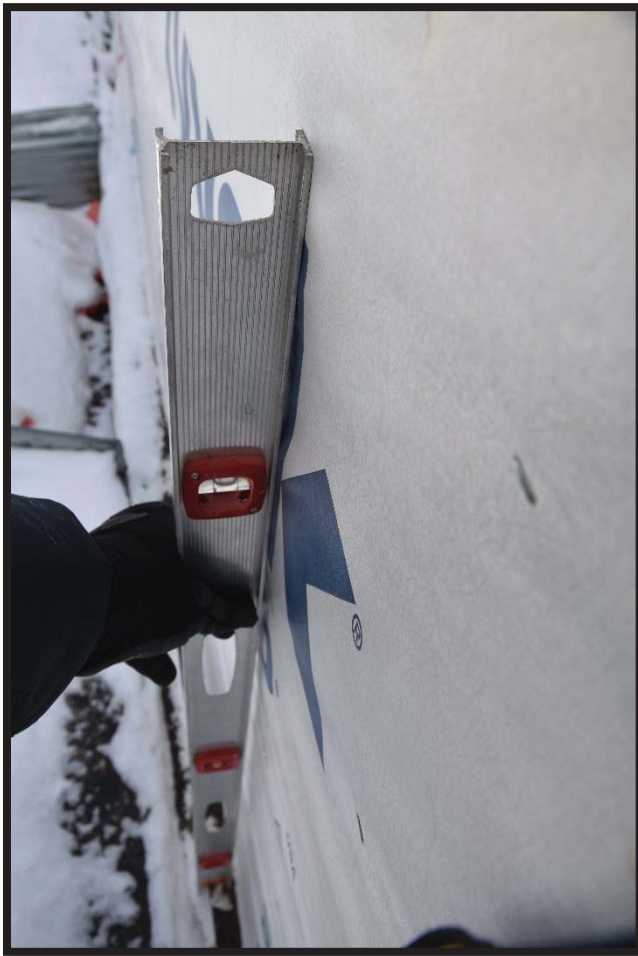
17. Top of exterior wall leaning out relative to bottom of wall.
