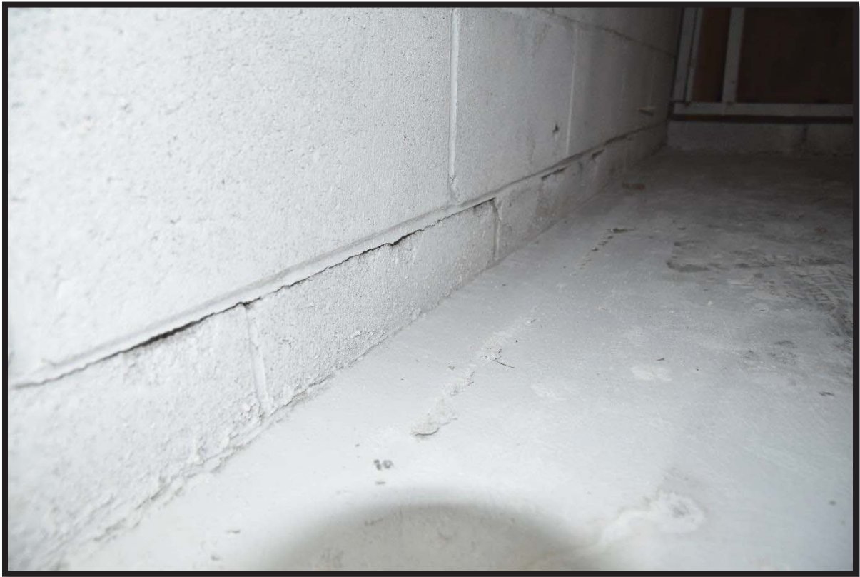
9. Horizontal crack in foundation wall.
