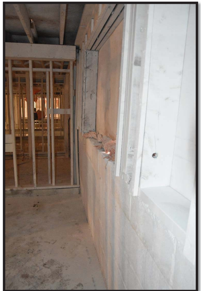
14. Exterior wall frame out of plumb.
