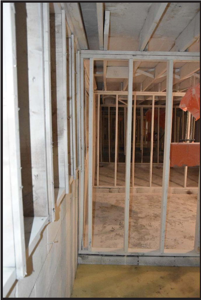
13. Misalignment in exterior wall framing.
