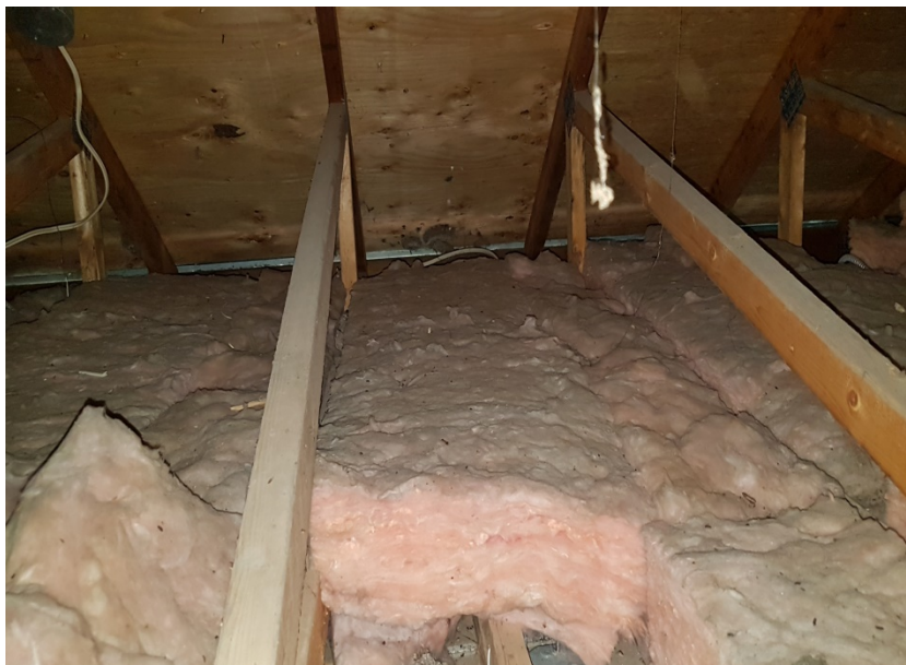
Photo 1 – Non-asbestos fibreglass insulation in the attic.
