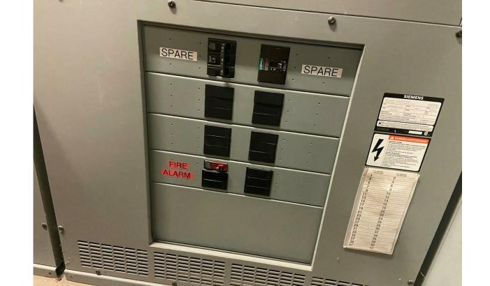
SPARE BREAKER IN EX. DISTRIBUTION BOARD DPA TO BE UTILIZED FOR 50A 3Ø SERVICE TO CU-01
