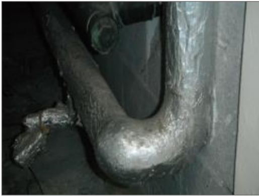
Photo 2 – Asbestos-containing parging cement on hot water heating pipe systems with foil jacketing.
