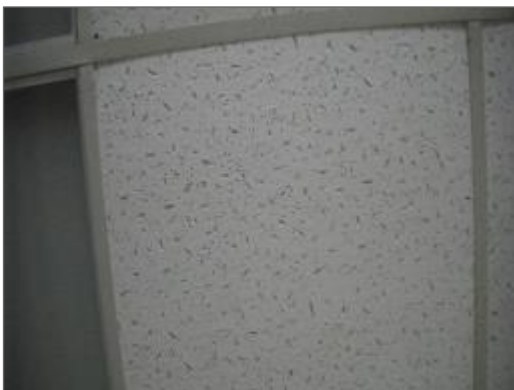
Photo 12 – Non-asbestos 24" x 48", lay-in, fissure, dimples and pinhole.
