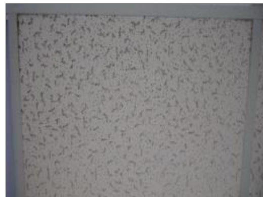
Photo 13 – Non-asbestos 24" x 48", lay-in, multi-directional ridges with large pinhole.
