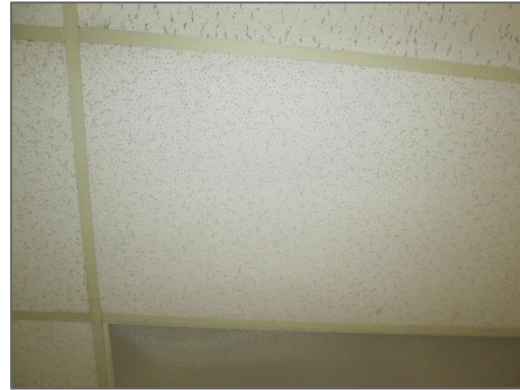
Photo 9 – Non-asbestos 24" x 48", lay-in, white depressed fissure with pinhole.
