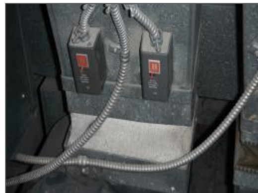
Photo 27 – Asbestos-containing vibration damper present in Upper Mechanical Room 2.
