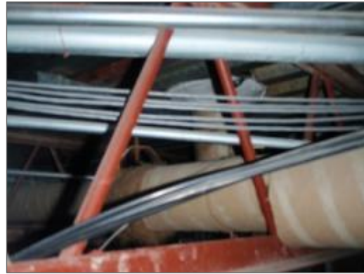
Photo 3 – Non-asbestos sweatwrap present on rain water leader pipe systems.
