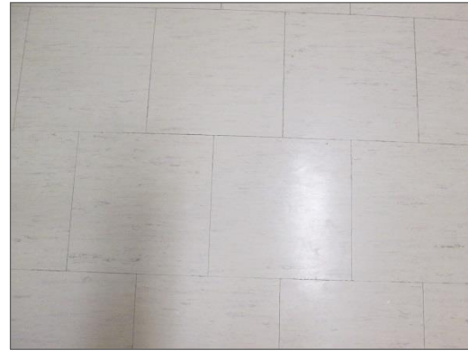
Photo 25 – Non-asbestos 12" x 12" vinyl floor tile white with blue streak with asbestos-containing mastic beneath.
