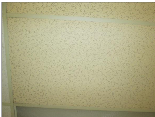
Photo 6 – Non-asbestos 24" x 48", lay-in, random fissure and medium pinhole.
