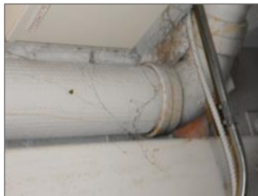
Photo 19 – Transite rain water leader; Storage Room (Location 44).
