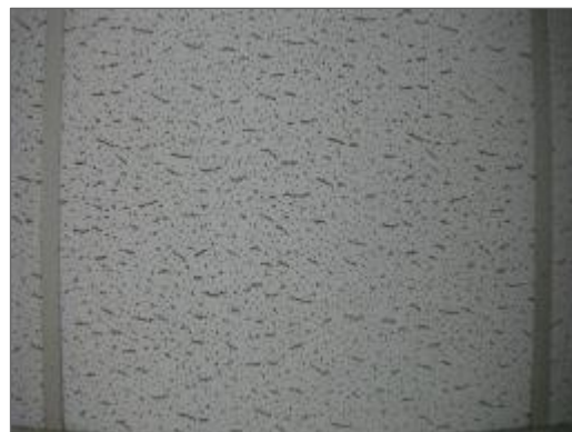
Photo 7 – Non-asbestos 24" x 48", width wise fissure and hole ceiling tile.
