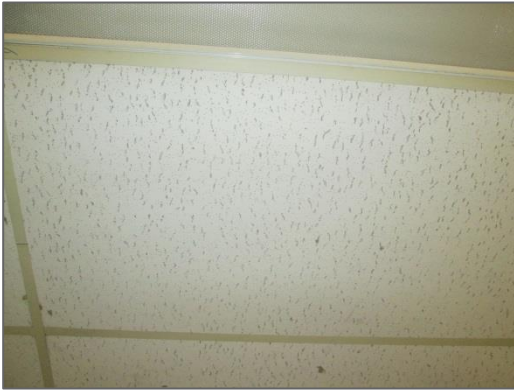
Photo 8 – Non-asbestos 24" x 48", multi directional ridges with pinhole.
