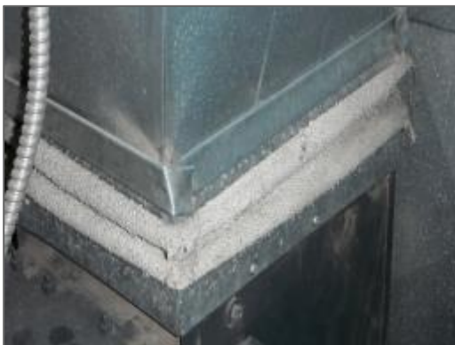
Photo 26 – Asbestos-containing duct vibration damper Upper Mechanical Room 2.
