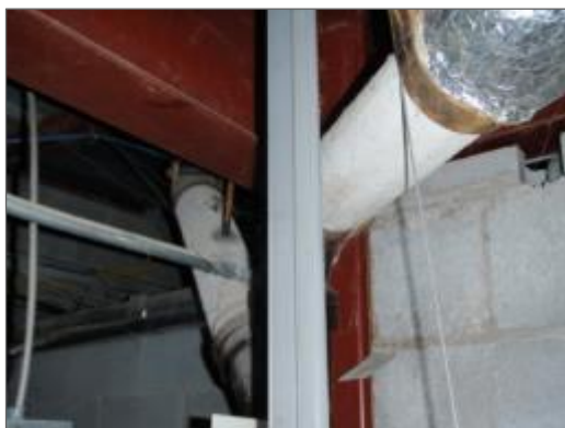
Photo 18 – Transite pipe present as a rain water leader above ceilings in the corridors.
