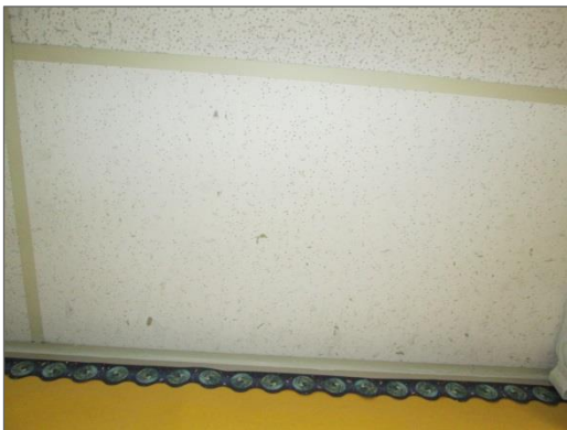
Photo 16 – Non-asbestos 24" x 48", lay-in, rough ridges and pinhole ceiling tile.
