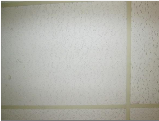
Photo 14 – Non-asbestos 24" x 48", lay-in acoustic ceiling tile present in the Corridors.
