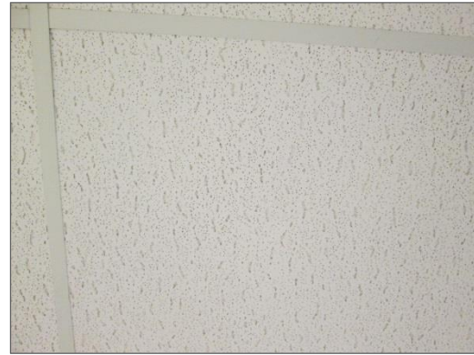
Photo 15 – Non-asbestos 24" x 48", lay in, ridges and pinhole ceiling tile.
