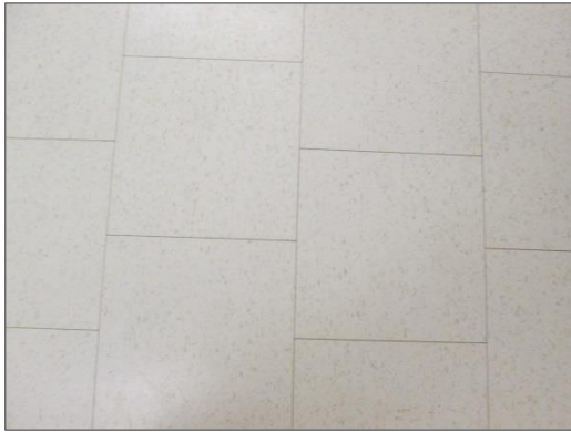
Photo 24 – Non-asbestos 12" x12" white with grey replacement tiles.
