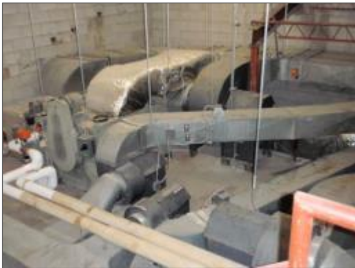
Photo 4 – Ducts in the upper Mechanical Room (Location 5) insulated with non-asbestos fibreglass.
