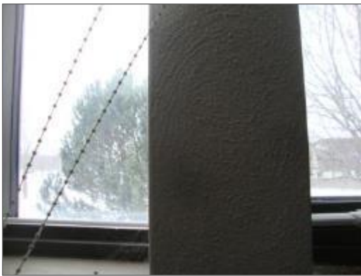
Photo 1 – Non-asbestos texture finish present on steel columns in Classroom 102 and 104.
