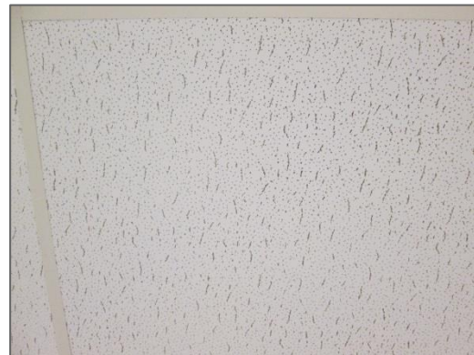
Photo 11 – Non-asbestos 24" x 48", ceiling tile fissure with tight pinhole bundle.
