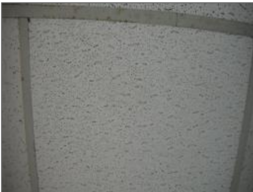
Photo 10 – Non-asbestos 24" x 48", lay-in, large width-wise fissure and large pinhole ceiling tile.
