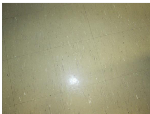
Photo 21 – Asbestos-containing 12" x 12" beige with brown and white streak floor tile.
