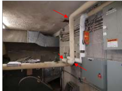
Asbestos-containing parging Fan Room 124 (Location 49).
