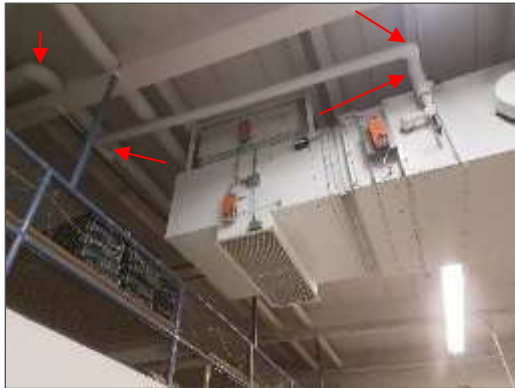
Asbestos-containing parging around AHU in Electrical Shop B107 (Location 92).
