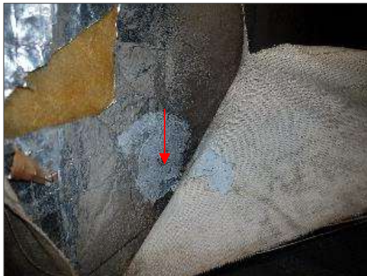
Asbestos-containing parging cement on pins of fibreglass ducts in Fan Room 124 (Location 49).
