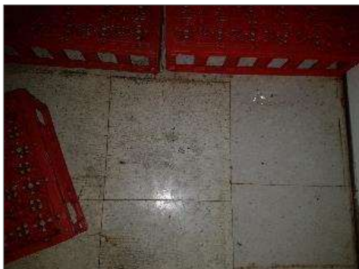
Non-asbestos 12" x 12" beige with brown splotch vinyl floor tiles (left) and 12" x 12" white with beige splotch vinyl floor tiles (right).
