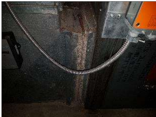
Presumed asbestos textile vibration dampers on AHU in Fan Room 124A (Location 50).
