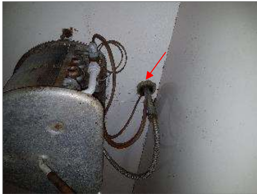
Asbestos-containing grey caulking in walk-in cooler at wall penetration.
