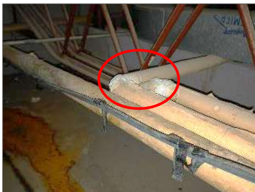
Asbestos-containing parging cement above walk-in cooler.
