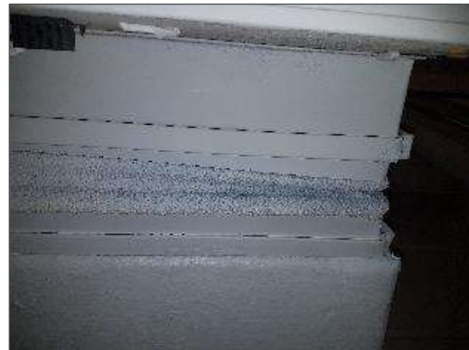
Presumed asbestos textile vibration dampers on AHU in Electrical Shop B107 (Location 92).
