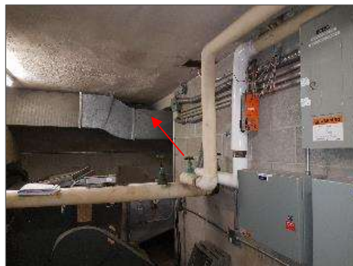
Asbestos-containing plaster ceilings in Fan Room 124 (Location 49).
