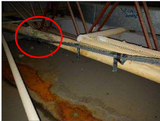
Visible water damage and mould observed on fiberglass pipe insulation above walk-in cooler.
