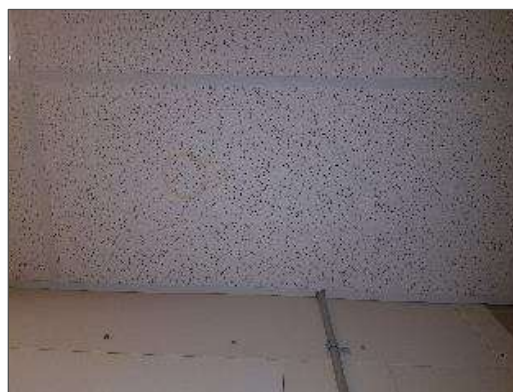
Non-asbestos 24" x 48", lay-in width wise fissure and pinhole ceiling tile in Kitchen 126 (Location 34).
