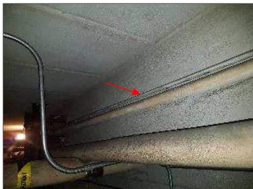
Non-asbestos plaster bulkheads in Mech Room (Location 84).
