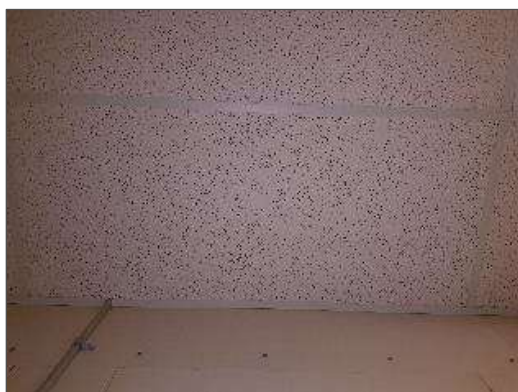
Non-asbestos 24" x 48", lay-in, fleck and pinhole ceiling tile in Kitchen 126 (Location 34).
