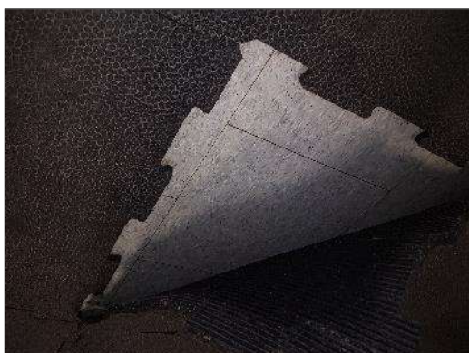
Non-asbestos grey and white splotch replacement tiles.
