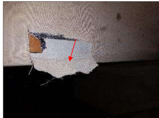
Asbestos-containing glued-on paper of fibreglass duct in Fan Room 124 (Location 49).
