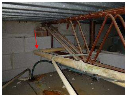
Asbestos-containing parging cement above walk-in cooler.
