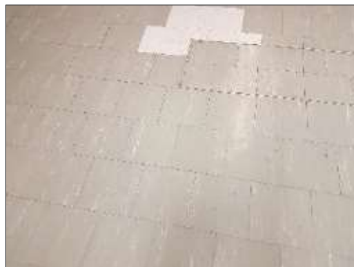
Asbestos-containing 9" x 9" grey with white streak vinyl floor tiles.
