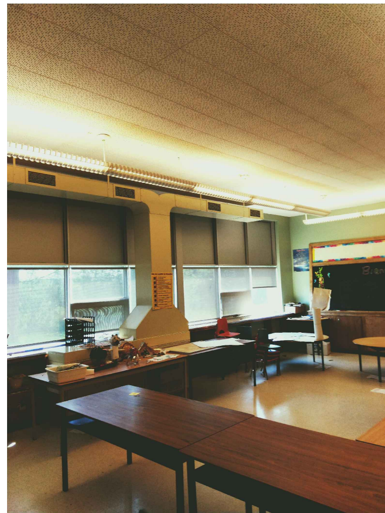
EXISTING UNIT VENTILATOR IN CLASSROOM
