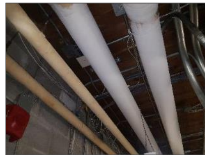
Photo 2 – Non-asbestos fibreglass pipe insulation in Electrical Room 124B.
