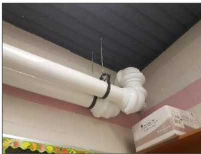
Photo 1 – View of non-asbestos fibreglass pipe insulation in classrooms.
