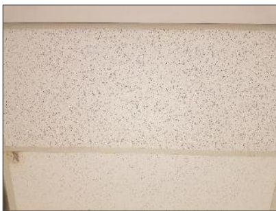
Photo 8 – Non-asbestos 24" x 48", lay-in ceiling tile with pinholes and random flecks.
