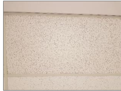
Photo 7 – Non-asbestos 24" x 48", lay-in ceiling tile with dense pinholes with fissure widthways.
