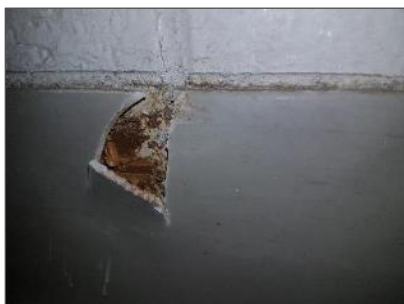
Photo 13 – Non-asbestos vinyl baseboard adhesive.
