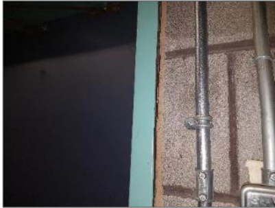
Photo 14 – Asbestos containing beige caulking around doorframe in Room 124B.
