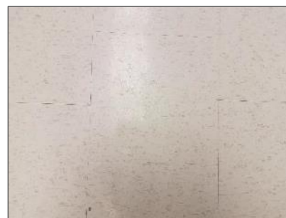
Photo 12 – Non-asbestos 12" x 12" white vinyl floor tile with grey streak.
