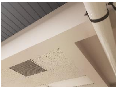
Photo 9 – Drywall bulkheads are located in Classrooms 124, 126, 137 and 133.
