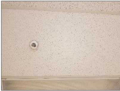
Photo 6 – Non-asbestos 24" x 48", lay-in ceiling tile with medium and large pinholes.
