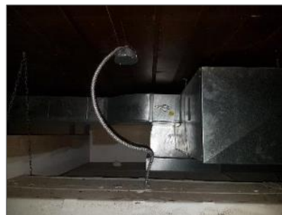
Photo 5 – Ducts above ceiling tile are uninsulated.
