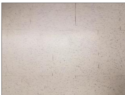
Photo 11 – Non-asbestos 12" x 12" white vinyl floor tile with blue fleck.
