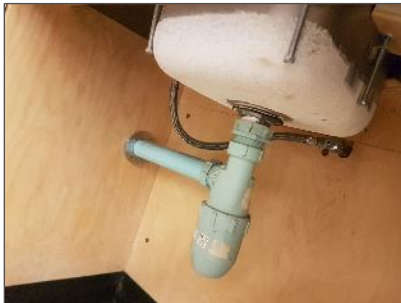
Photo 15 – Non-asbestos white sink mastic in room 124.
