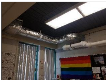
Photo 4 – View of foil-faced, non-asbestos fiberglass duct insulation.
